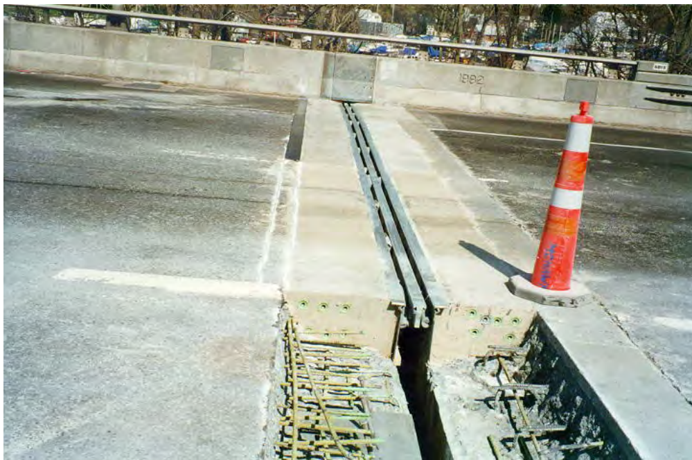
Figure 5.6-13 Modular Type Expansion Joint Replacement.
