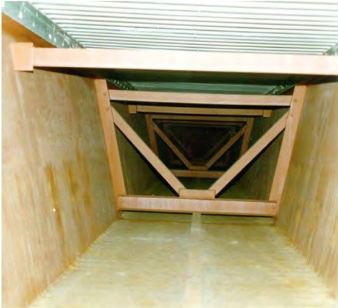
Figure 5.7-33 Inside Steel Box Girder.
