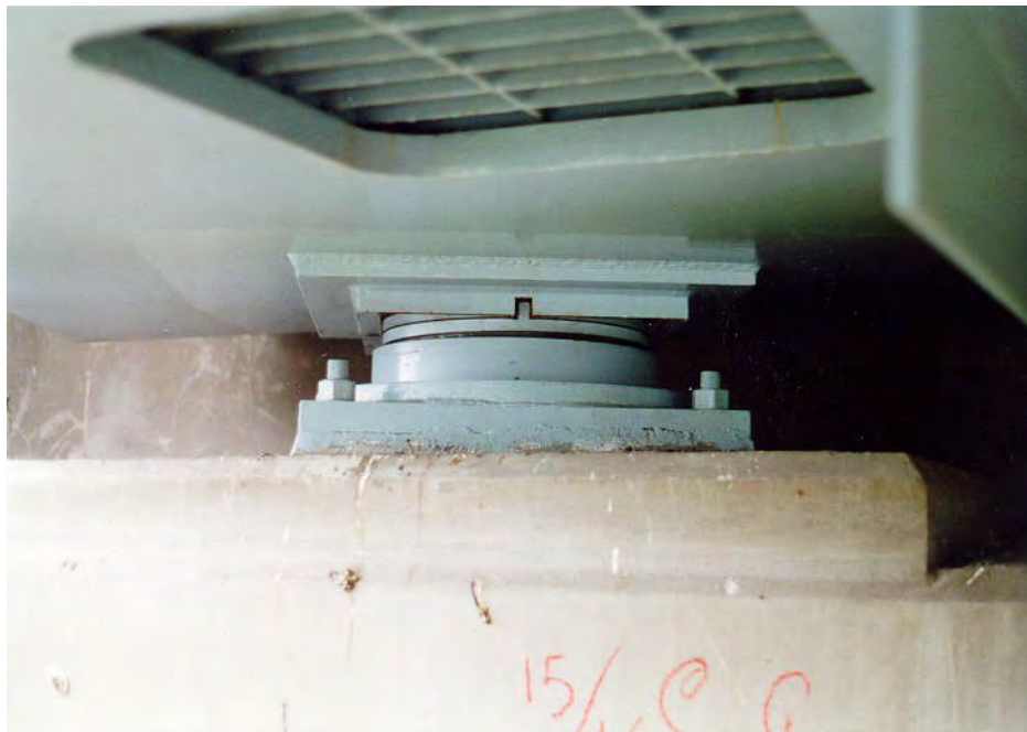
Figure 5.7-15 Center Guided Pot Bearing
