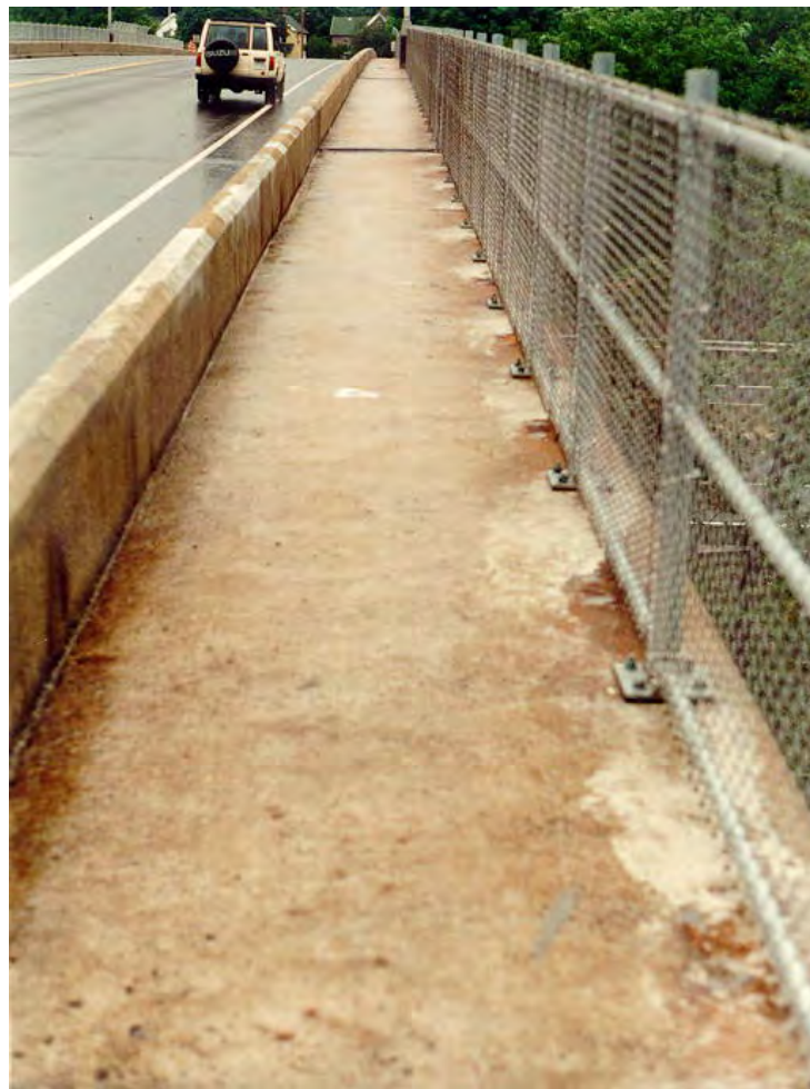
Figure 5.6-7 Concrete Sidewalk with Pedestrian Fence and Traffic Divider.
