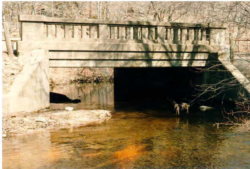
Figure 5.7-21 Typical Concrete Slab Bridge
