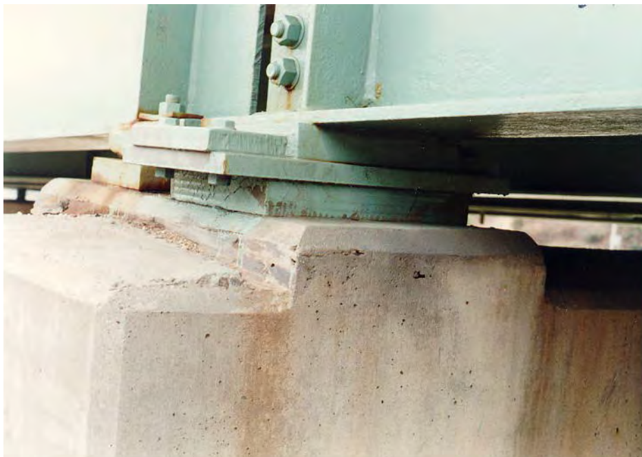
Figure 5.7-11 Retrofit Detail. Elastomeric Bearing Installed
