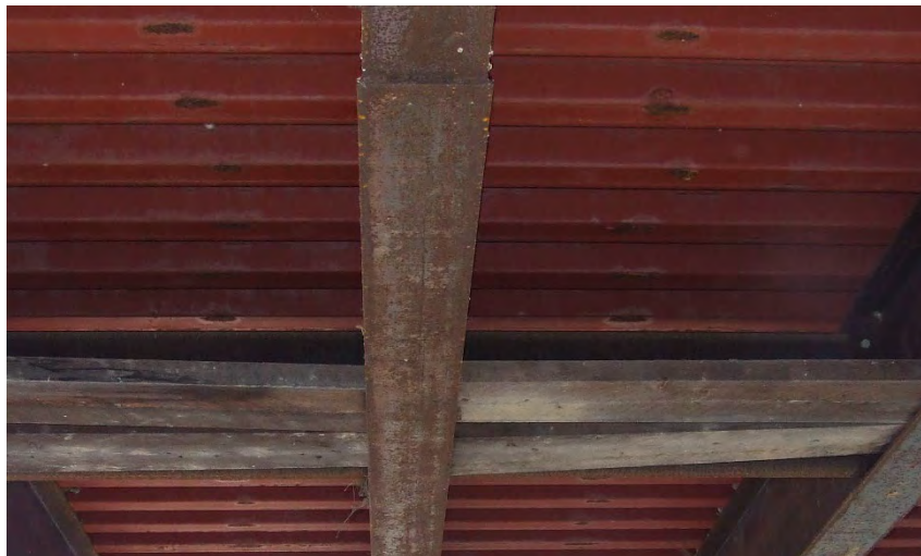
Figure 5.6-4 Underside of Corrugated Metal Deck
