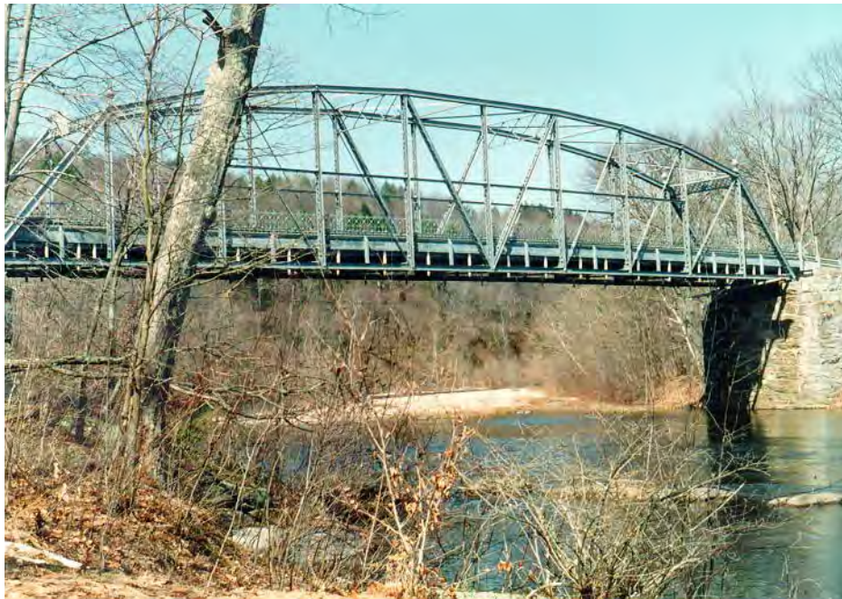
Figure 5.7-34 Historic Steel Through Truss Bridge.
