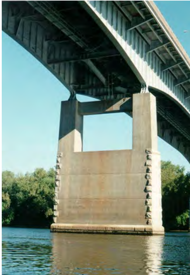
Figure 5.8-2 Tall Concrete Pier with Decorative Stone Masonry Facing
