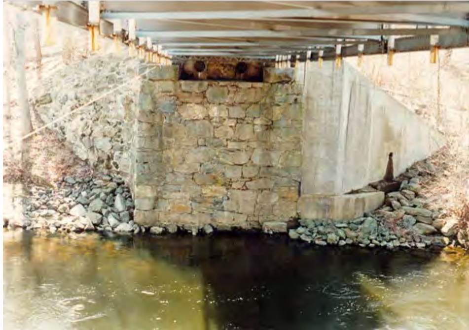
Figure 5.8-3 Tall Stone Masonry Bridge Abutment with Newer Concrete Wingwall Added.
