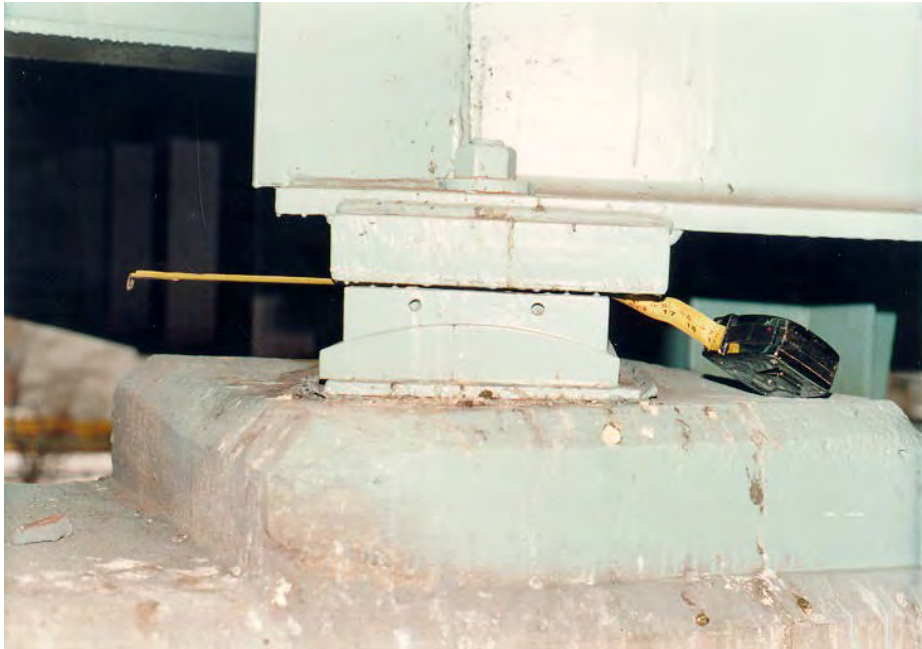
Figure 5.7-10 Bronze Sliding Plate Bearing with a Gap
