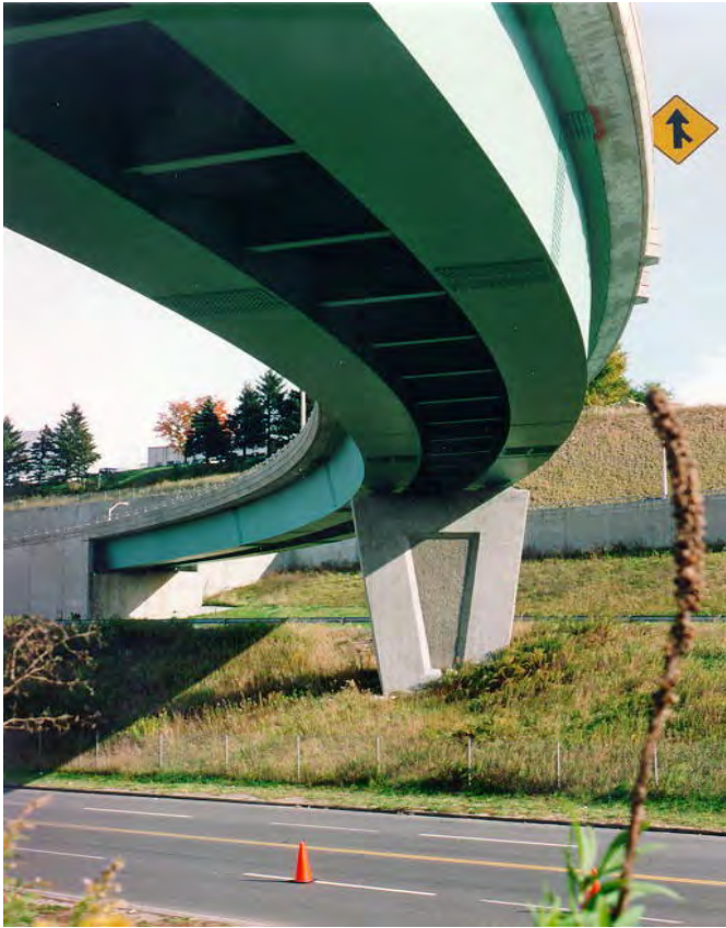
Figure 5.7-32 Curved Steel Box Girder Bridge.
