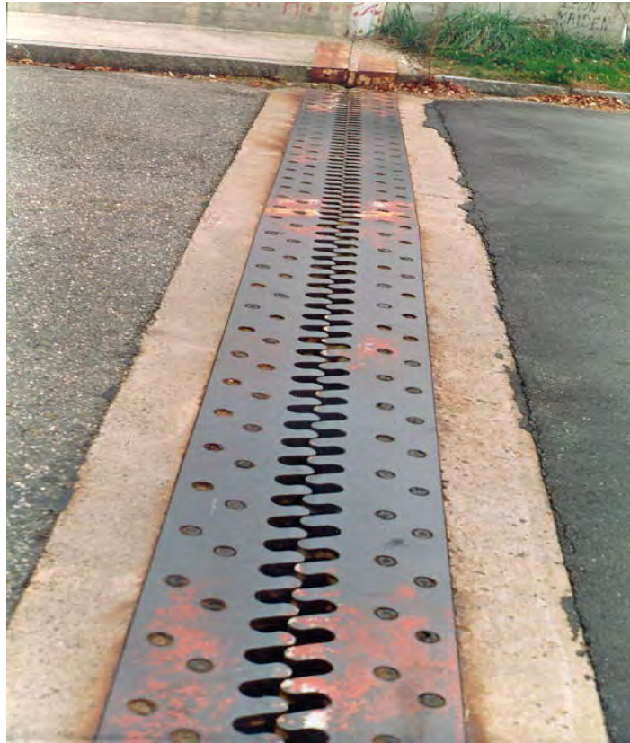
Figure 5.6-11 Steel Finger Joint.
