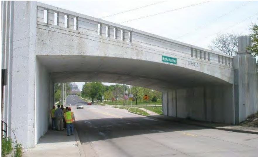
Figure 5.7-24 Single-span Rectangular Concrete Rigid Frame Bridge
