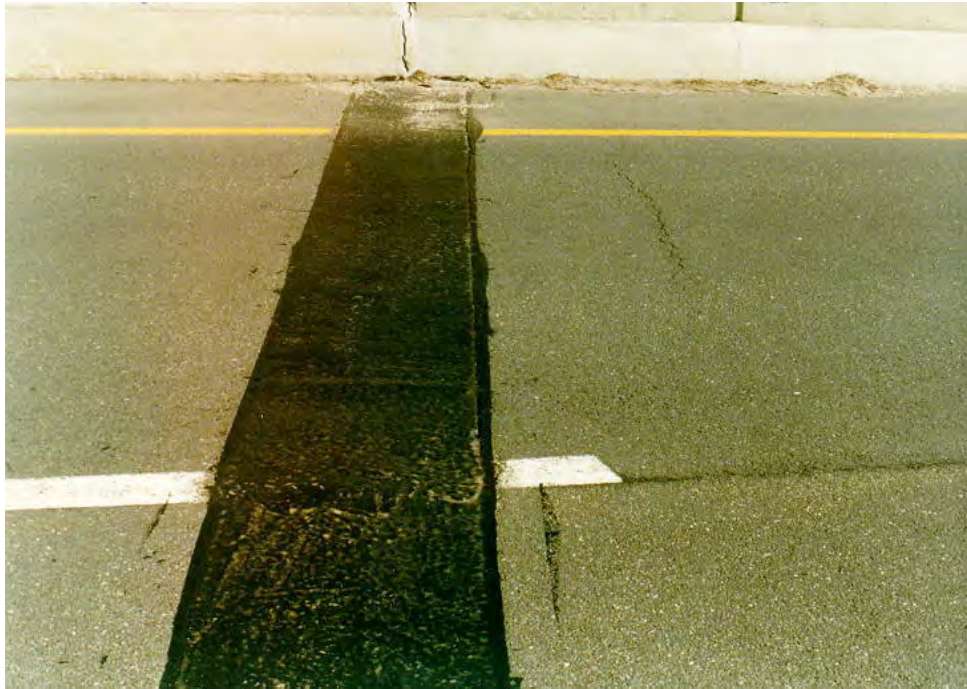
Figure 5.6-12 Asphaltic Plug Expansion Joint.
