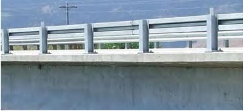
Figure 3.6-3 T-101 Rail on Concrete Deck: B.RH.01 = 3503
