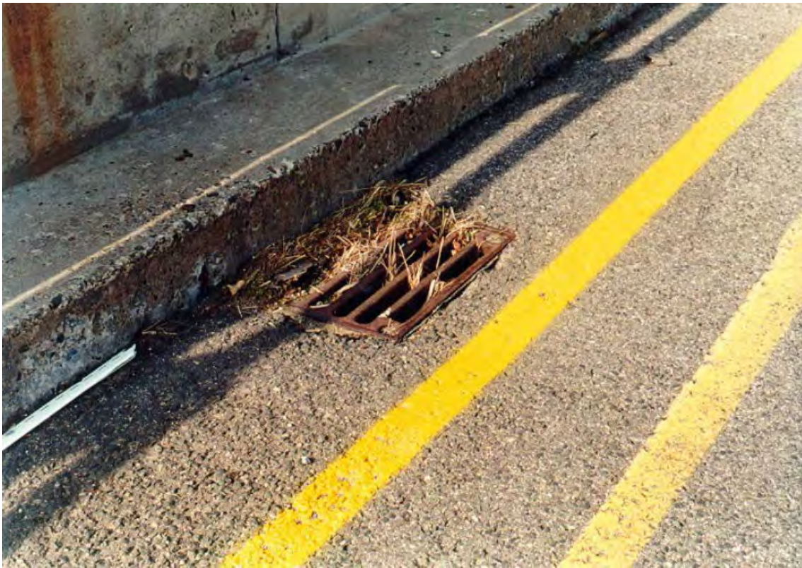
Figure 5.6-6 Typical Concrete Curb with Safety Walk
