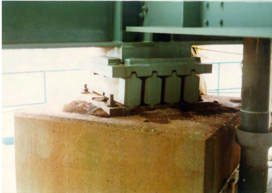
Figure 5.7-12 Nested Rocker Bearing Used for Very Large Spans.
