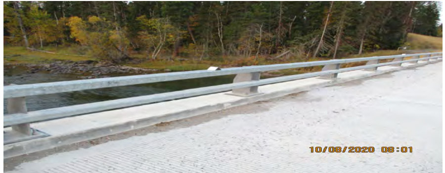
Figure 3.6-6 W830 bridge rail: B.RH.01 = 3504
