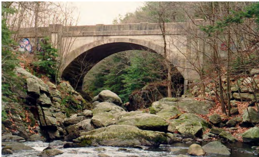
Figure 5.7-23 Figure 5.7.5-1 A Closed Spandrel Reinforced Concrete Arch Bridge
