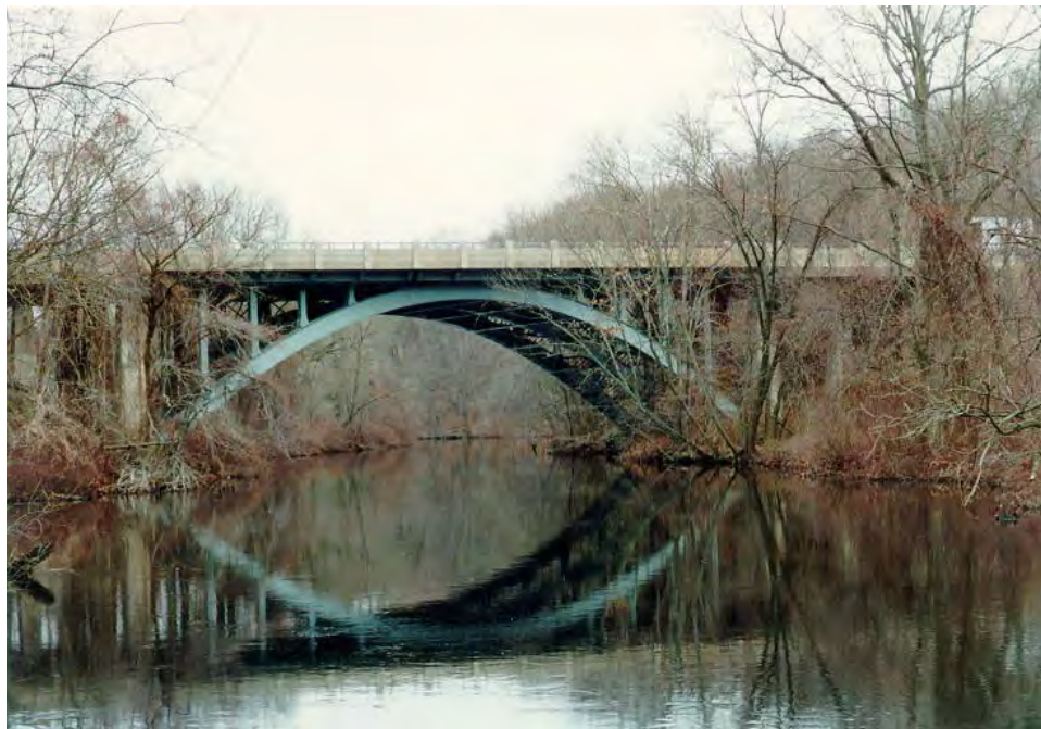
Figure 5.7-35 Steel Deck Arch Bridge.
