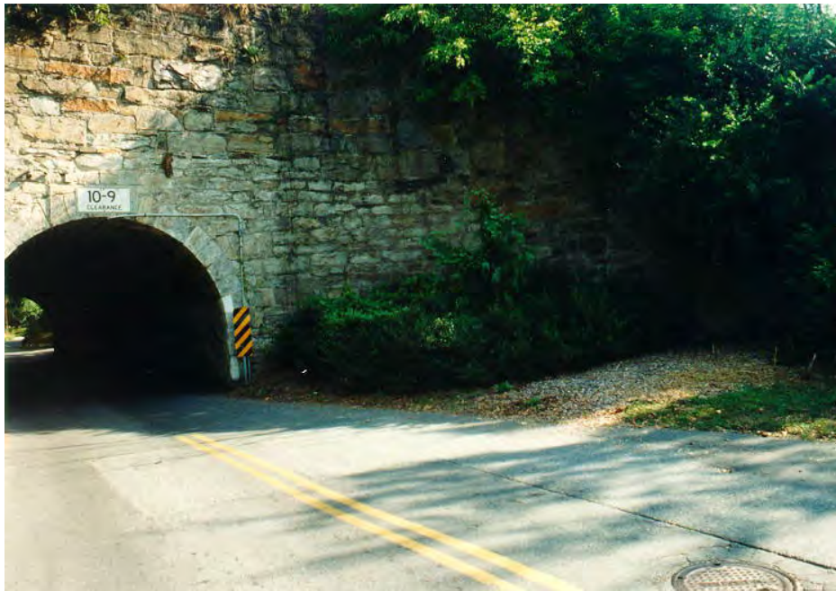
Figure 5.7-39 Stone Masonry Arch and Spandrel Wall
