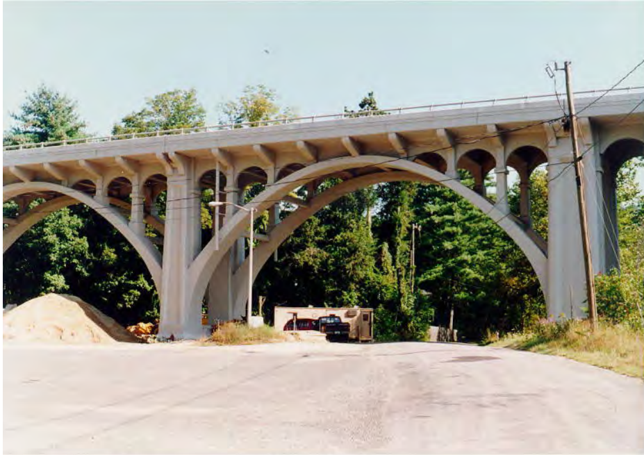
Figure 5.7-25 Open Spandrel Concrete Arch Bridge
