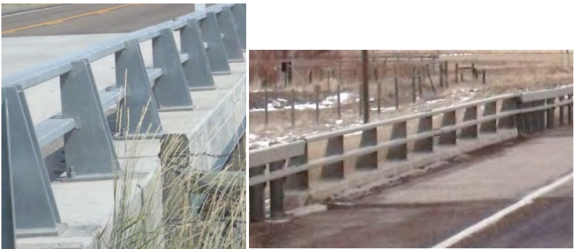
Figure 3.6-5 W740 bridge rail: B.RH.01 = 3503
