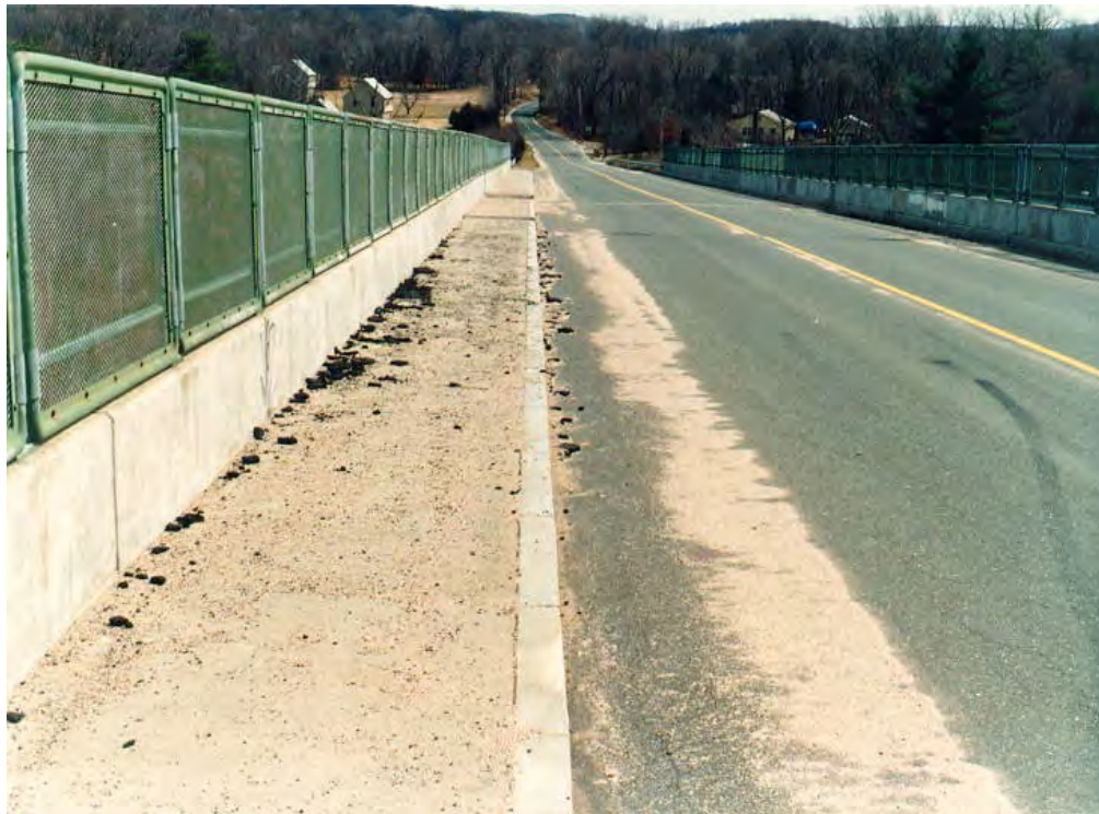
Figure 5.6-10 Pedestrian Fence atop Concrete Parapet.
