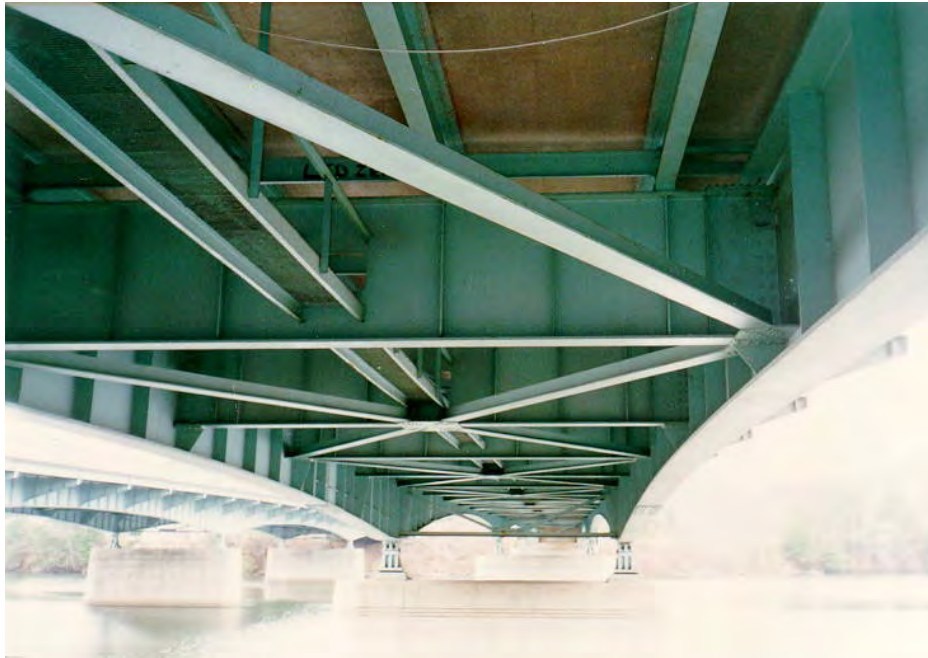
Figure 5.7-30 Typical Framing on a Girder-Floorbeam-Stringer Superstructure.
