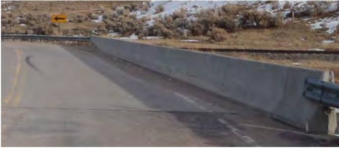
Figure 3.6-4 Concrete Barrier Rail: Code 'I'
