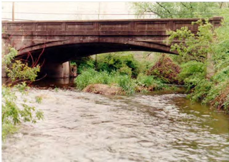
Figure 5.9-2 Sand Bar and Vegetation Growth in the Channel.
