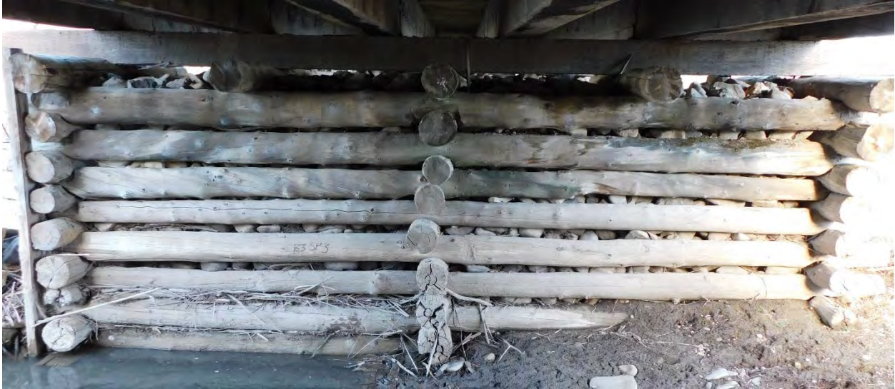
Figure 6.3-9 Timber Cribbing Pier Wall.
