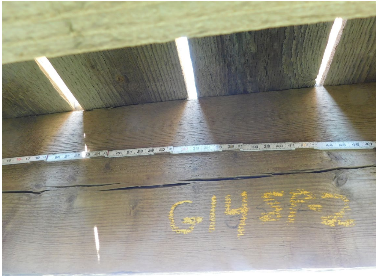
Figure 3.6-2 Example of Beam Checking
