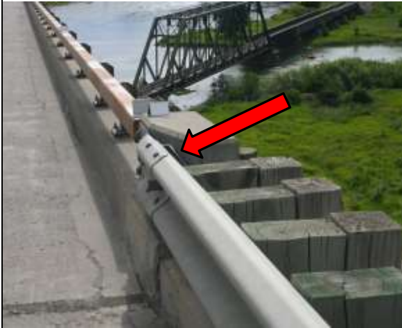
Incorrectly Lapped
