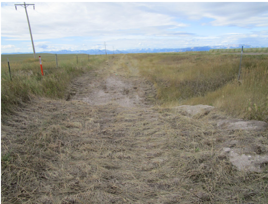
Figure 1: Outlet ditch does not drain
