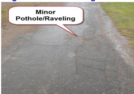
Figure Three: Raveling
