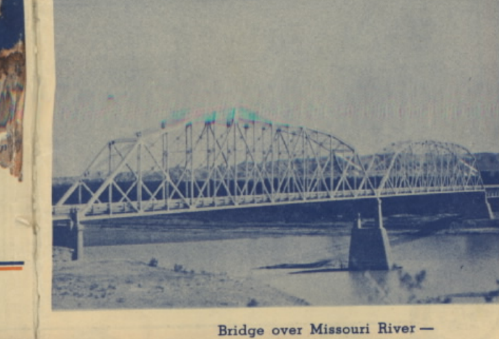
Bridge over Missouri River — Near Culbertson, Montana
