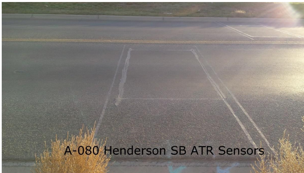
Figure 14 ATR Sensors (Inductive Loop and Piezo) at Henderson Source: Montana Department of Transportation
