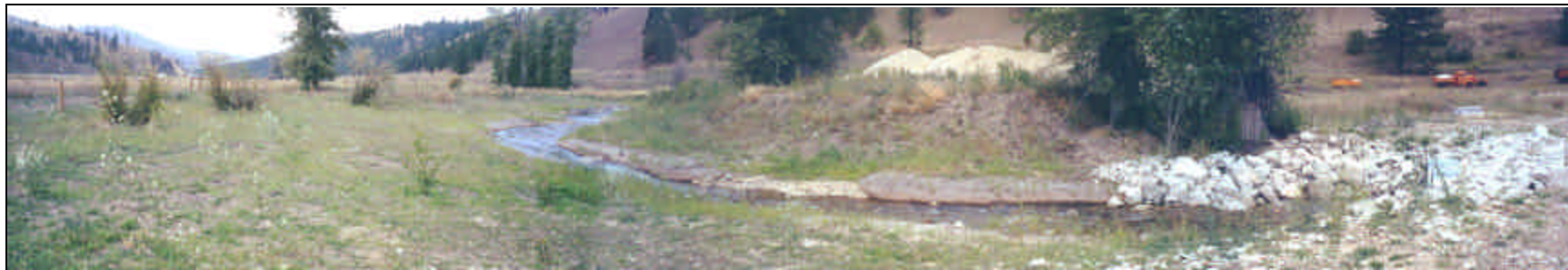
Photo Point No. 11: View looking north along main creek, below upper road crossing and culvert near Grasser complex. Mature cottonwoods and remnant shrub communities present along creek. Example of intact fabric work along streambank, floodplain margins planted with riparian shrubs and trees.
