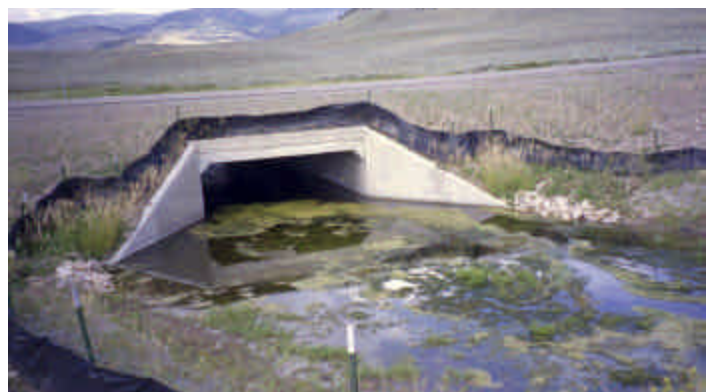
Photo Point 6: 15 degrees North Culvert under highway where creek leaves the analysis area.
