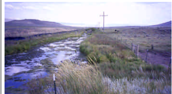
Photo Point 6: 90 degrees East Stream channel parallel to highway at west end of analysis area.
