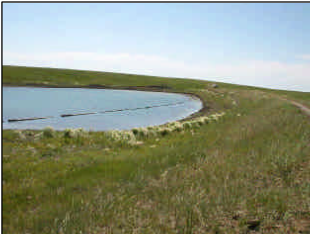
Location: C Description: Wetland buffer Compass Reading: 280°
