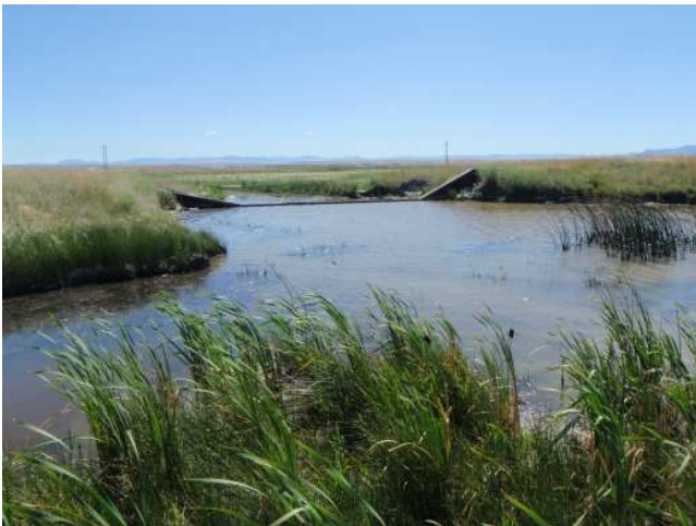
Photo: Weir structure Bearing: 150 Degrees
