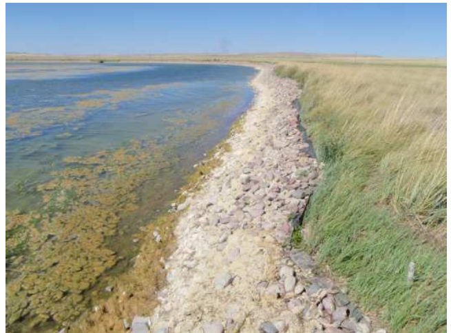
Photo: Rock toe Bearing: 0 Degrees
