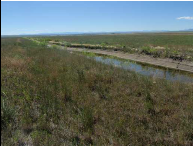
Photo Point 3 – Photo 1 Location: Inlet canal Bearing: 130 Degrees Taken in 2010
