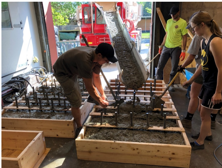
Figure 26: Placement of the Slabs
