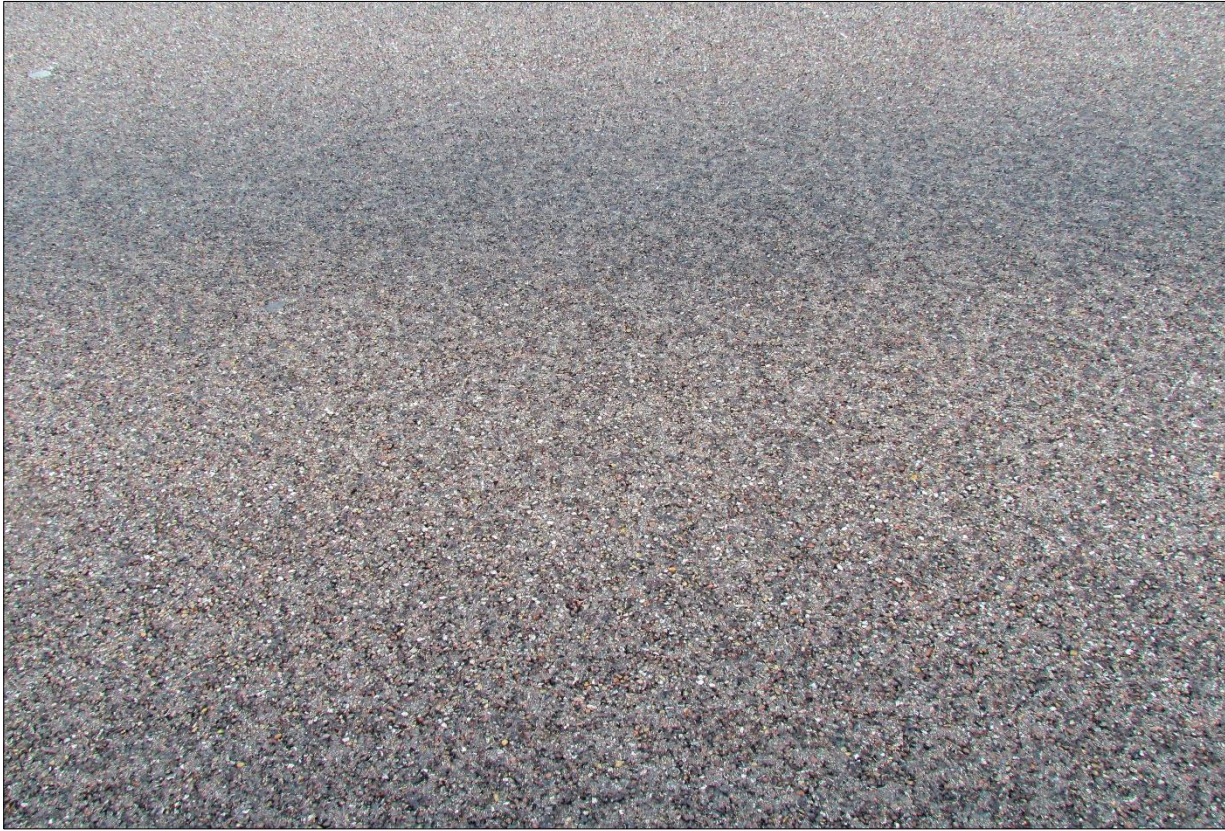
↑↓ Representative images of the 3/8" AC section pavement texture (surface was slightly wet).
