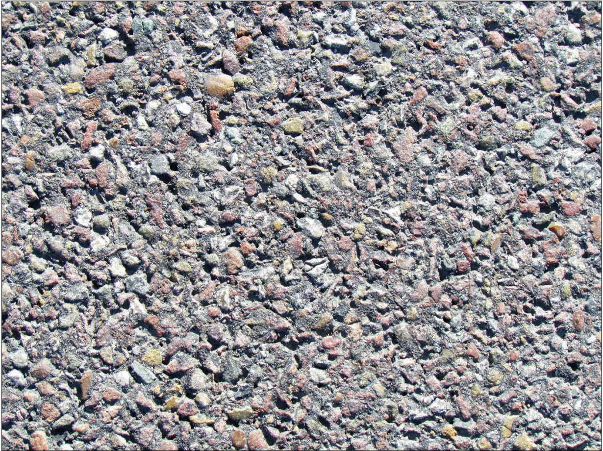
↑ Closer view of pavement texture.
