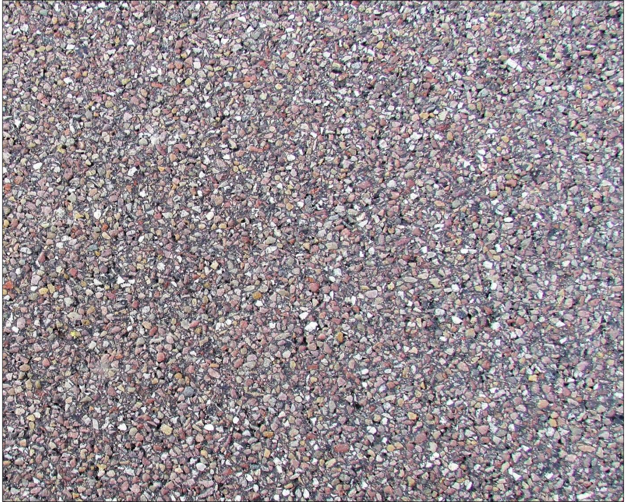
↑ Representative image of the 3/8" AC section pavement texture.
