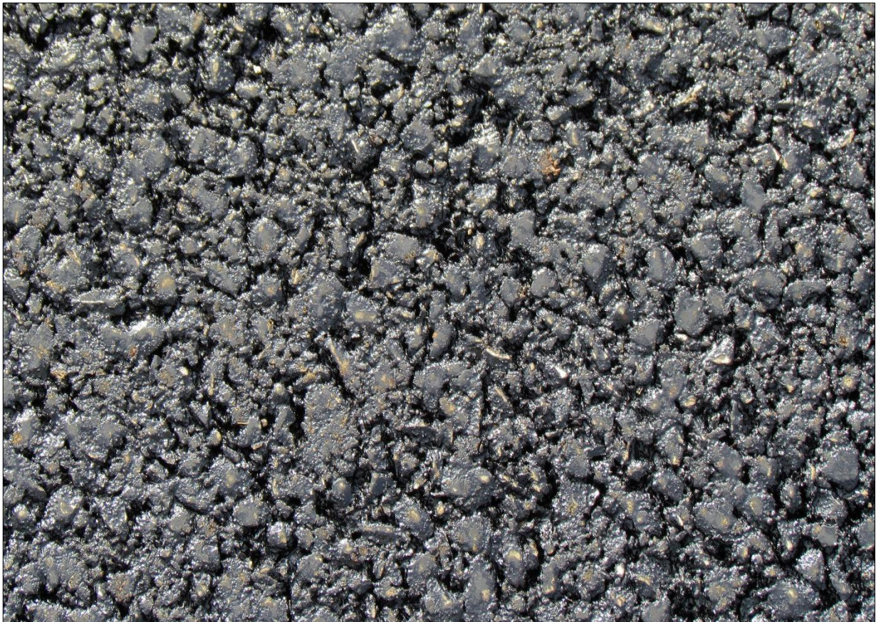
↑↓ Representative images of the 3/8" AC section pavement texture.
