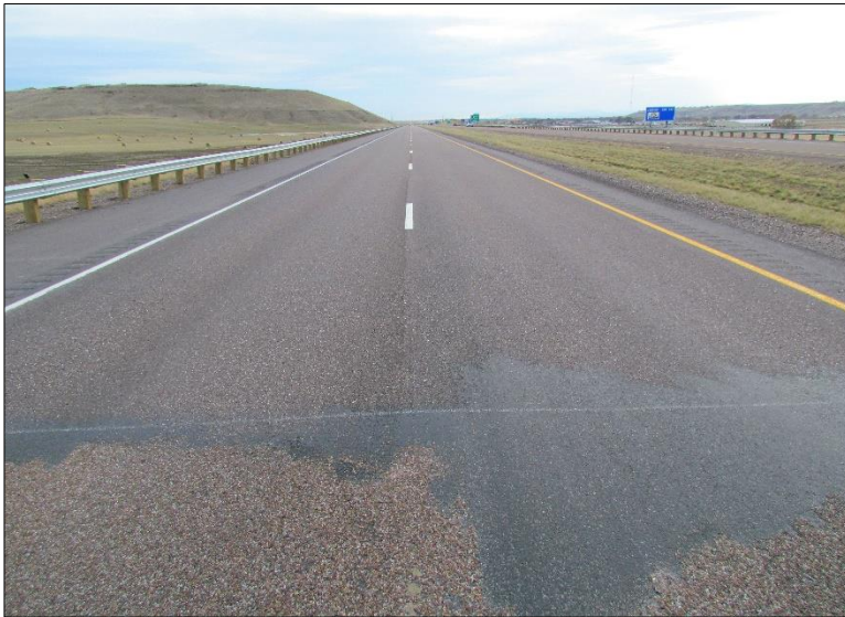
← View south at transition of chip seal and 3/8" section.
