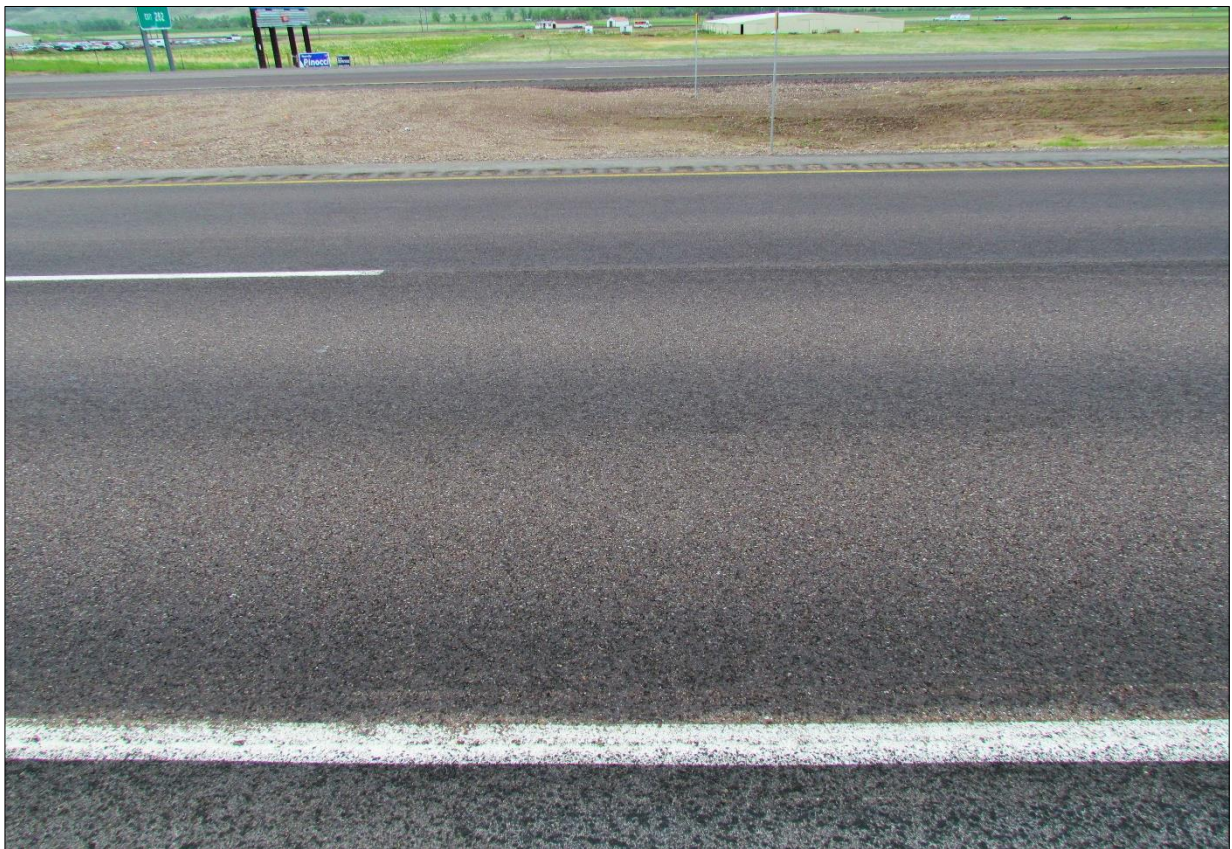
↑↓ Representative images of the 3/8" AC section at approximate reference point 282.5; upper view is northbound I-15 view north, lower image transverse view.
