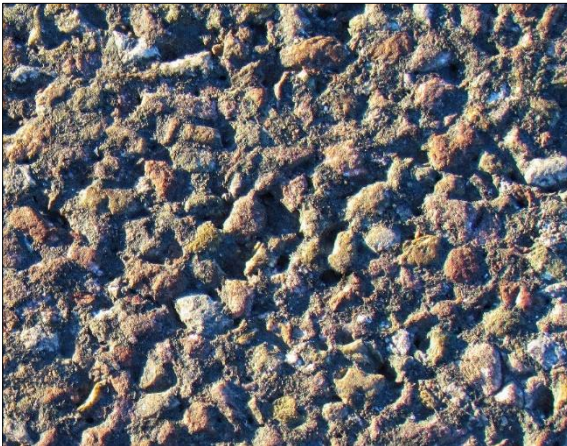
← Close-up of the 3/8" AC section pavement texture on January 2019 .
