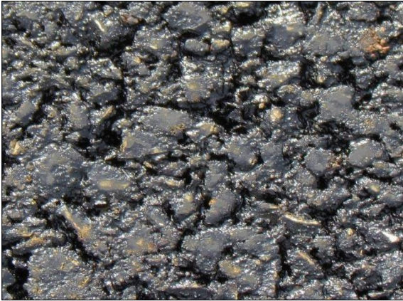
← Close-up of the 3/8" AC section pavement texture on November 2017 .
