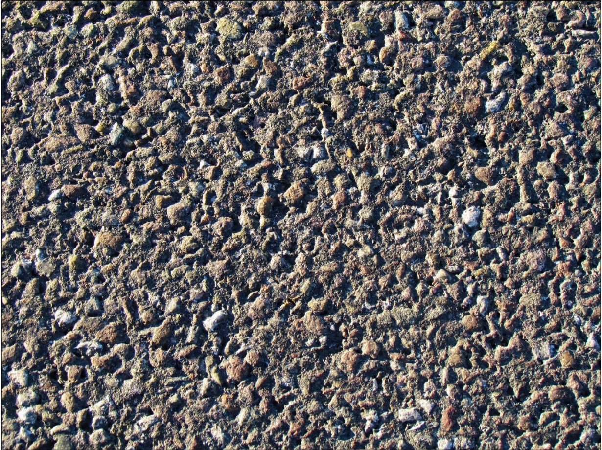
↑ Representative image of the 3/8" AC section pavement texture.
