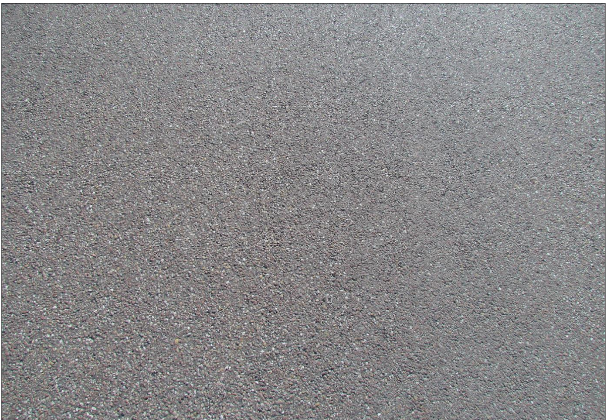
↓ Representative image of the 3/8" AC section pavement texture.
