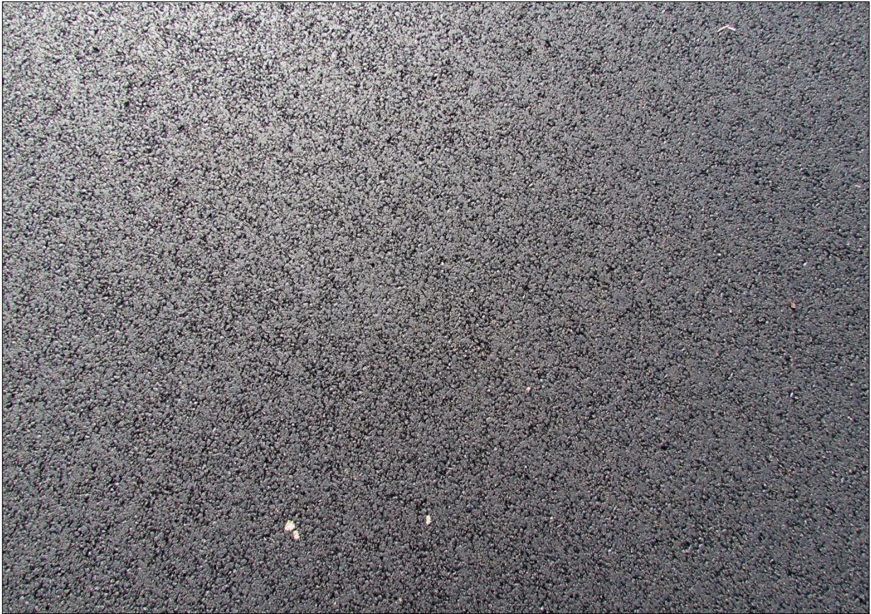
↑↓ Representative images of the 3/8" AC section pavement texture.
