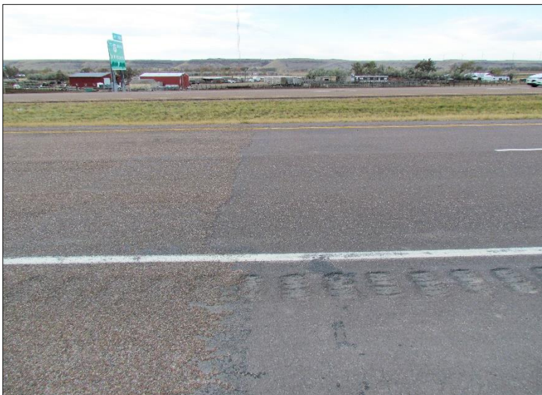
← Transverse view of 3/8" section (south end).
