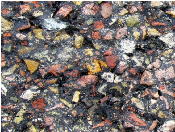
← Close-up of the 3/8" AC section pavement texture on May 2018 (Note: pavement was damp when image was taken).
