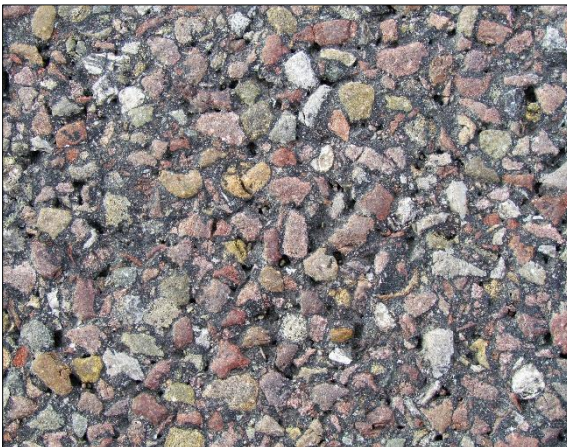
← Close-up of the 3/8" AC section pavement texture on October 2019 .
