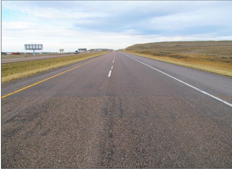
← View north at transition of chip seal and 3/8" section; approximate reference point 282.
