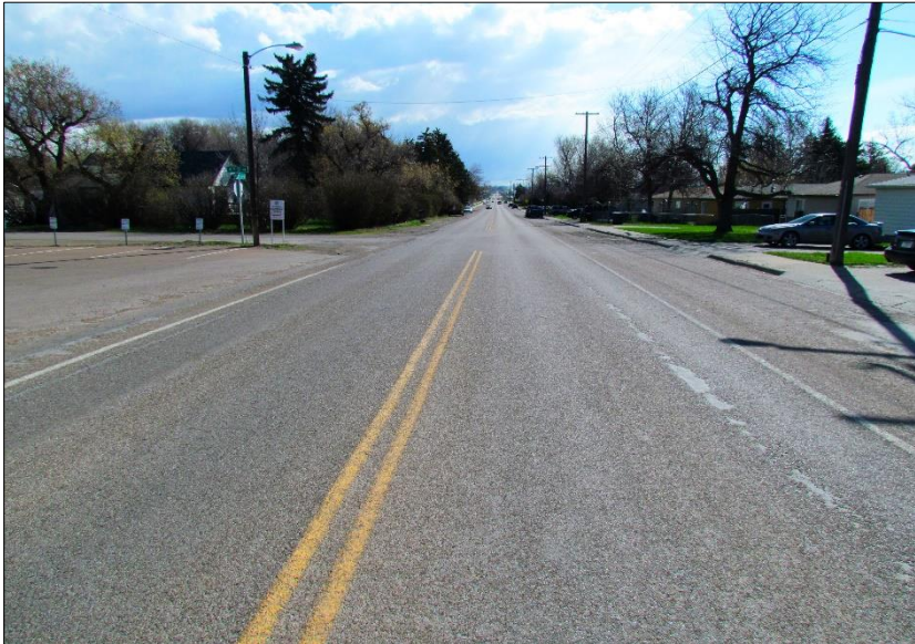
← West end of project; view east.
