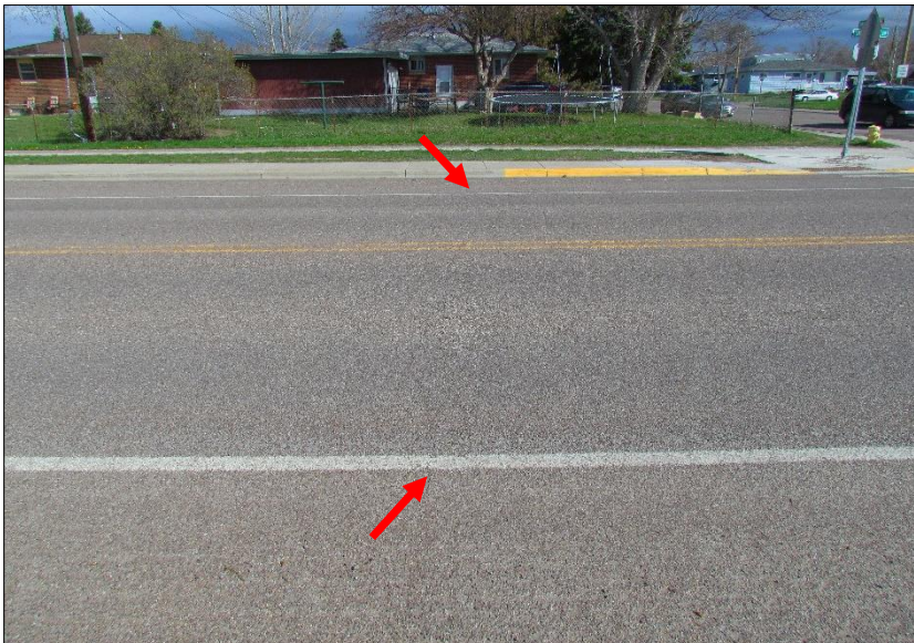
← Although difficult to see in this image; one low- severity longitudinal crack has appeared on the project near Riverview B intersection (red arrows).
