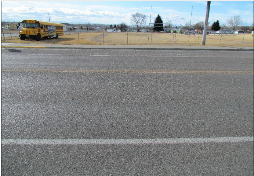
← Transverse view of pavement.
