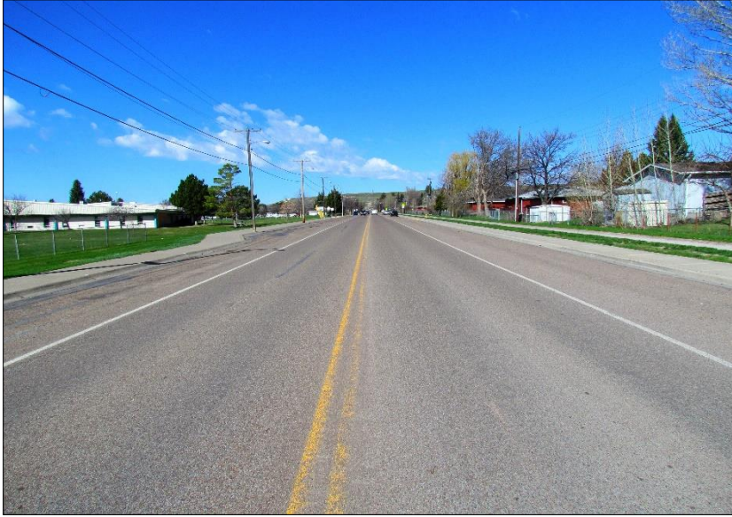
← East end of project; view west.
