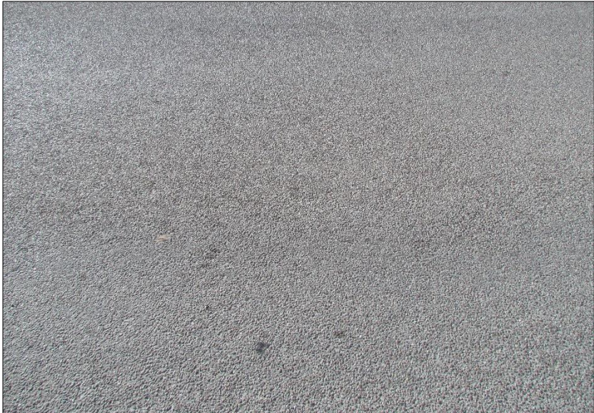
← Example of pavement surface condition.
