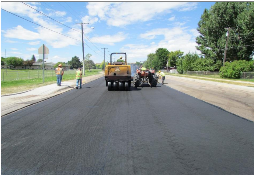
← The second pass of fabric being applied. Note the pneumatic roller insure a direct pass over the overlapping geotextile seam.
