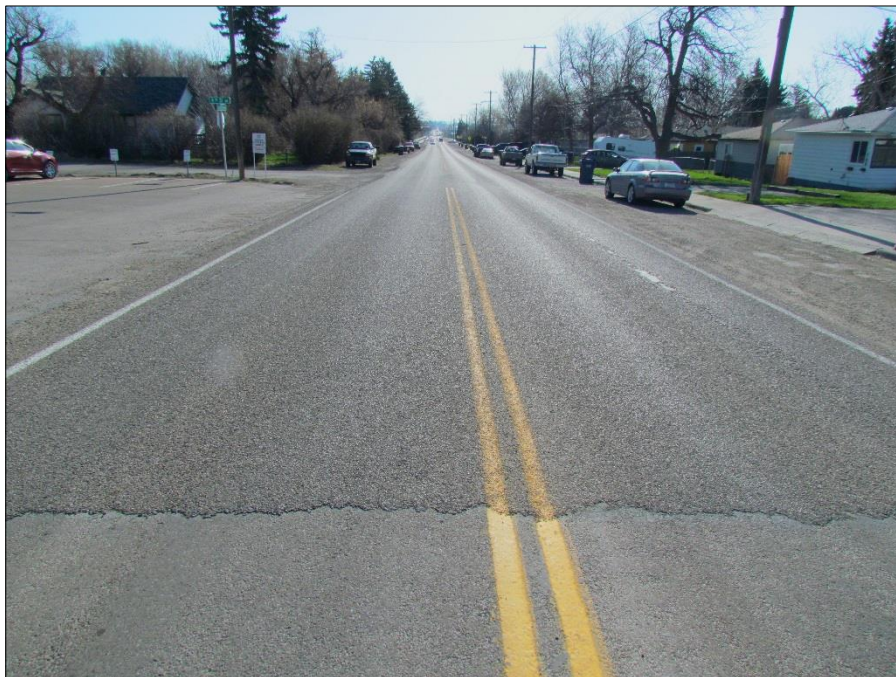
← West end of project; view east.
