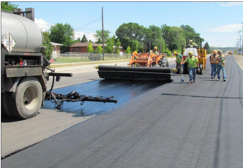
← View of fabric placement at front end of geotextile train.
