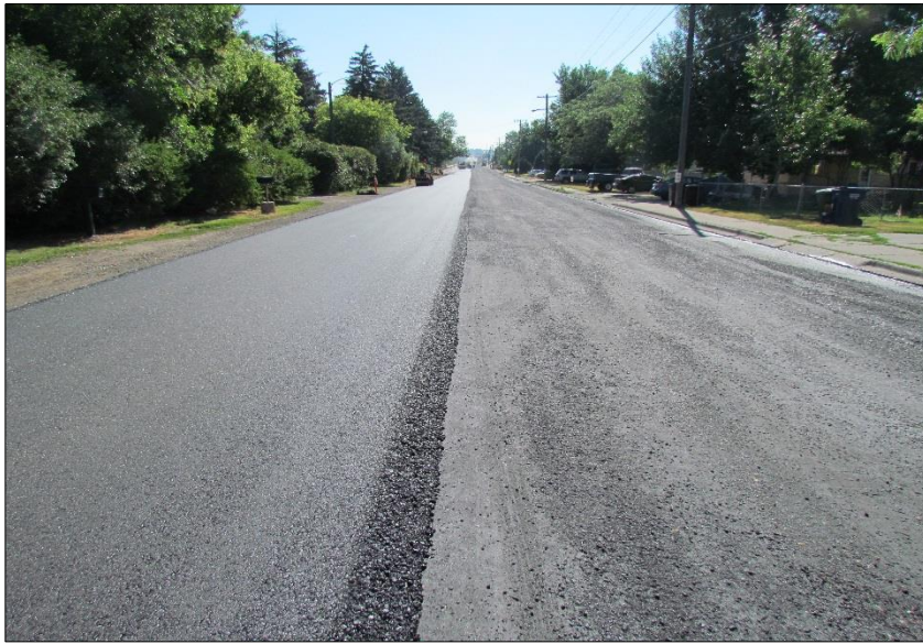
← Representative image of completed paving pass; view west.
