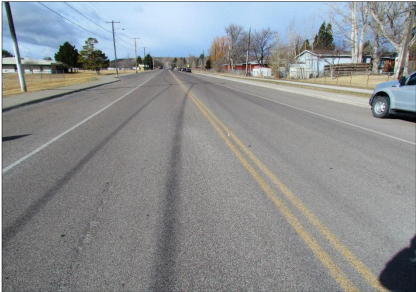
← East end of project; view west.
