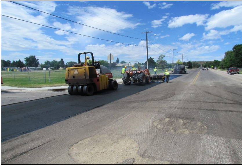
← As the first pass begins a pneumatic compactor 9-wheel roller follows close behind to insure good adhesion to the fabric, tack coat and underlying pavement.
