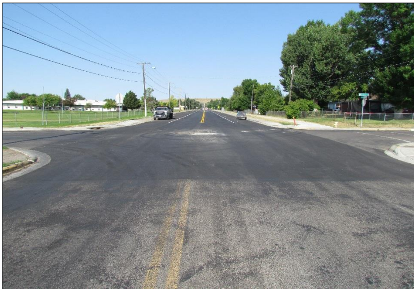
← Completed project; east end, view west.
