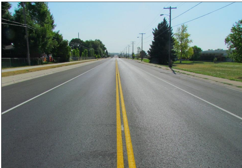
← Completed project; west end, view east.
