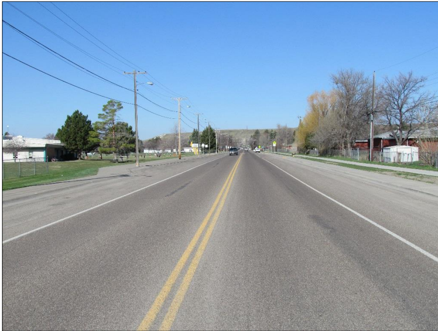
← East end of project; view west.
