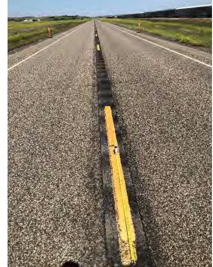
View to the north of SCLRS Design S2 (24"LF, 12"wide) and strike zone cone markers.
