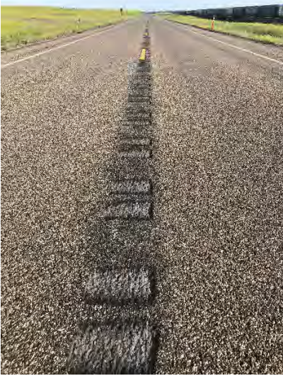
View to the north of the Standard CLRS and strike zone cone markers.
