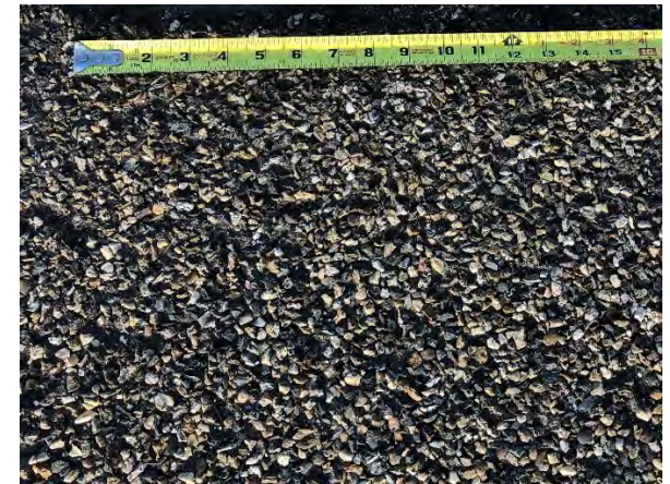
View of the MT-39 pavement (3/8" aggregate chipseal) installed in 2011.
