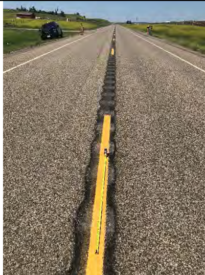
View to the north of SCLRS Design S3A (24"LF, 14"wide) and strike zone cone markers.
