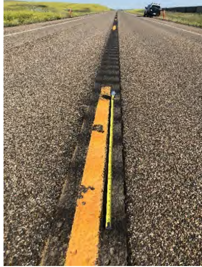
View to the north of SCLRS Design S1 (14"LF, 12"wide) and strike zone cone markers.
