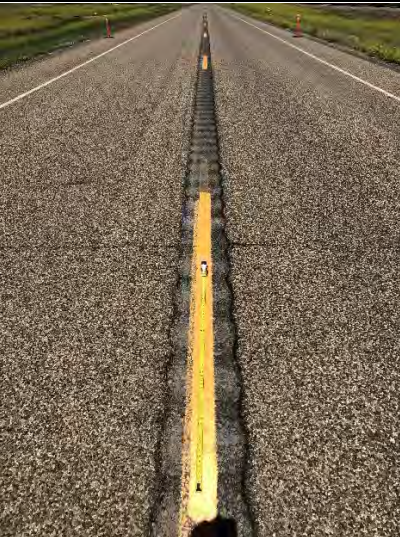
View to the north of SCLRS Design S3 (14"LF, 14"wide) and strike zone cone markers.
