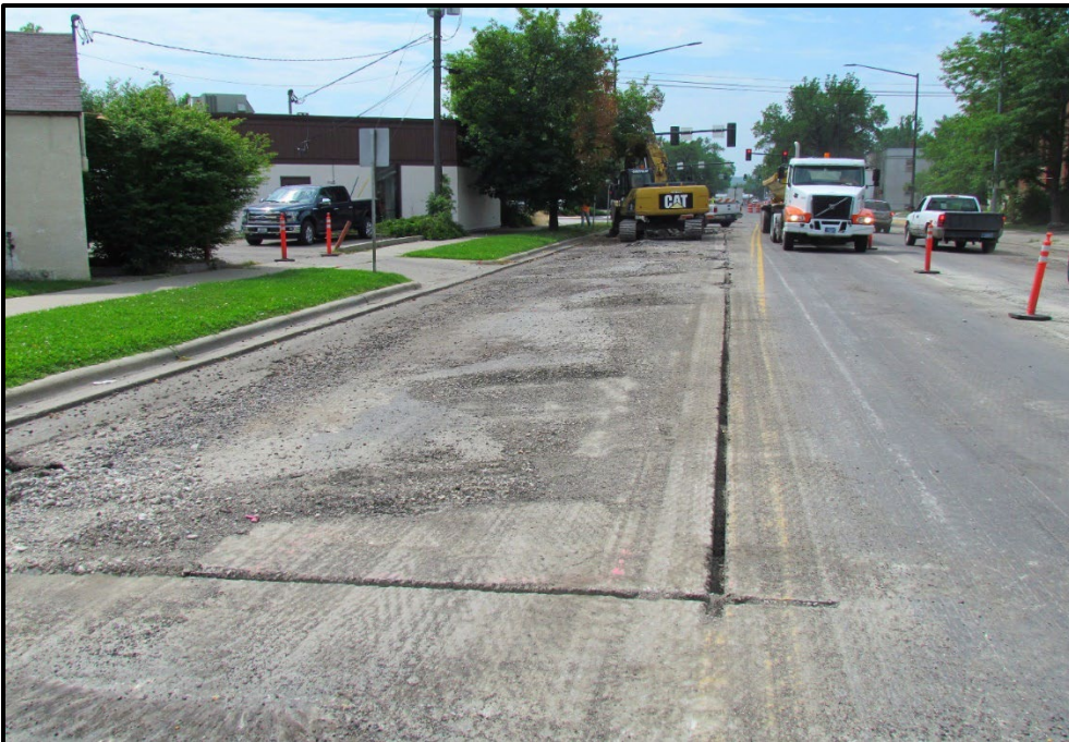
↑ After milling, several sections of pavement needed full depth replacement.
