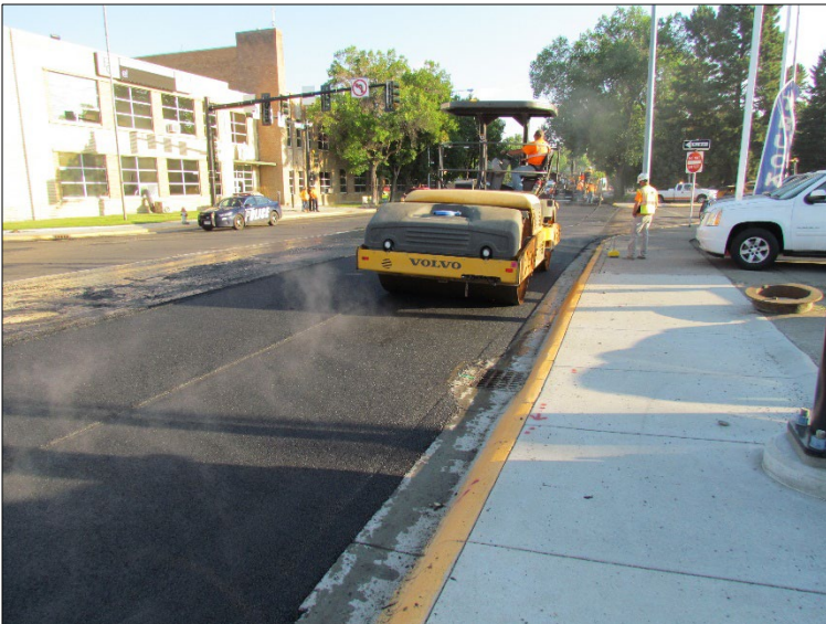
← Double steel drum rollers were used for compaction.
