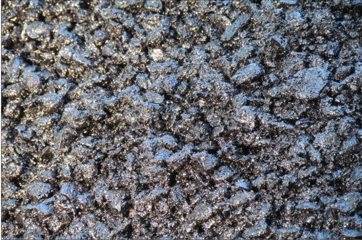
↑ Close-up of uncompactied FRAC. The fibers were not noticeable in the mix, however if you handled and separated the aggregate, the fibers were visible.
