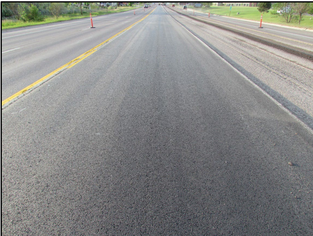
↑ View of the roadway during the paving operation.
