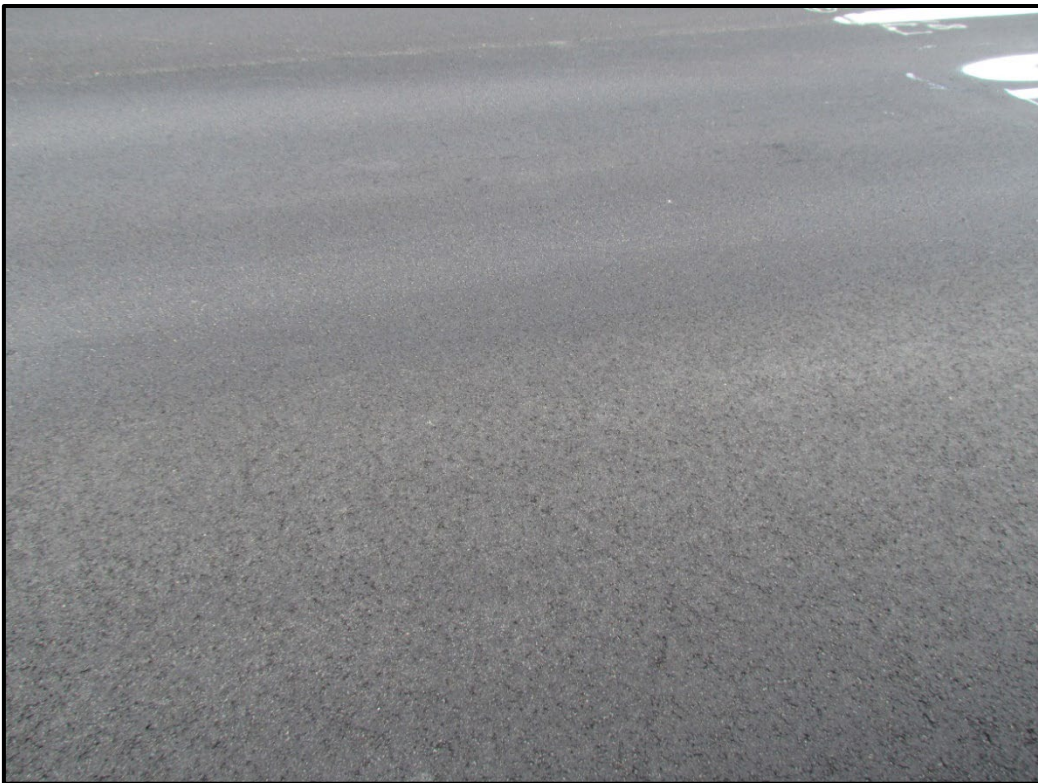
↑ Close-up of the plant mix surfacing.
