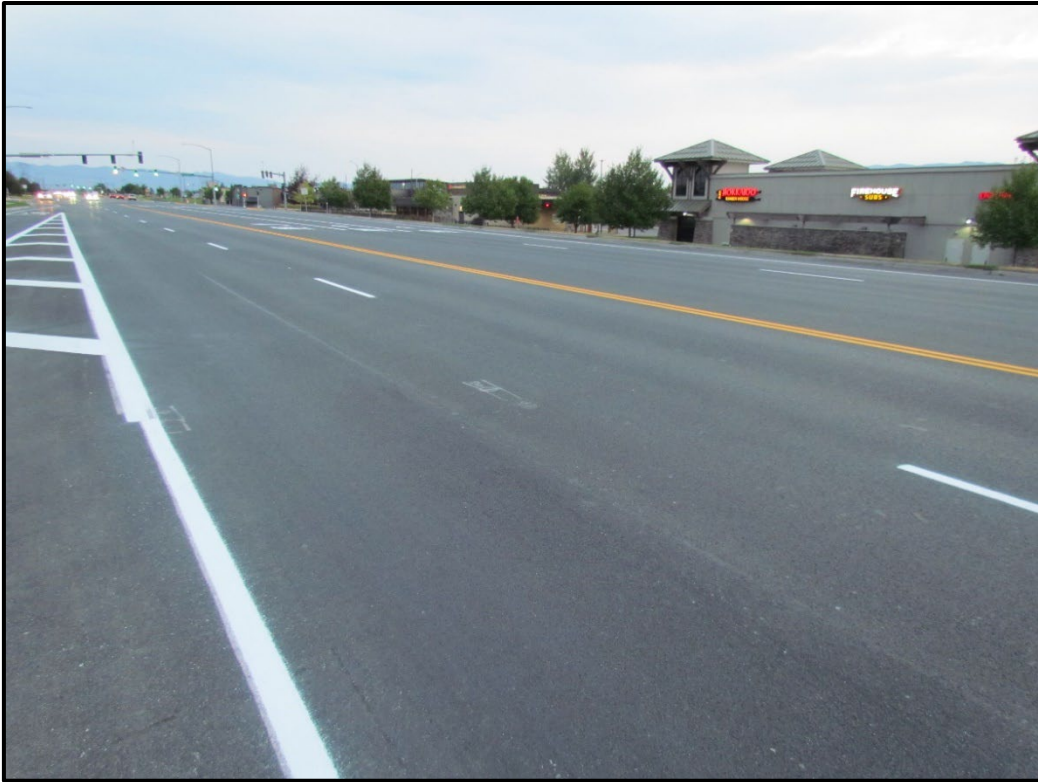
↑ View north of the finished project.
