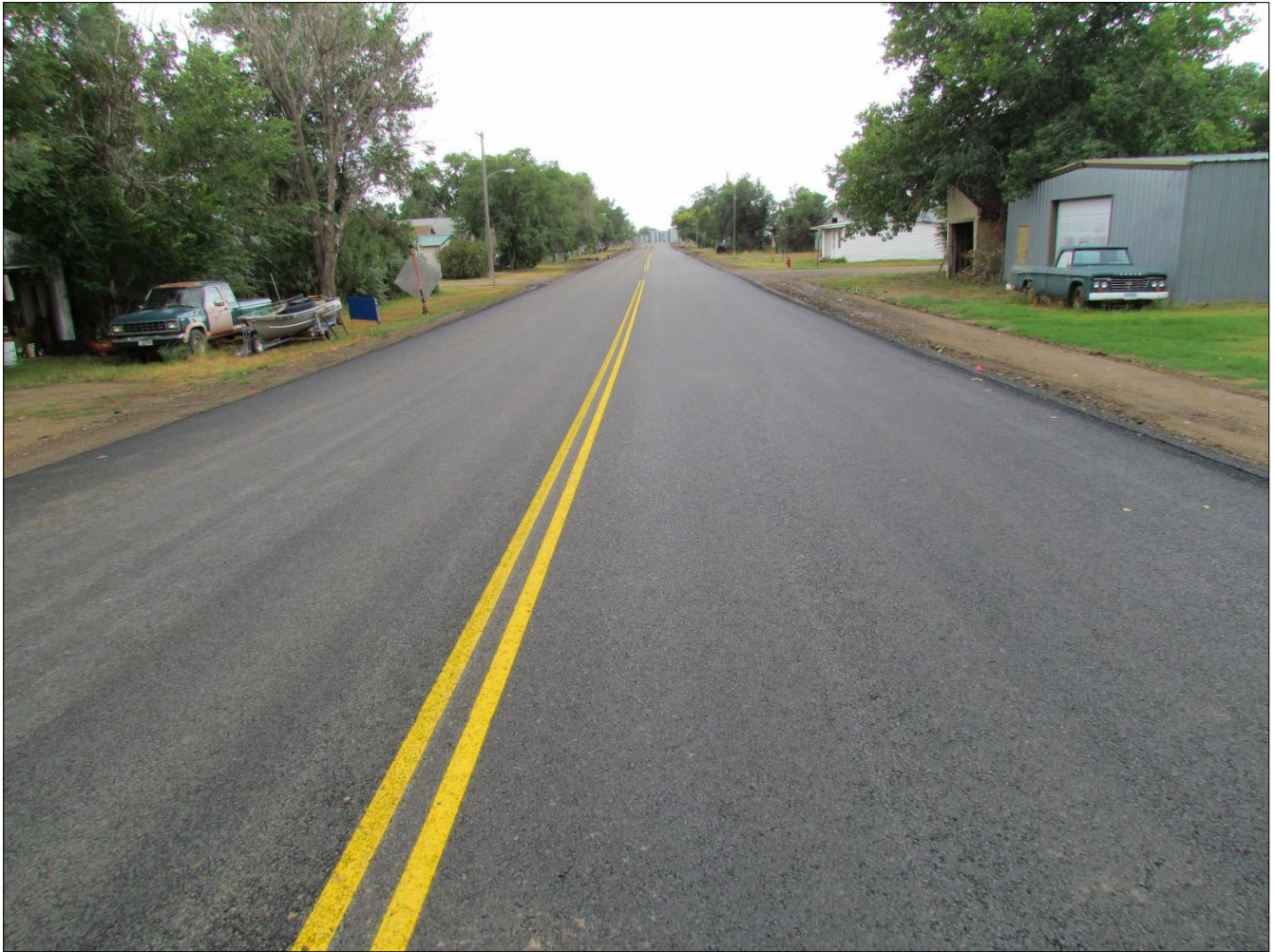
↑ Representative image of completed paving phase of project (Section 6 - Sargent St.) view south.
