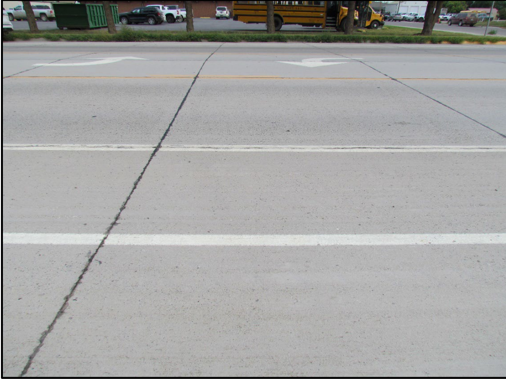
↑ MT Hwy 200 and Western Ave intersection, test section, transverse view
