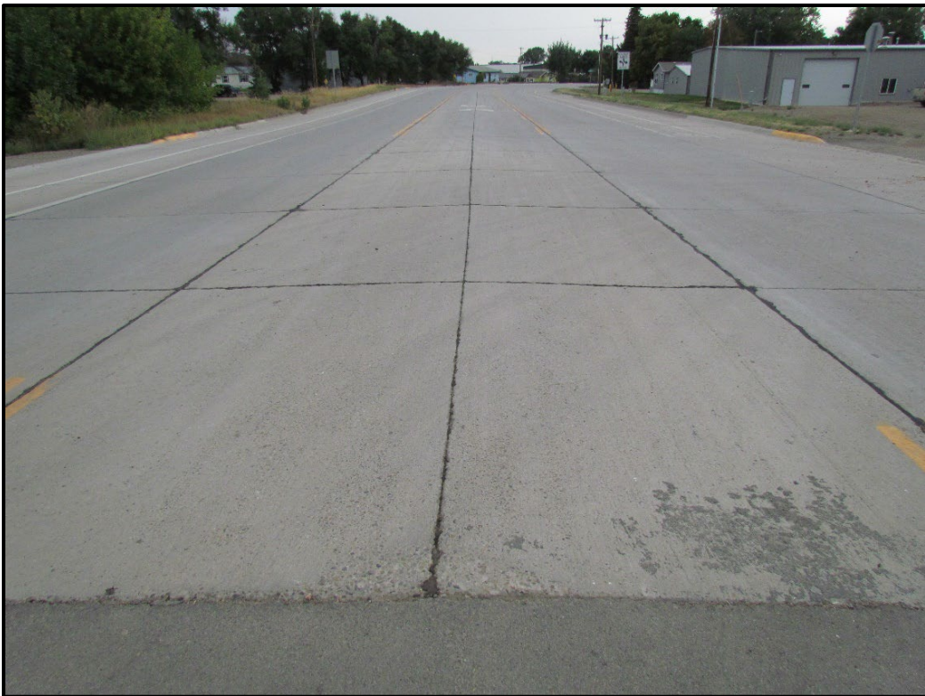
↑ South end of project, view north.
