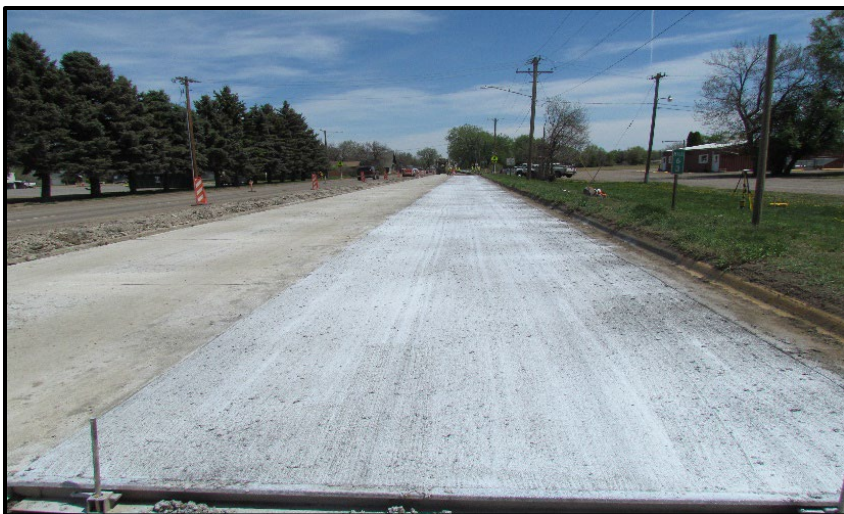
← PCCP section that is completed and curing compound placed.
