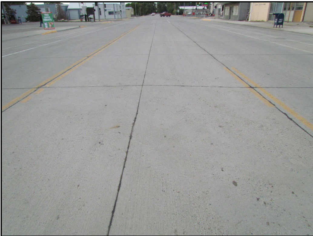
↑ MT Hwy 200 and 6 th St intersection, test section, view south.
