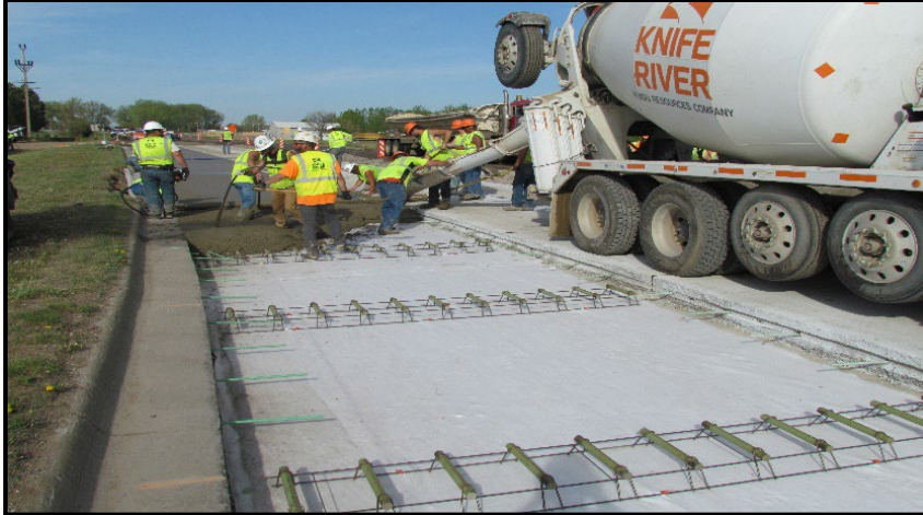
← PCCP placement in driving lane and bike lane.
