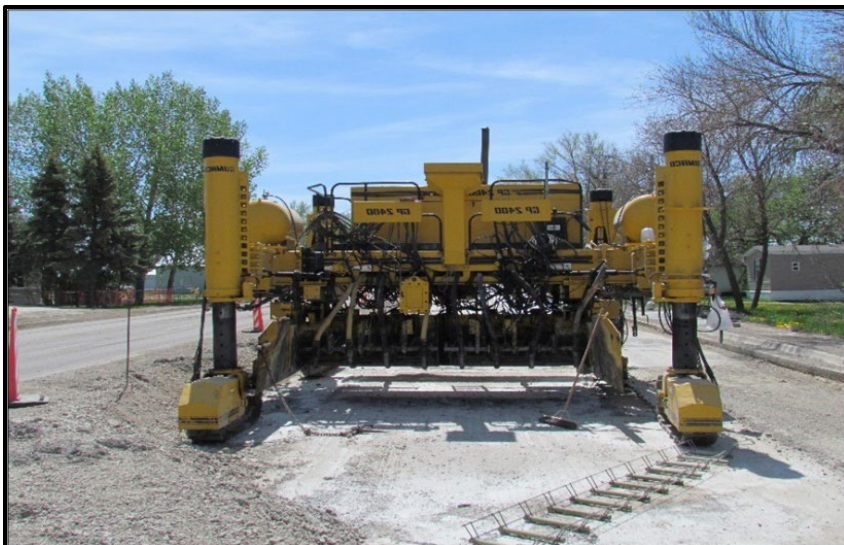
← GOMACO GP 2400 concrete paver for the median portion of operation.
