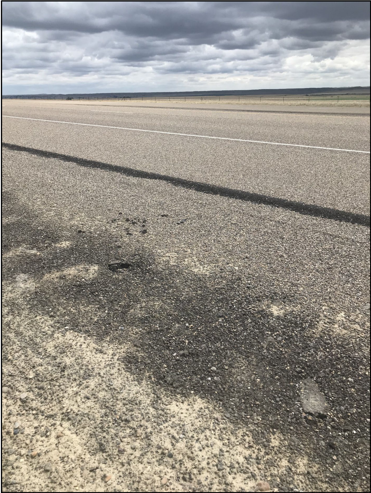
↑ RP 197.60, view east. Westbound shoulder, test section, typical 1.
