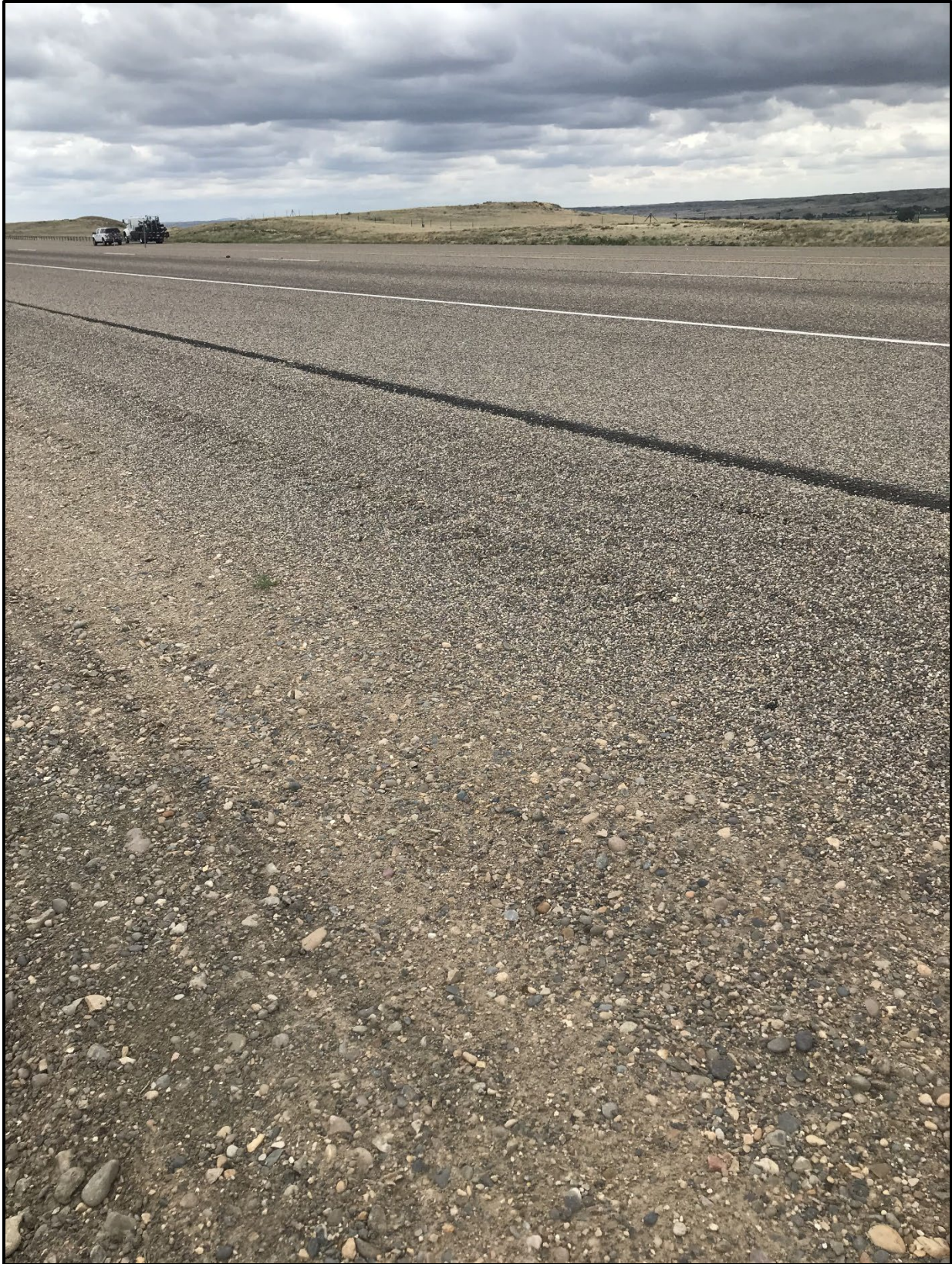
↑ RP 193.50, view east. Westbound shoulder, test section, typical 1.
