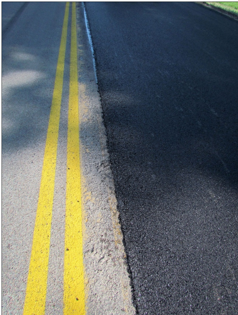
← Example of compacted AC at longitudinal centerline.
