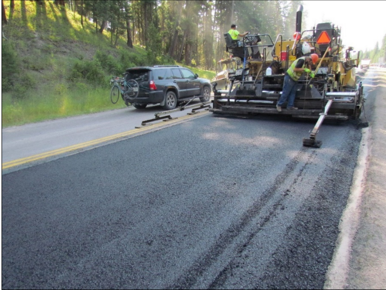
← Start of the southbound paving phase.
