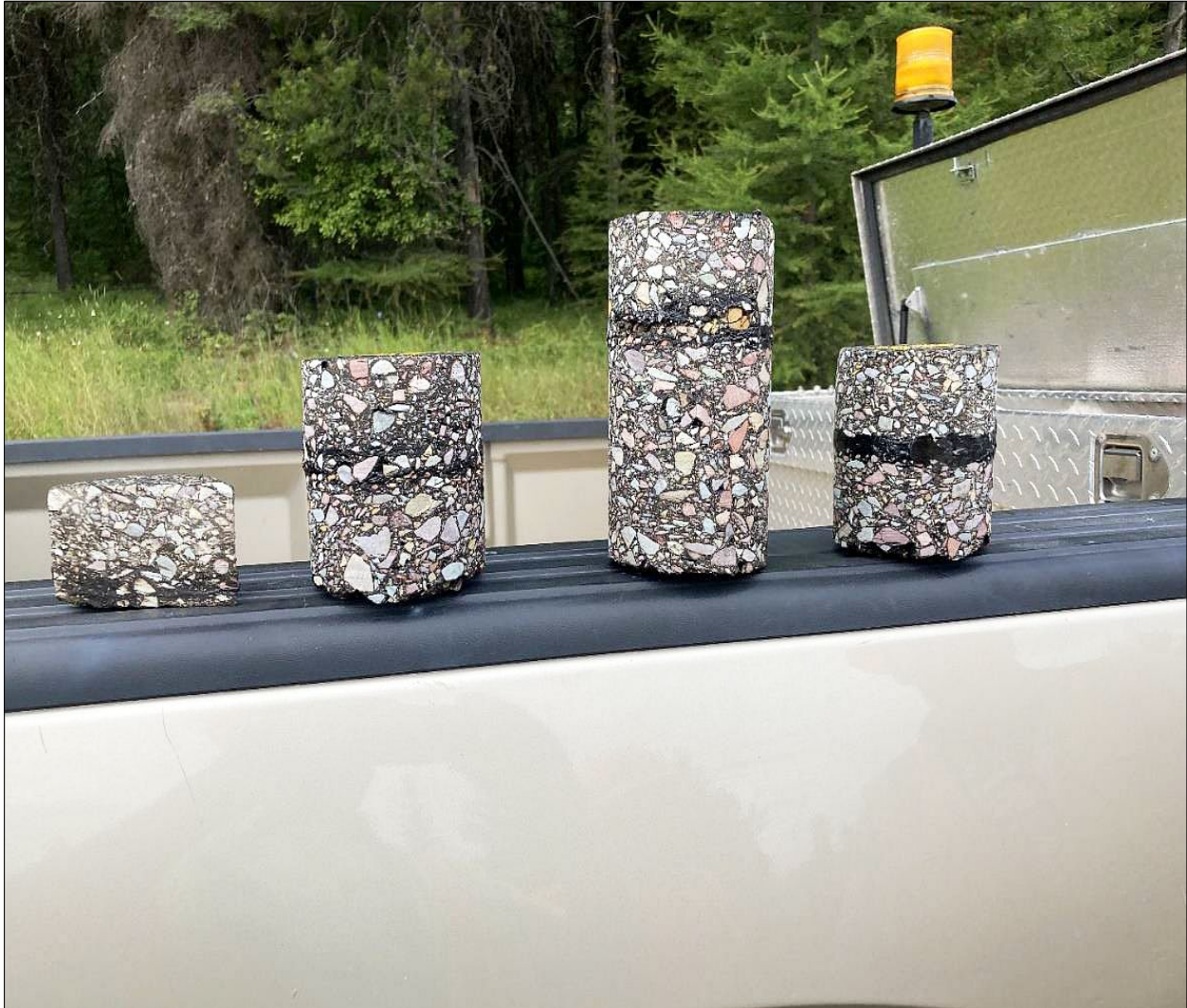
↑ Several core samples taken from the projects centerline which shows the extent of the VRAM migration into the AC matrix. The core on the far left is split. Image courtesy of CES Review Section.
