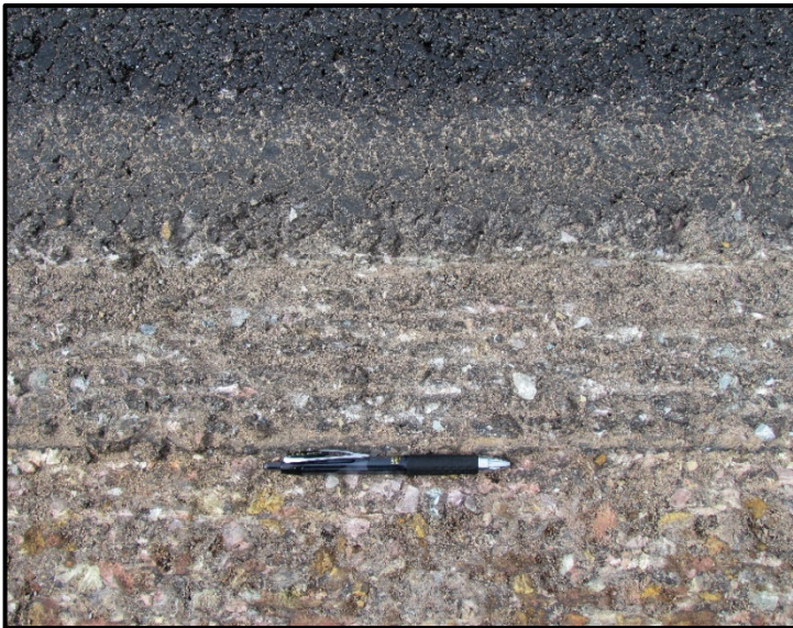
← This image shows the mill pass that has cut into the southbound lane JBAND strip. The pen marks the edge of the JBAND strip.
