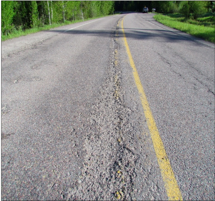
↩️⬇️ Several examples of centerline joint condition prior to start of project. Top image is near RP 32, lower is near RP 43.
