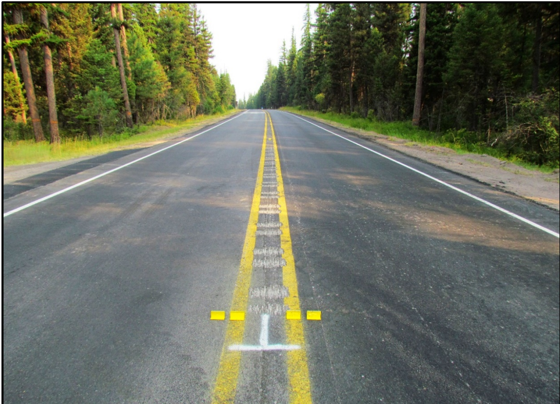
↑ Northbound lane paving completed. ↓ Project with temporary striping and centerline rumble strip. Chip seal was completed in August 2020.
