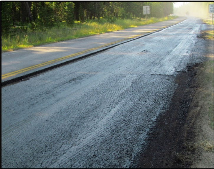
← Completed tack run.
