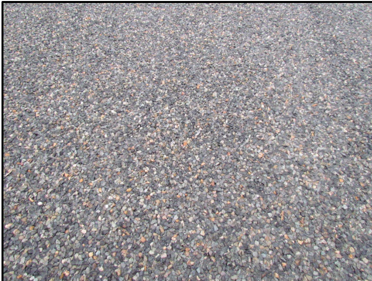
← Close-up of chip seal surface.
