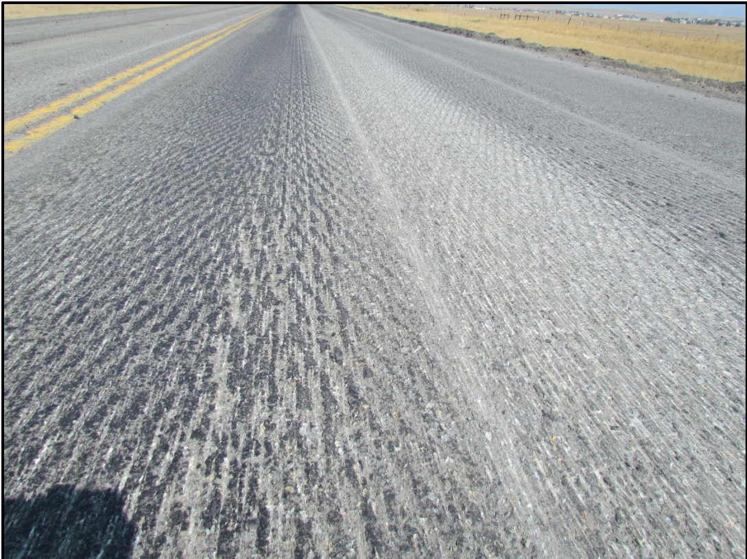
↑↓ Section of roadway with completed road smoothing.
