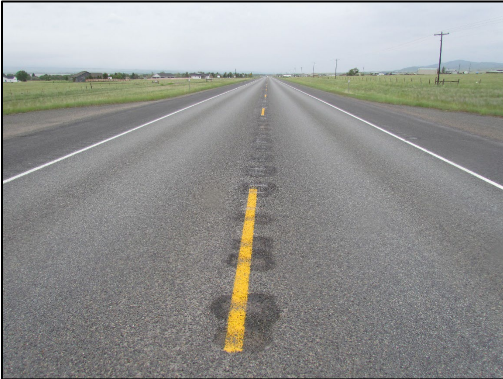
↑ RP 72.0, view south. This is in the non-road smoothed section. Wheel path wear is also seen in this section.
