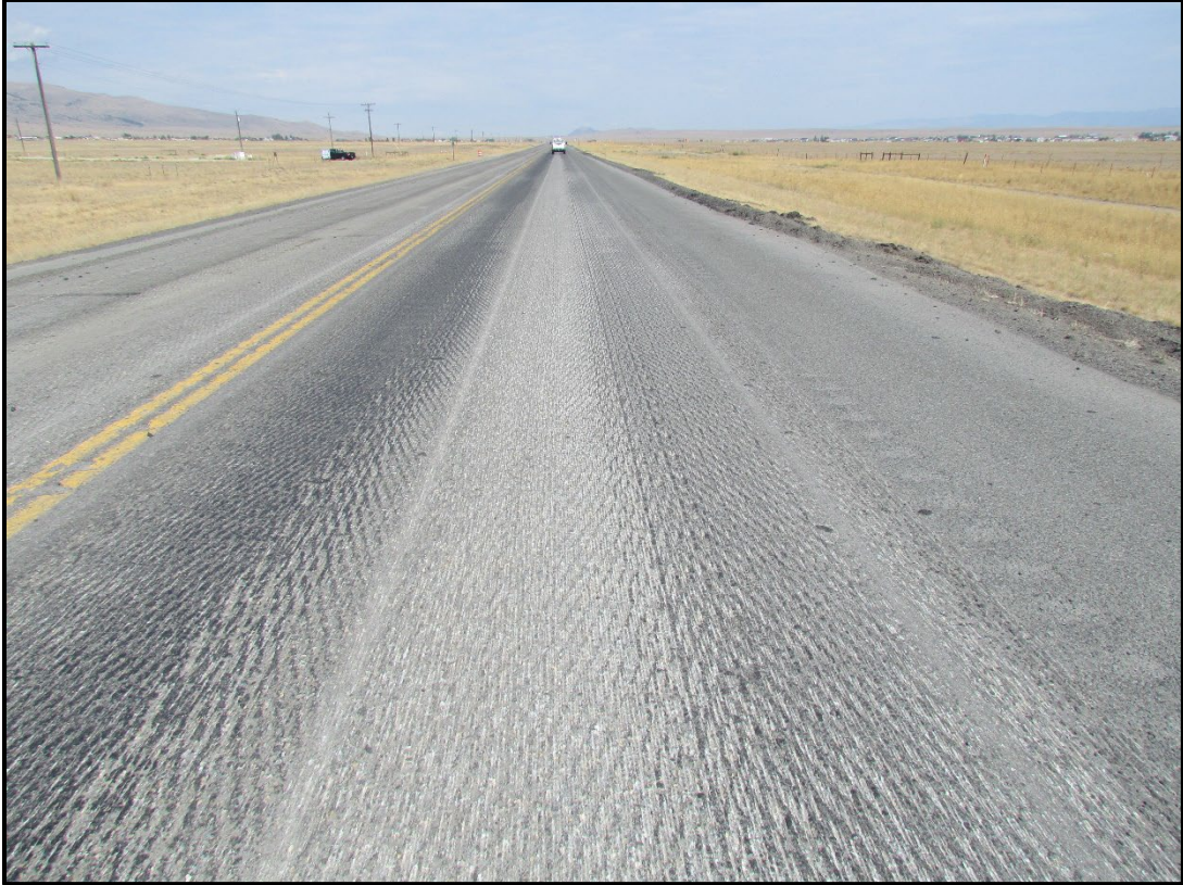
↑↓ Section of roadway with completed road smoothing.
