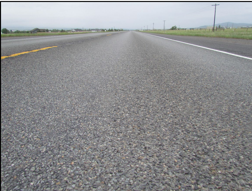
↑ RP 72.0, close-up view of the surface texture.
