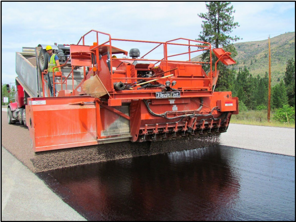
↑ Self-propelled chip spreader placing chips.
