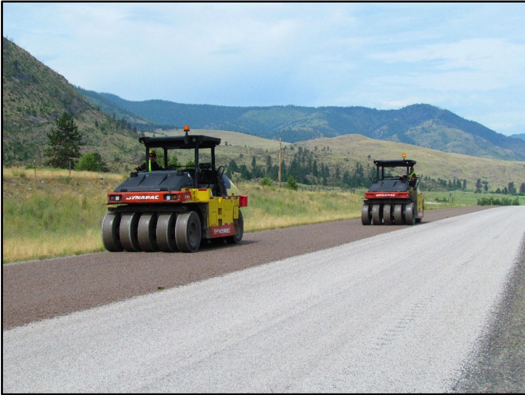
↑ Two nine-wheel pneumatic rollers were used to set the chips.
