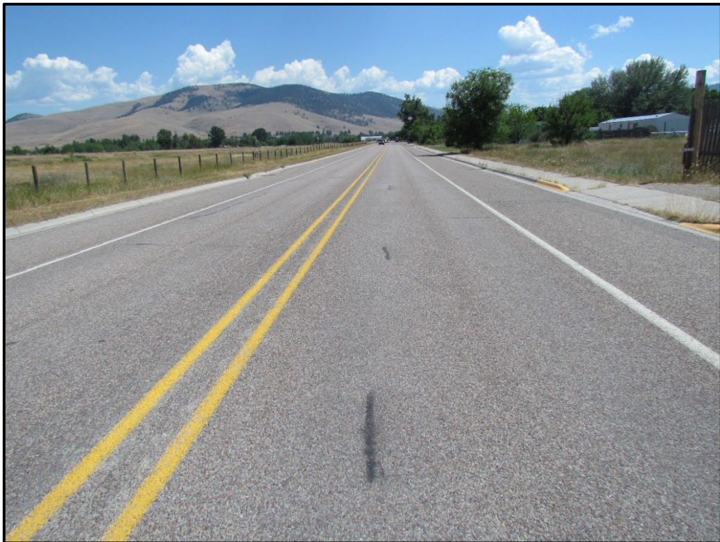
↑ RP 108.5, begin CHFRS-2P section, view east.
