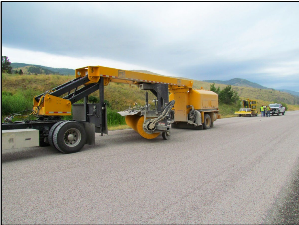
↑ Several sweepers were used to remove loose chips.
