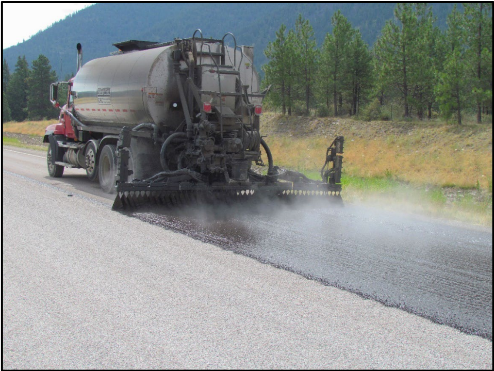
↑ Chip emulsion application.
