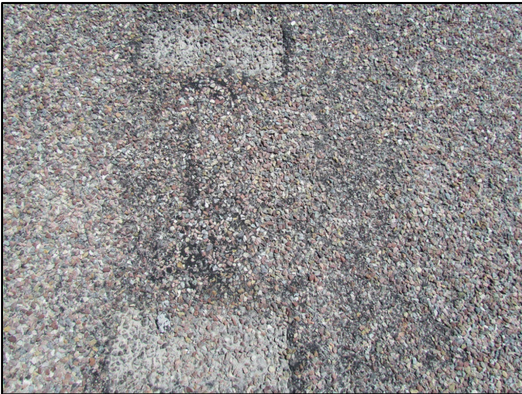
↑ RP 102.8, CRS-2P section, close-up view of the chip seal at the centerline.
