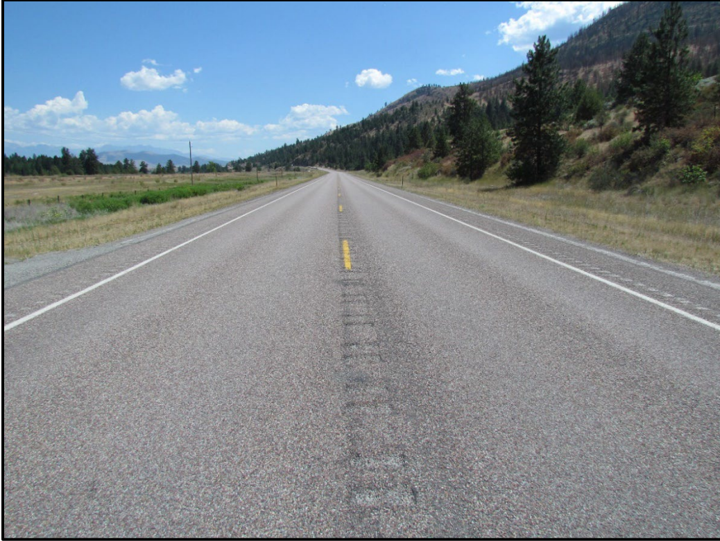
↑ RP 102.8, CRS-2P section, view east.
