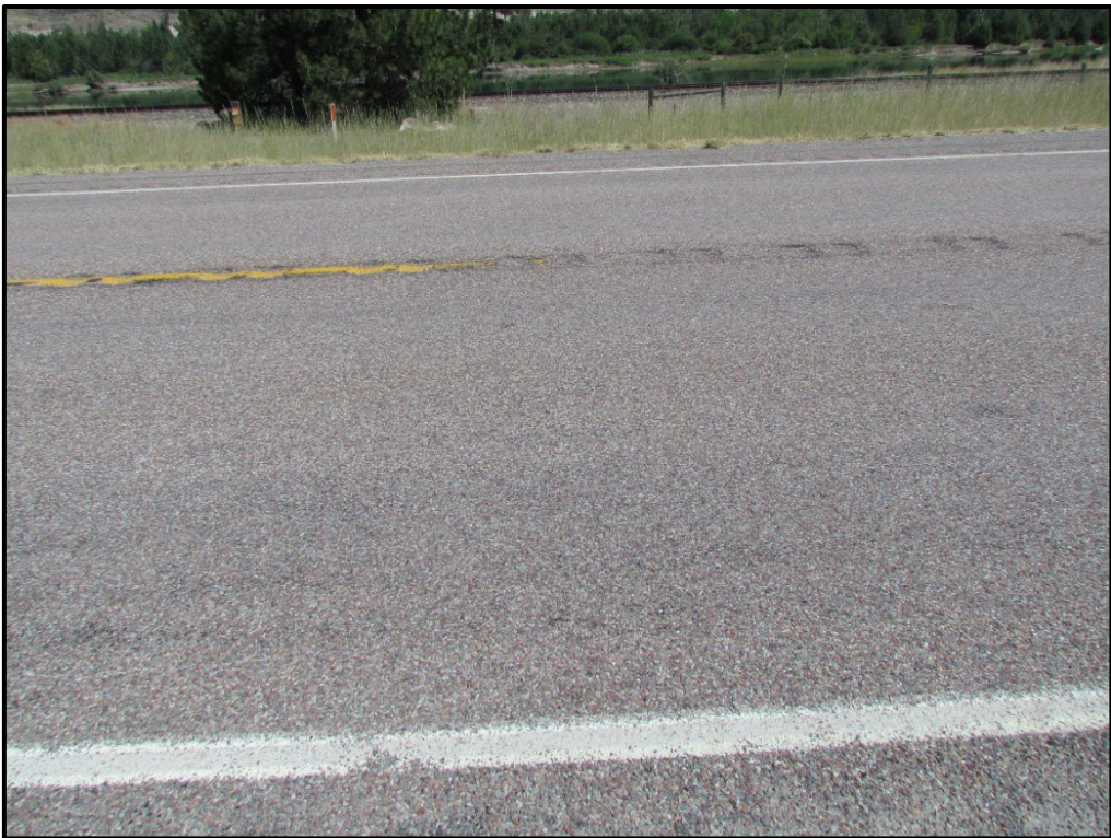
↑ RP 99, CRS-2P, transverse view.
