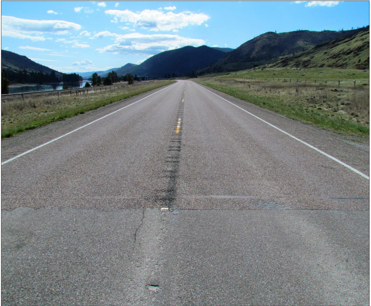
↑ Section CRS-2P : Approximate project length RP 98.7-108.5; Project start at west end on Primary HWY 200; view east.
