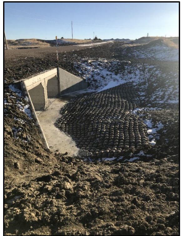
↑ Flexamat was also placed at the inlet and outlet of the box culverts.
