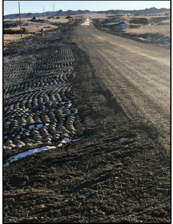
↑ Outlet side of roadway.
