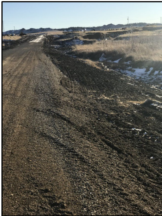
↑ Inlet side of roadway.
