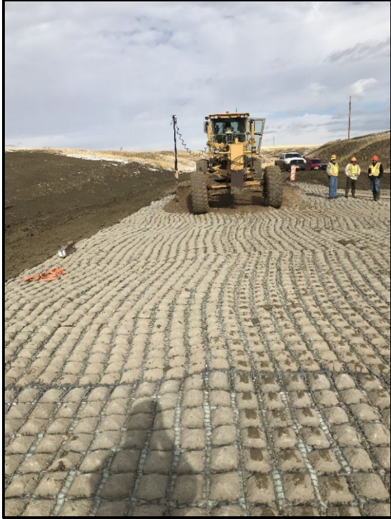
↑ Surfacing gravel being placed.
