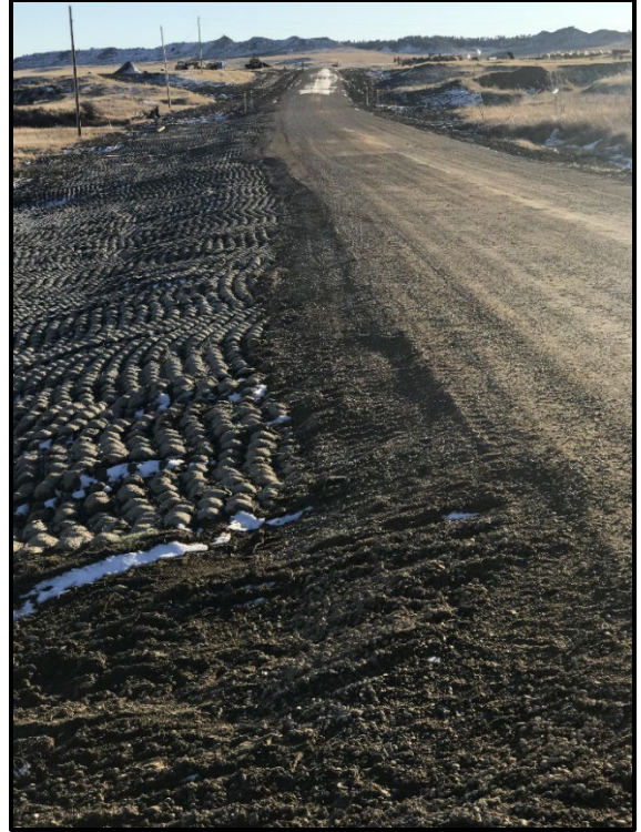
↑ Outlet side of roadway.
