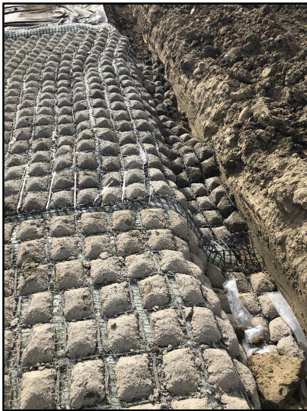
↑ View of how the Flexamat was anchored on the inlet side of the road.
