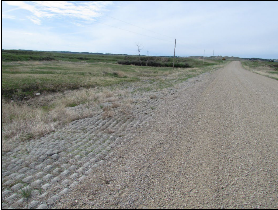
↑ Outlet ditch with Flexamat, view south.
