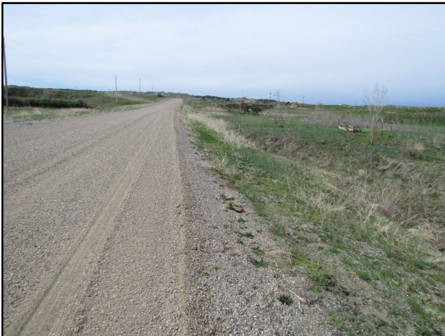
↑ Inlet ditch without the Flexamat, view south.
