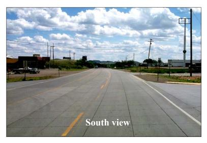
Highway 16 (P-20) suffered from rutting, plastic deformation and transverse cracking. The Montana Department of Transportation decided to construct a thin-whitetopping project based on minor rehabilitation criteria. Whitetopping is an alternative to the regular program of mill & fill. This procedure bonds a flexible layer to a rigid layer to form a bonded composite
