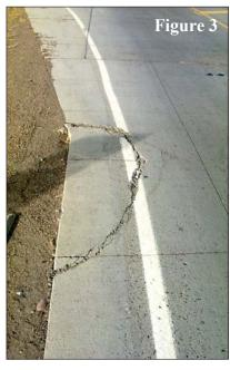
to the back and forth action of the unit) created the undulation or 'rough ride' as indicated. In addition, since the paver rested on the east edge of the previously placed southbound lane during construction, it most likely accelerated the roughness aspect of the ride for the northbound lane. Regardless of the ride analysis and the transverse cracking, which can be attributed to constructability issues, this project is performing well. The next evaluation will be held in the fall of 2005.
