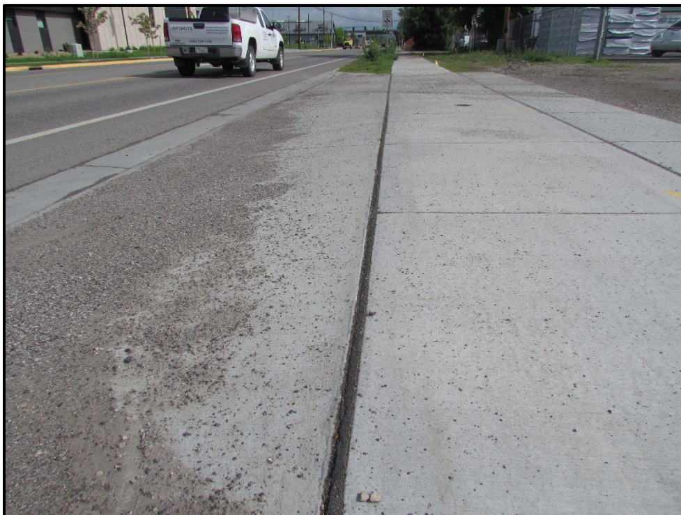
↑ An example section that was highlighted as a place where the Nomaflex worked well specifically because of the long length of the joint and the workability of the product.
