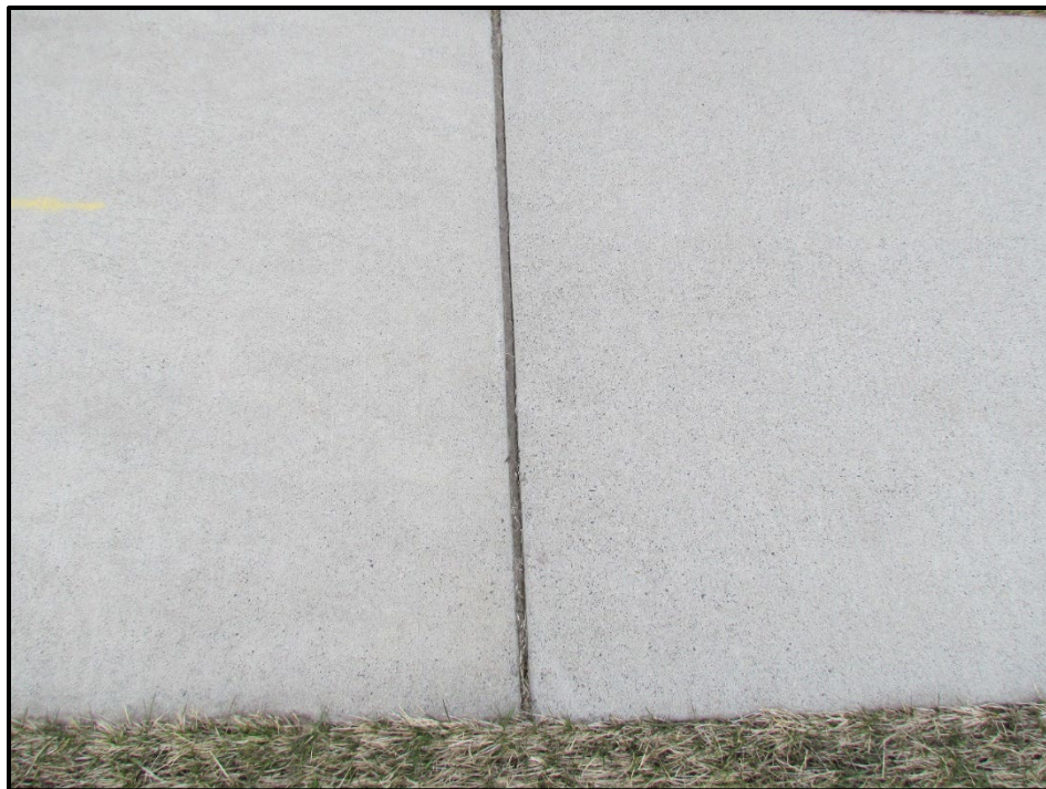
↑ Example of asphalt fiber joint filler that is considered a control from a section of existing sidewalk near but outside of the project limits that's typically used when constructing concrete expansion joints.
