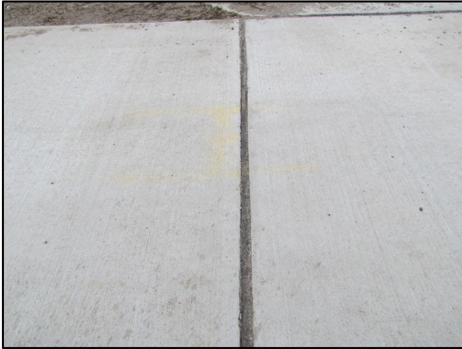
↑ Example of the Nomaflex used on the project. The photos for this visit are between Tamarack Street and Oak Street on the eastern sidewalk.
