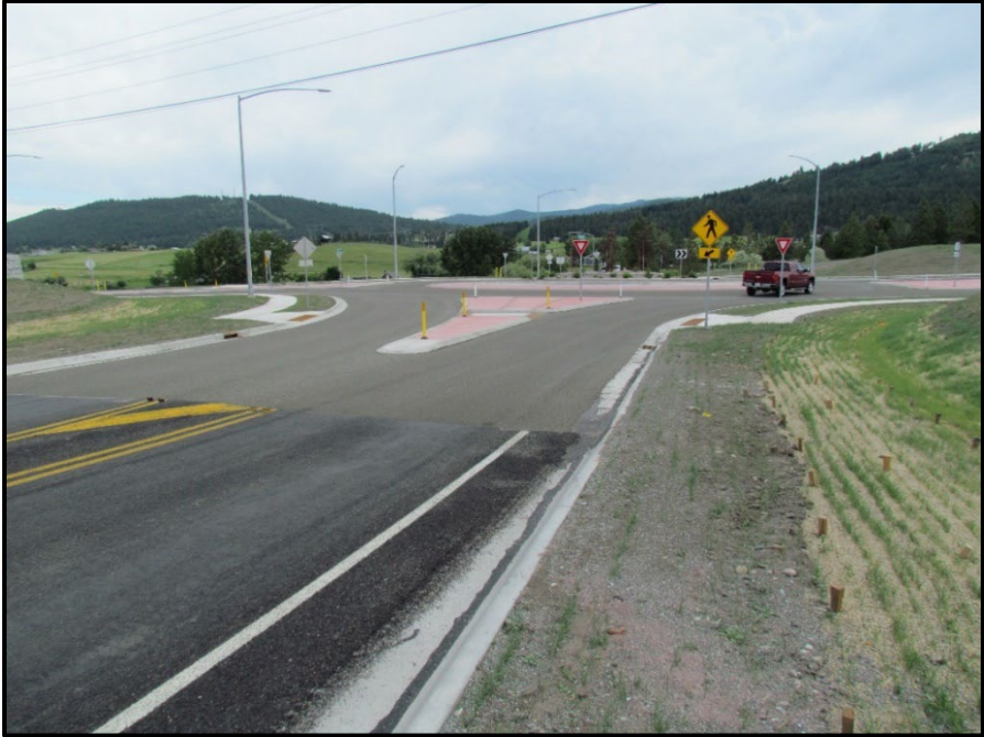
↑ View of roundabout from southbound lane of Spring Creek Road.
