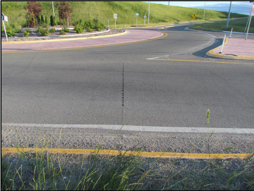
↑ View north of the main section of the roundabout.
