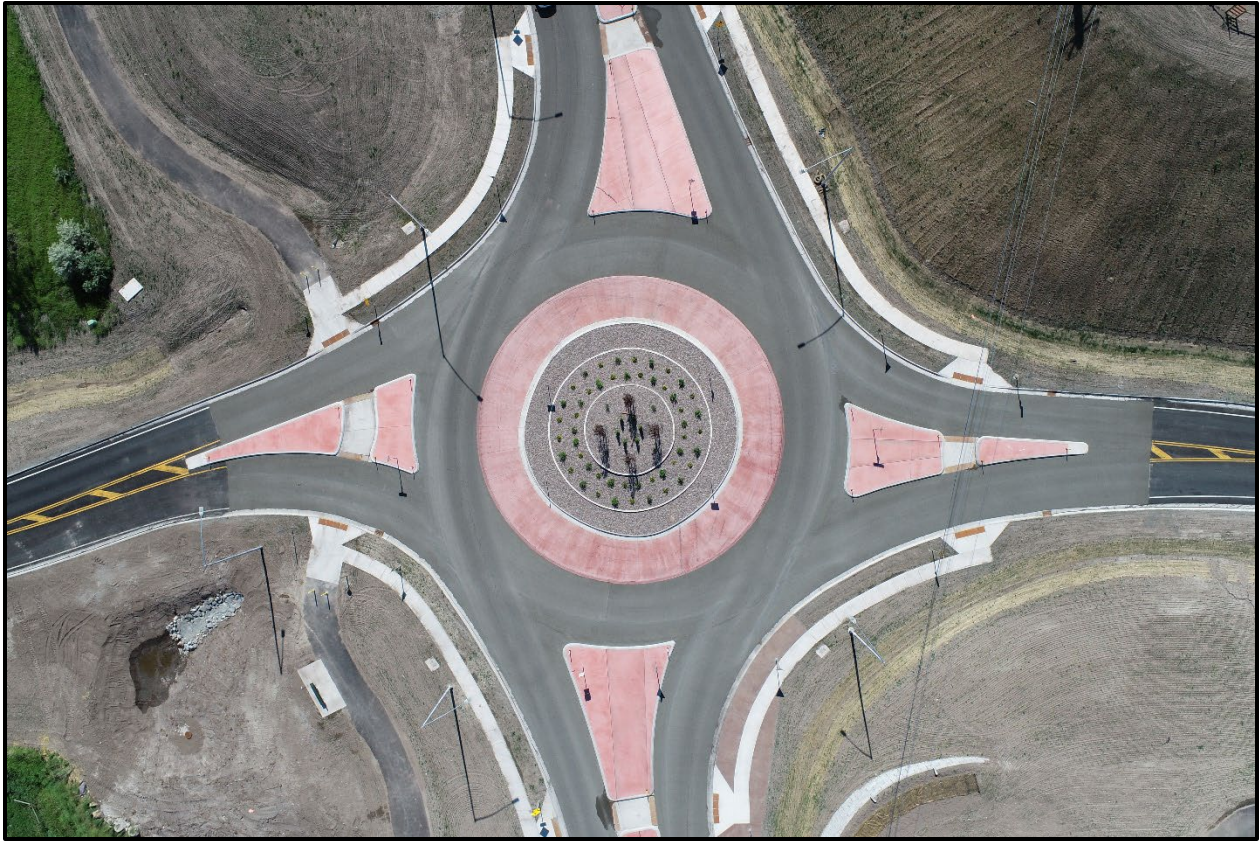
↑ Aerial photo of the completed polymer overlay on the PCCP roundabout.
