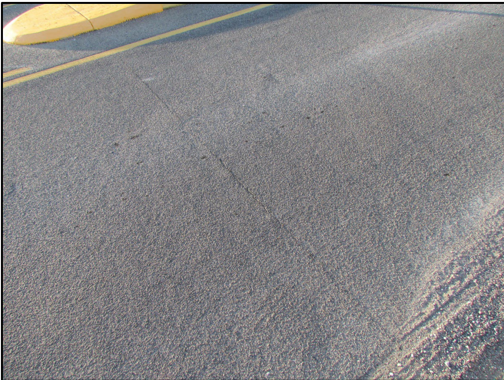
↑ Close up view of the surface and texture of the polymer overlay.
