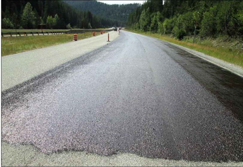
← Completed pass of FSCS emulsion.
