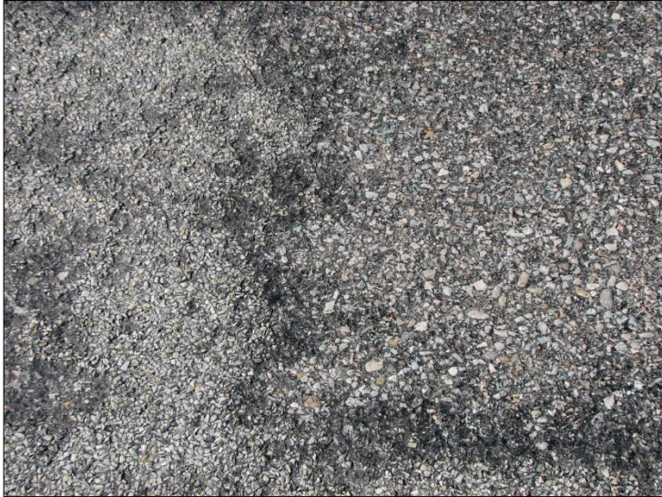
← Example section of FSCS removed to the level of exposed asphalt cement (AC).
