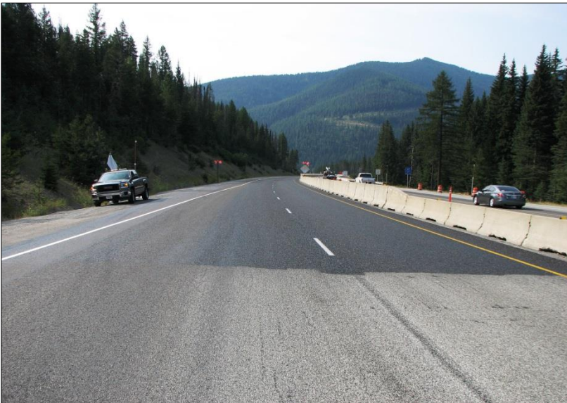
← Section of westbound FSCS at approximate reference point 0.0/Lookout Pass: View east.
