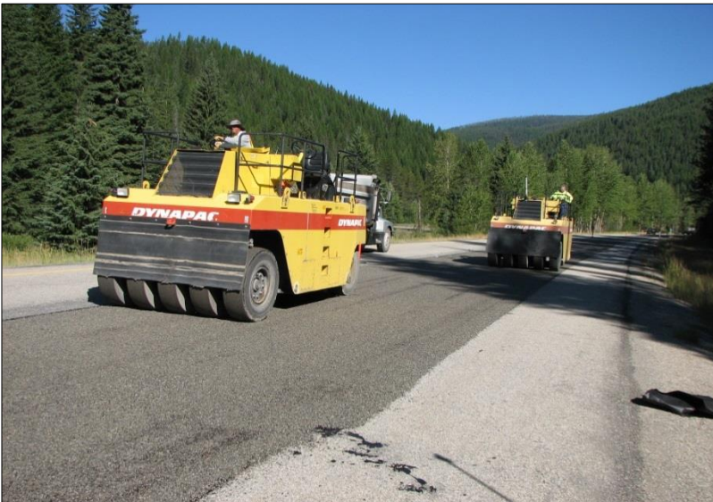
← Several nine tire pneumatic roller are used in the compaction phase.
