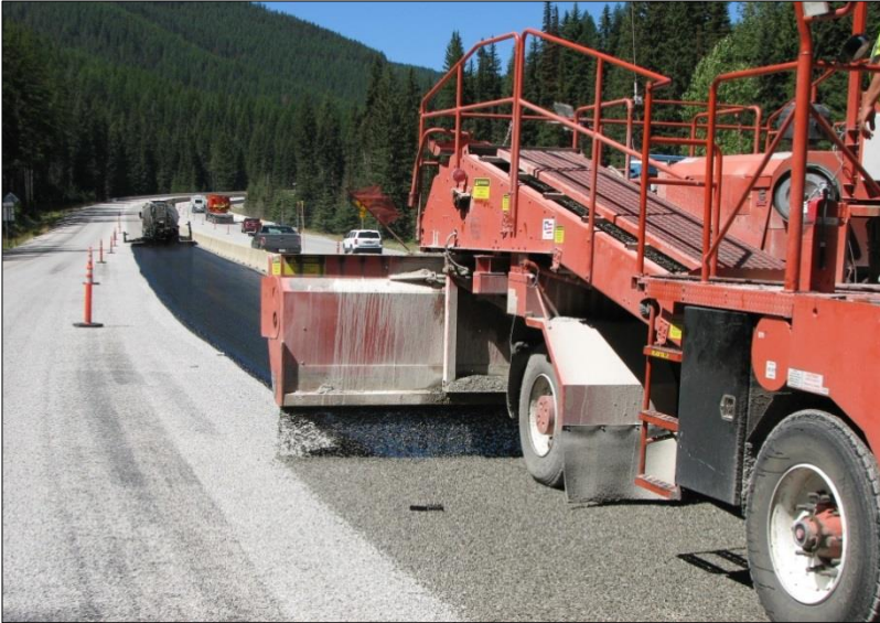
← Representative image of chip spreader applying the specified Type 2 cover material.
