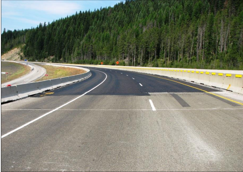
← Section of eastbound FSCS at approximate reference point 5.7/Taft Area Interchange: View west.
