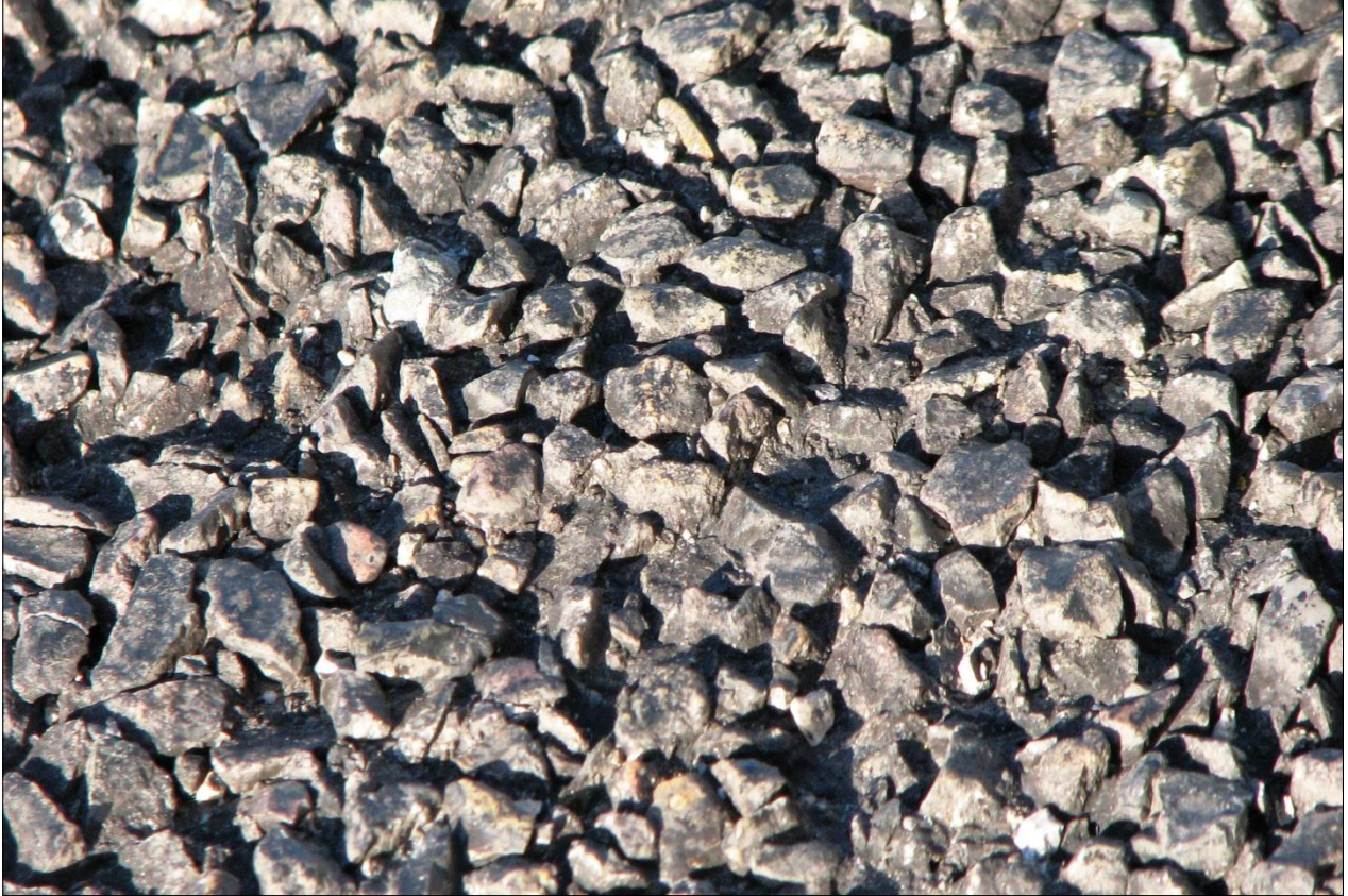
↑ Close-up of chipped surface of Test Section 1.
