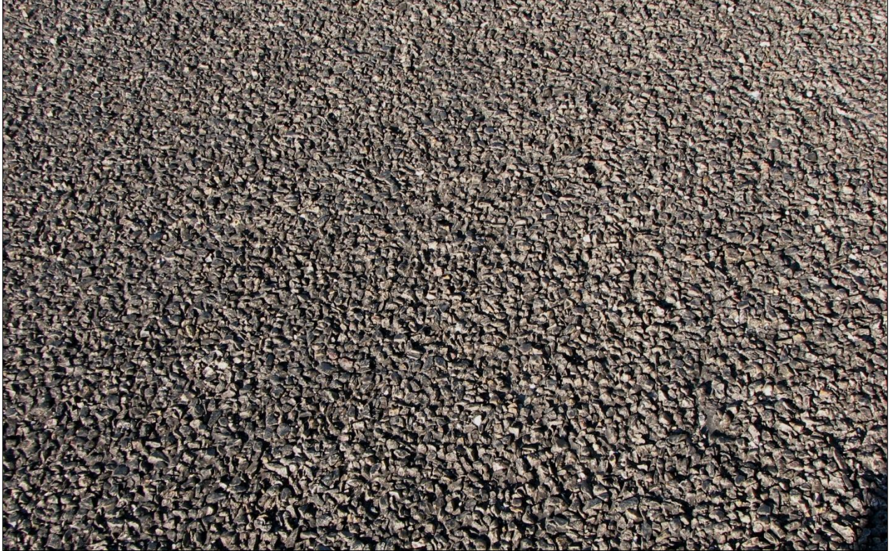
↑ Closer view of pavement texture of Test Section 1.
