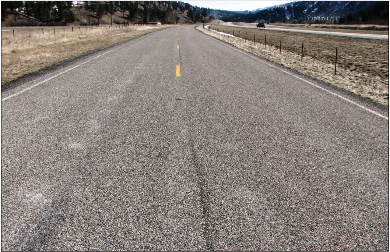
↑ Control Section: Conventional Chip Seal – Mile point 3 looking east.
