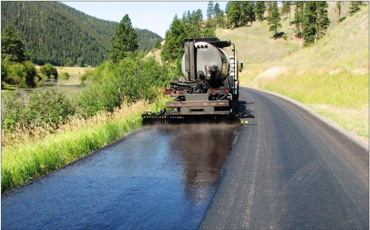
↑ Application of AC emulsion at approximately 150°F (66°C).
