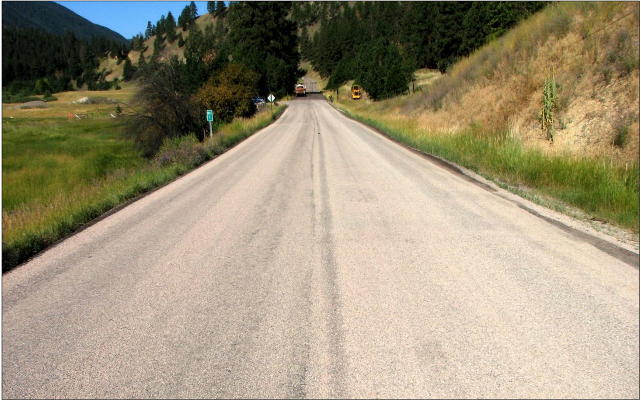
↑ Completed chip seal.
