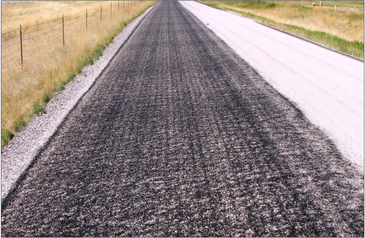
↑↓ Images of the Test Section 2 application, (SS1 .05 gallon per sq. yd.). Both views looking west.
