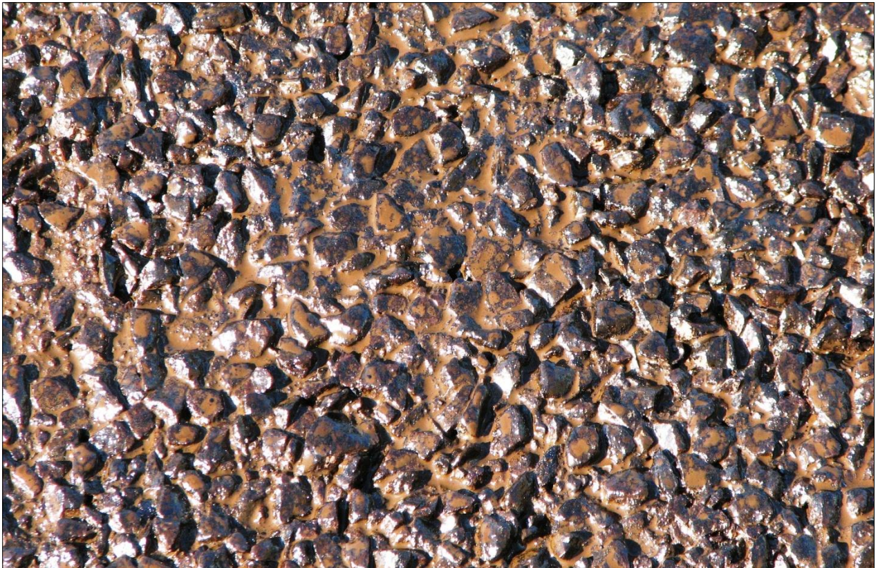
↕ Several close-up images of the Section 1, SS1 application directly after placement.
