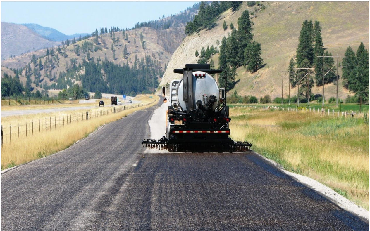
↑↓ Images of the Test Section 2 application, (SS1 .05 gallon per sq. yd.). Both views looking west.
