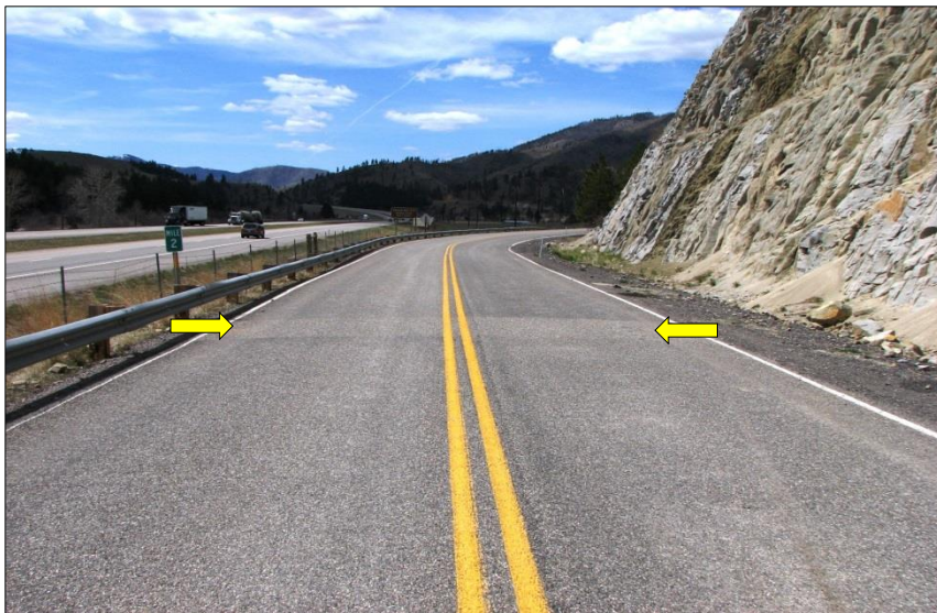
← Transition of TS2 and TS1 at mile post 2; view west.
