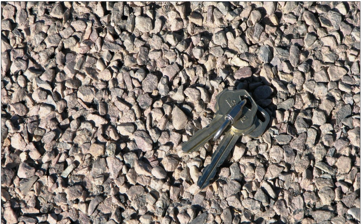
↓ Close-up of pavement surface.
