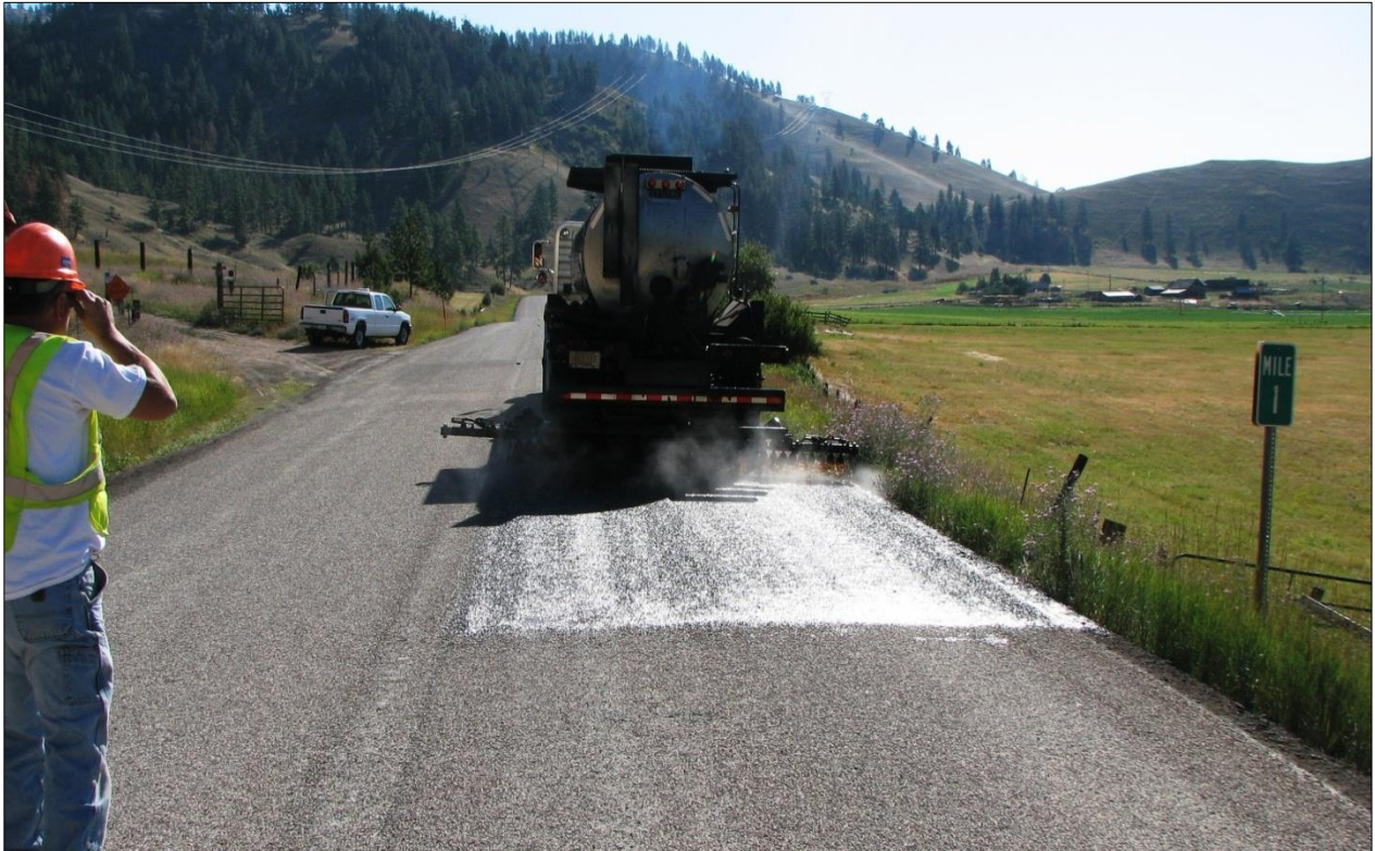
↑ Beginning of the Test Section 1 run of the SS1 at .1 gallon per sq. yd. concentration.
