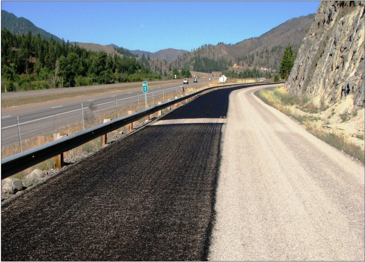
↑ View of the Test Sections 1 & 2 transition at mile marker 2, view west.
