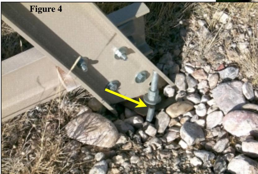
broken sill support has, up to this time, not caused a catastrophic failure of TS1. Nor is there any evidence that this loose rear sill attachment may have caused stress that allowed the center clip bracket to shear off. It was also observed the right front frame to bolt attachment has bent slightly. This may be the result of the freedom of the rear connection, which is allowing the stress from wind turbulence to deflect the bolt. The sill frame will be closely monitored in future
