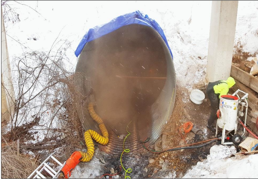
← ↓ The base of the culvert where active corrosion took place is sand blasted (Kleen Blast Abrasives) to bare metal and vacuumed clean.
