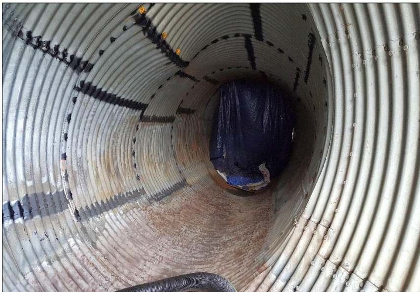
← Completed sand blasting.
