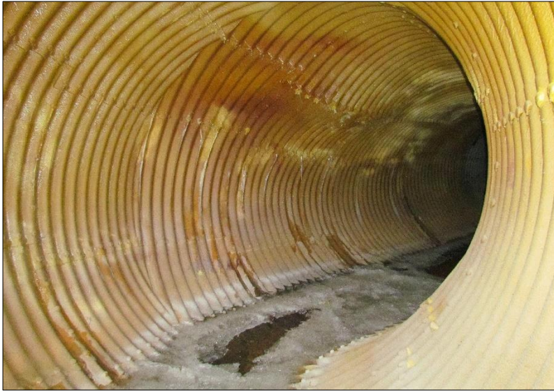
← Overview of culvert inlet.
