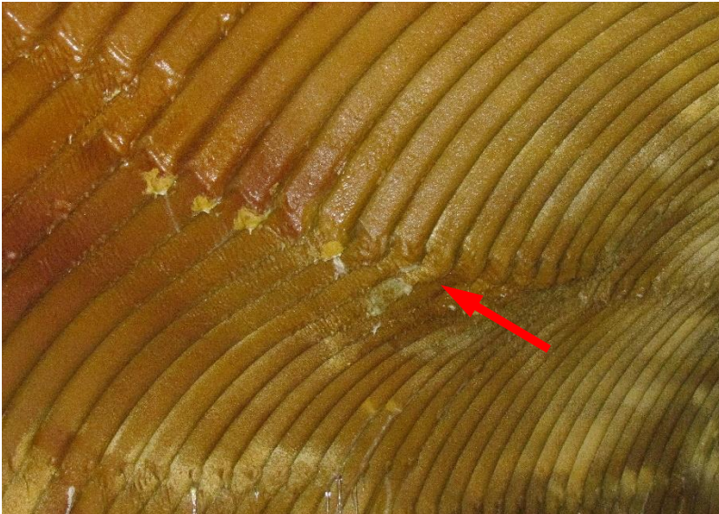
← Area of culvert deflection.
