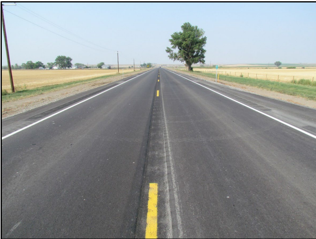
↑ RP 6.0, Sta 255+37, view west. Completed plant mix surfacing.
