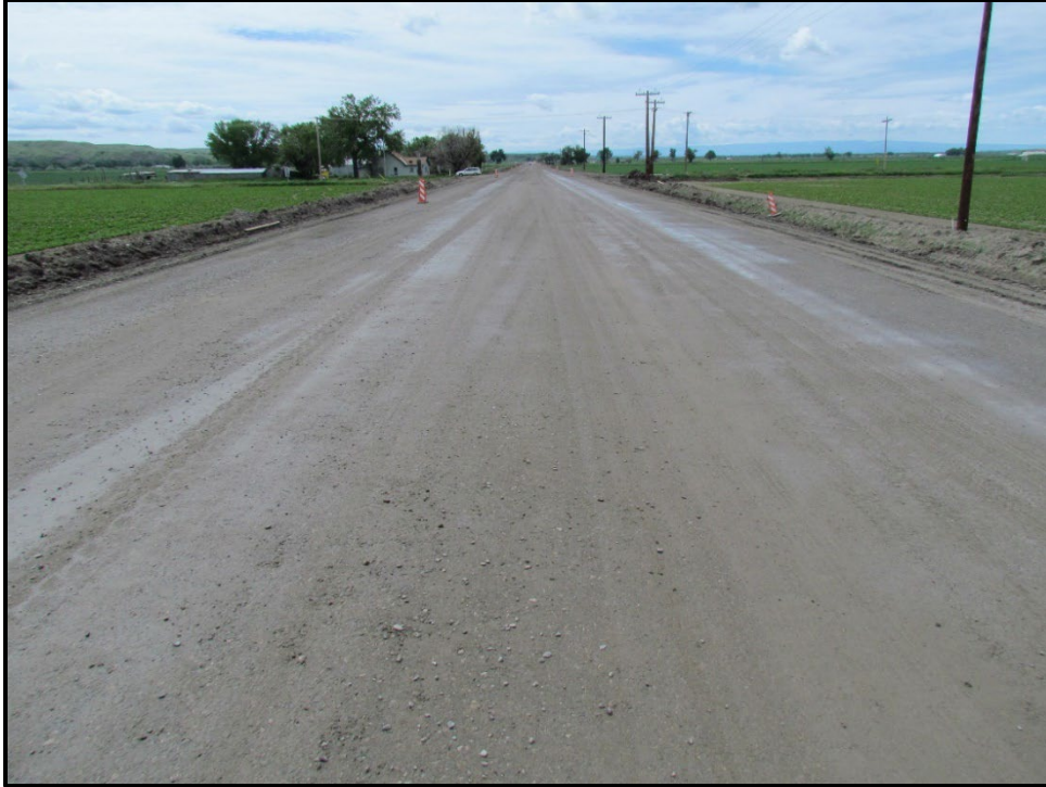
↑ Completed CAC surfacing after compaction. Approximately station 92+00, view south.
