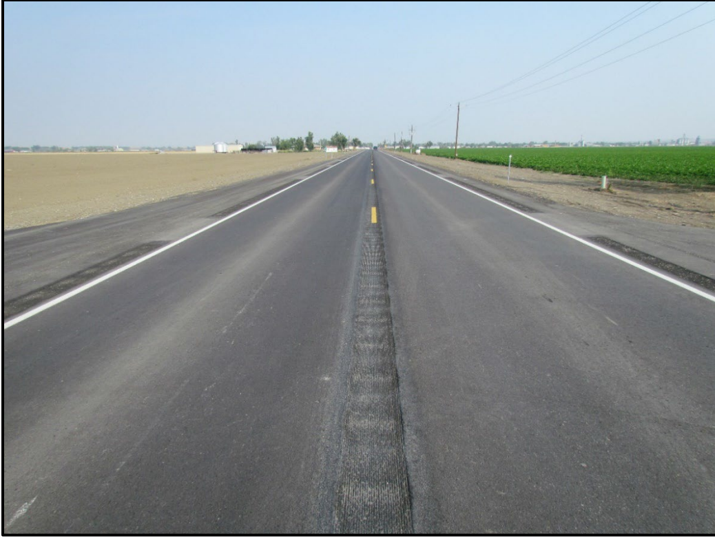
↑ RP 2.0, Sta 44+17, view north. Completed plant mix surfacing.
