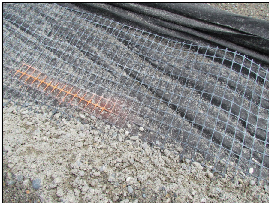
↑ Close up view of the grid. There was slight waviness in the product but was being mitigated as well as possible. MDT inspectors stated it might have helped to require anchors for the grid but upon reviewing the product information from the supplier, when using anchors, the waviness issues were harder to eliminate.
