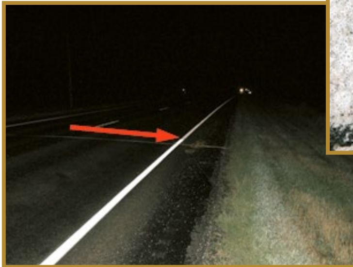
Red Arrow Notes Delineation of 3M Ceramic Elements Beads Vs. Conventional Beads
