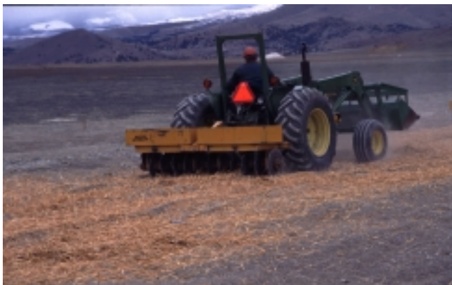
Crimped straw can be used alone or in conjunction with temporary seeding to help stabilize soils (BMP SS-6).
