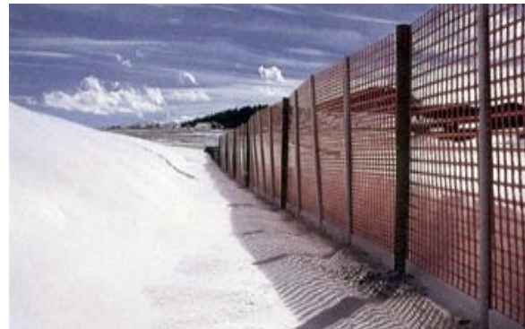
Fence can be used to limit snow accumulation in selected areas (BMP SN-2).
