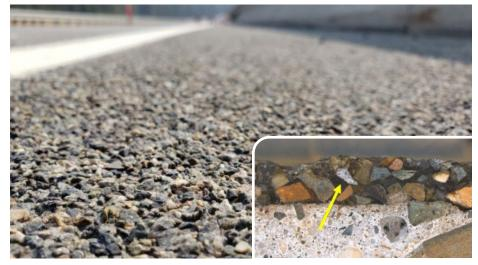
Polymer overlays with high friction materials can extend the life of a bridge and provide skid resistance.
