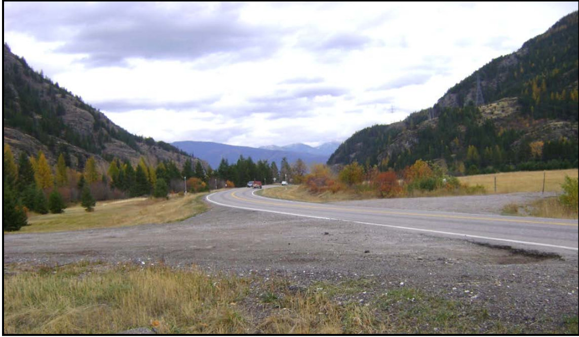
Photo 1. Looking east on the north side of US 2 at a recreational access point. RP 140.1 (Sta. 20).
