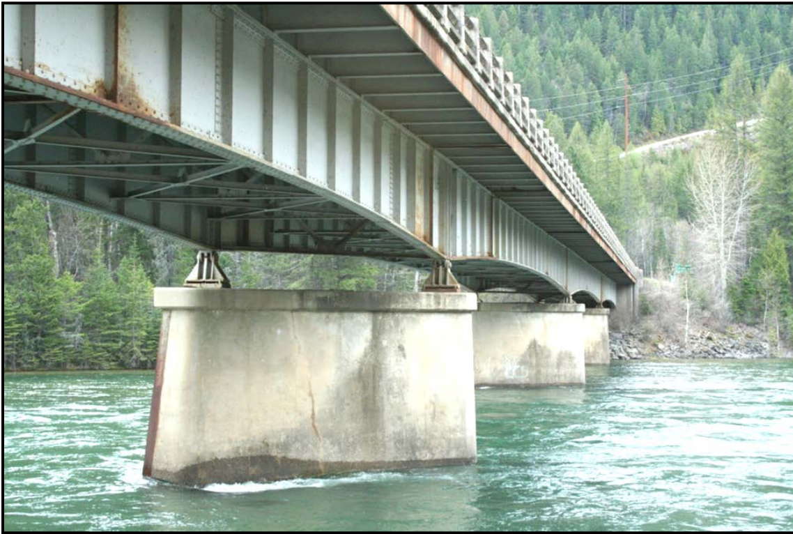
Photo 41. Looking east under the bridge over the South Fork of the Flathead River that is showing signs of corrosion. RP 142.1 (Sta. 129).
