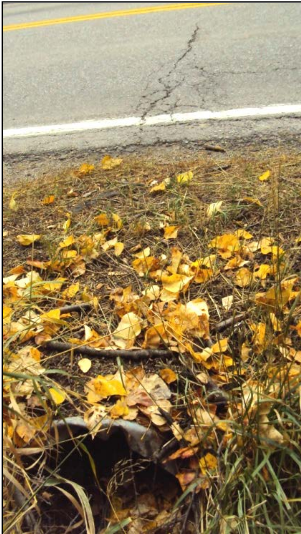
Photo 29. Single 18-inch CMP (approximately sixty percent buried) with minimal cover beneath roadbed on the south side of US 2. RP 141.3 (Sta. 73).
