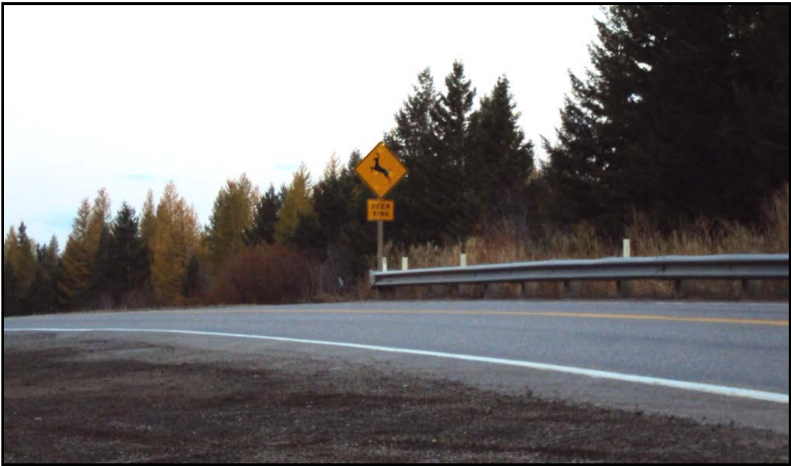
Photo 6. Wildlife crossing sign located on north side of US 2. RP 140.3 (Sta. 29).
