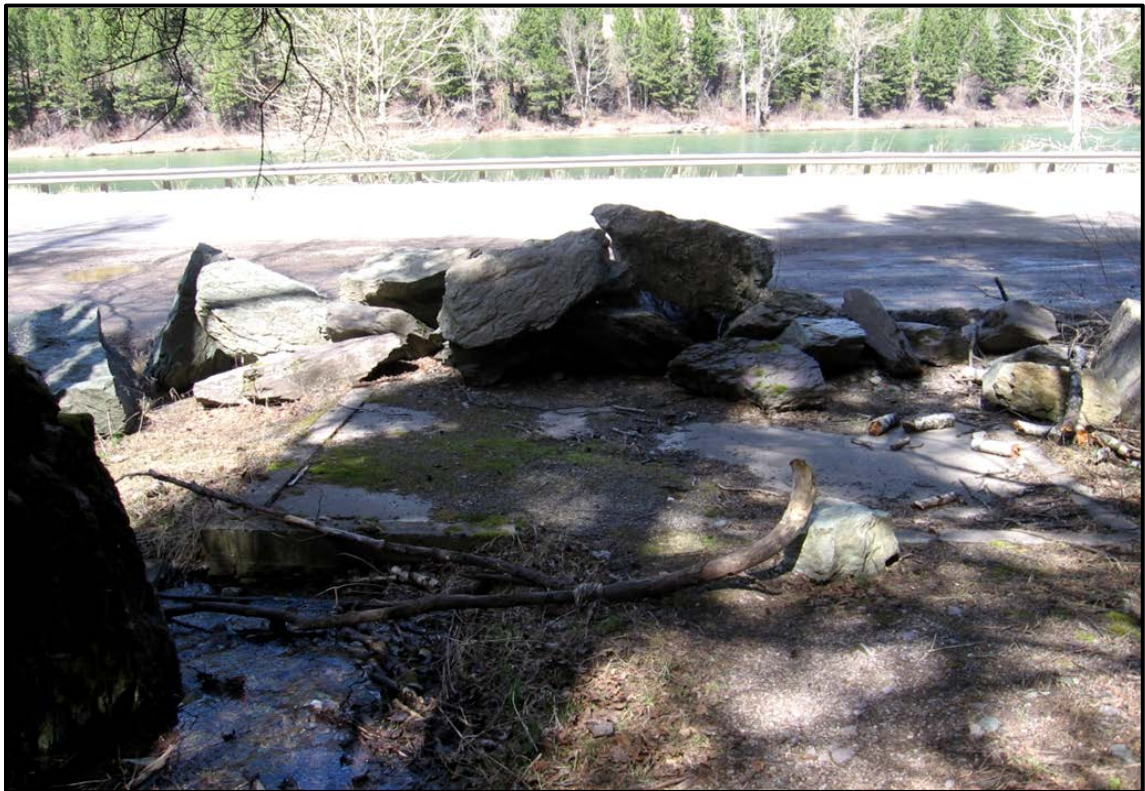
Photo 16. Looking north on the south side of US 2 at foundation for former rest area. RP 140.7 (Sta. 54).
