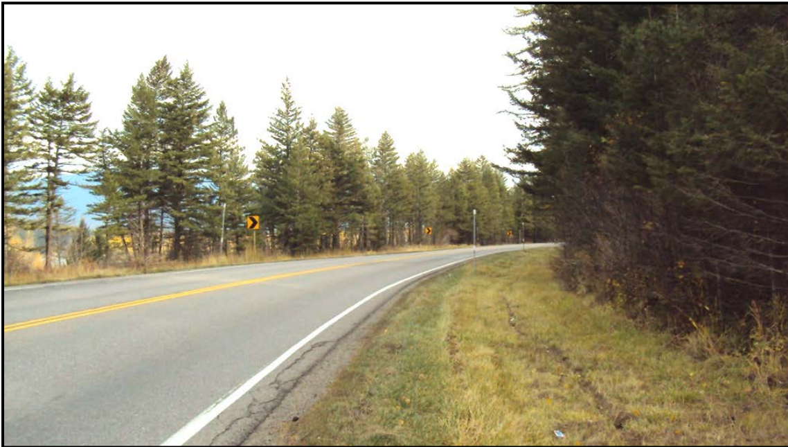
Photo 32. Horizontal curve and extended snow reflectors. RP 141.3 (Sta. 77).
