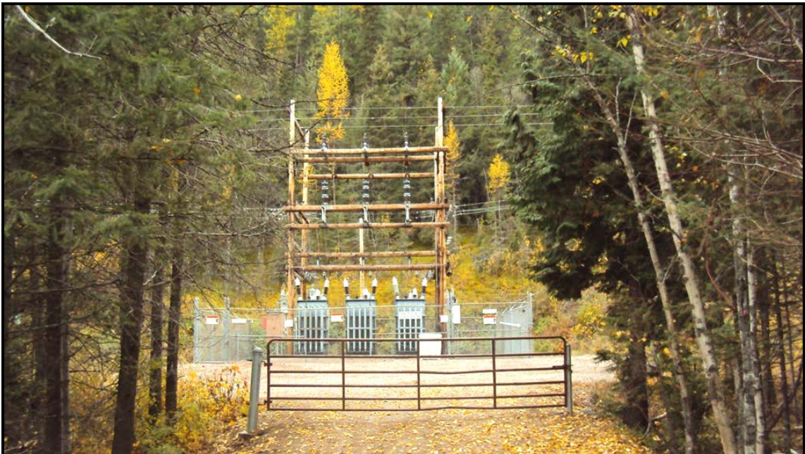
Photo 39. Substation located on south side of US 2. RP 141.8 (Sta.117).
