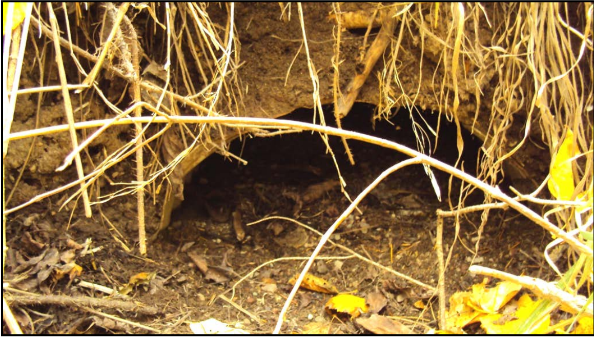
Photo 28. Single 18-inch CMP (approximately sixty percent buried) on the north side of US 2. RP 141.3 (Sta. 73).
