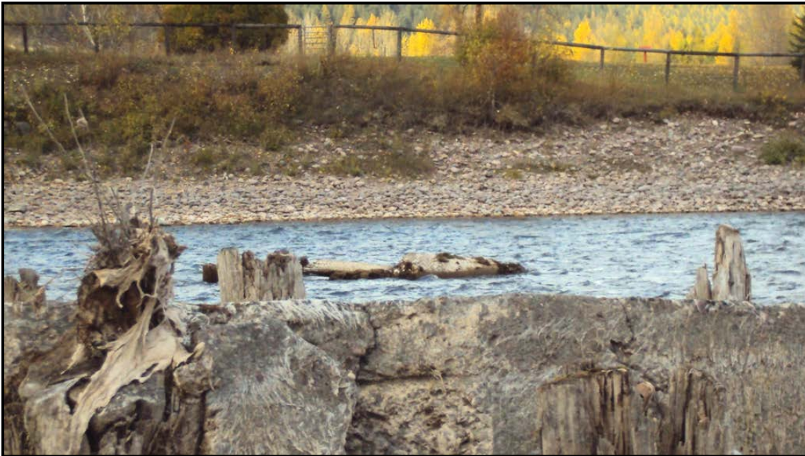
Photo 36. Looking north at a former bridge crossing. The concrete foundation of the former bridge can be seen. RP 141.7 (Sta. 111).
