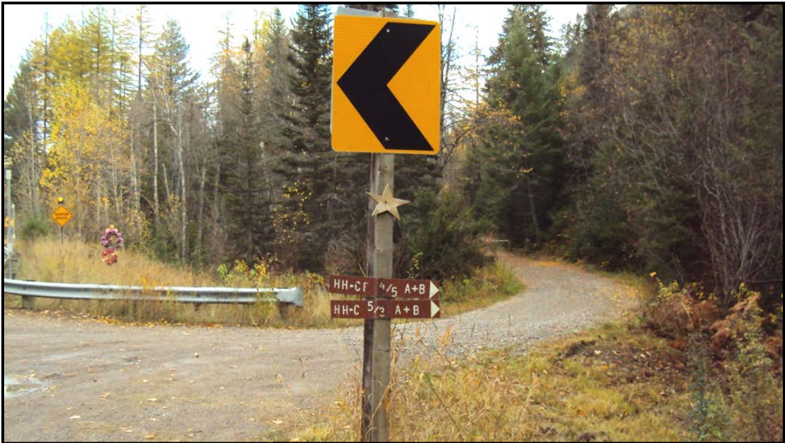
Photo 38. Looking south west on the south side of US 2 at a utility access road. RP 141.8 (Sta. 114).
