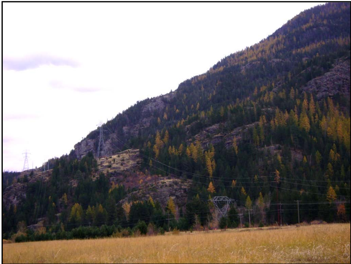
Photo 5. Power lines parallel US 2 to the south atop the rock outcroppings over the entire corridor. RP 140.1 (Sta. 20).
