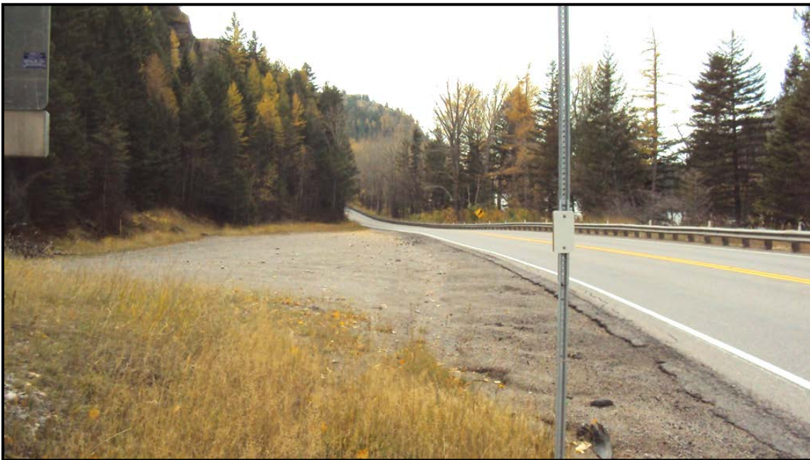
Photo 31. Roadside drainage issues along south side of US 2 looking west at the east pullout. RP 141.3 (Sta. 75).
