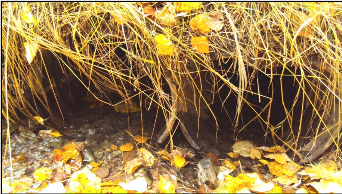
Photo 17. Two 18-inch CMP culverts south of US 2. RP 140.8 (Sta. 55).
