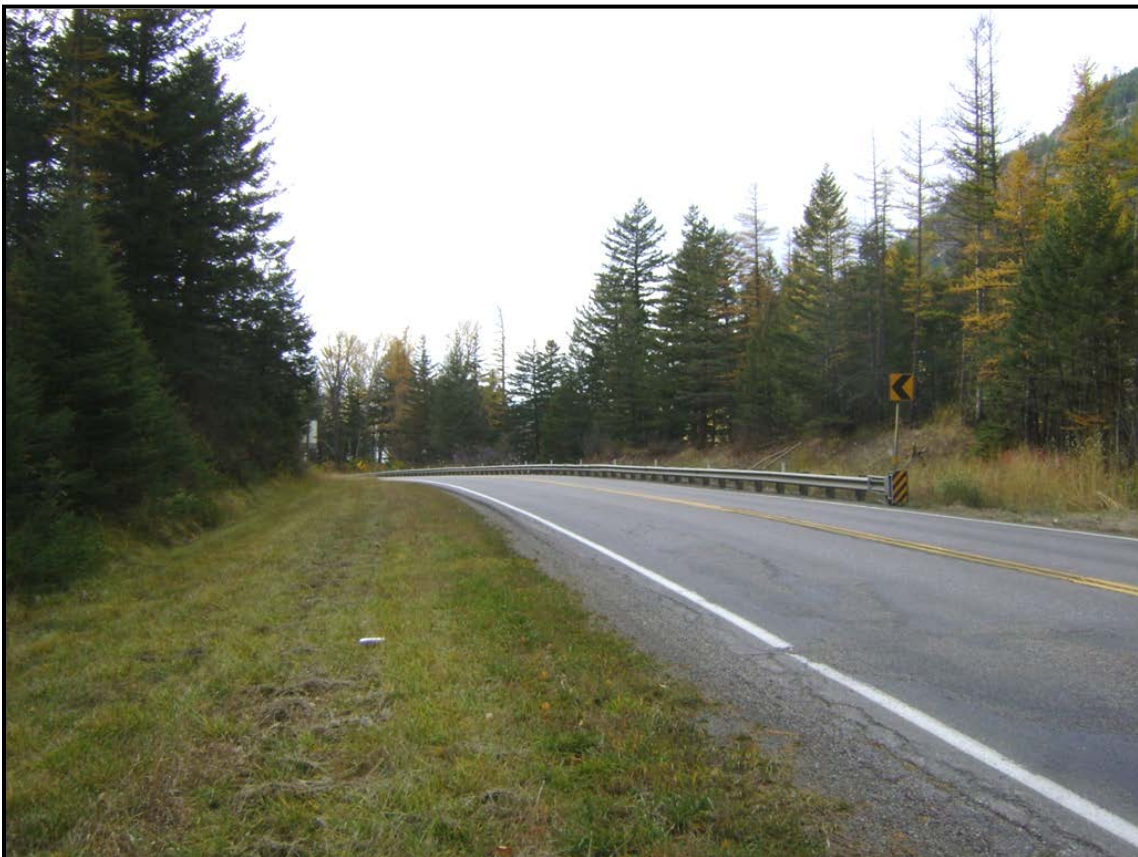
Photo 33. Looking west on the south side of US 2 at a horizontal and vertical curve. RP 141.3 (Sta. 82).
