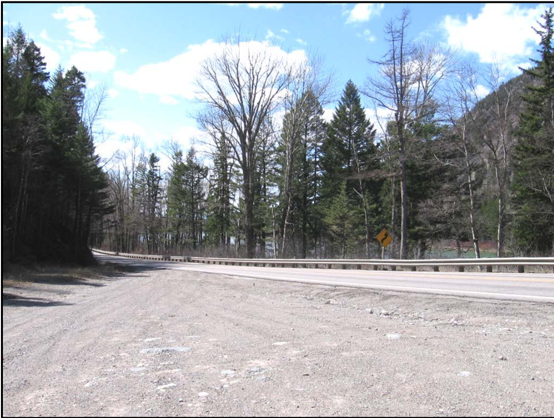
Photo 30. Looking northwest on the south side of US 2 at the east pullout. Roadside drainage issues are visible alongside the south side of the road. RP 141.3 (Sta. 75).
