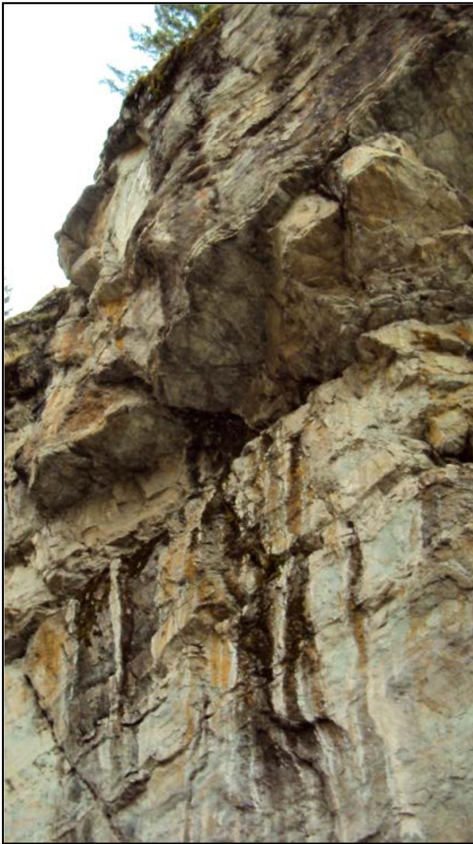
Photo 25. Evidence of water flow at east outcropping on the south side of US 2. Potential for falling rock. RP 141.1 (Sta. 67).
