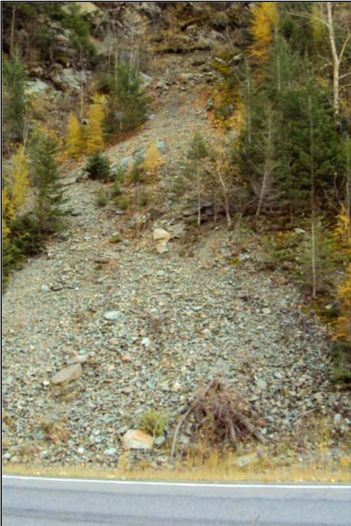
Photo 8. Unstable geologic features south of US 2. Potential for falling rock. RP 140.6 (Sta. 47).
