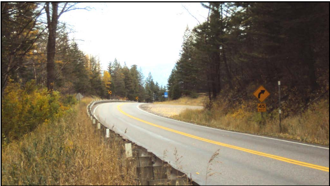
Photo 27. Looking east at a horizontal and vertical curve and a 45 mph warning sign. RP 141.2 (Sta. 70).
