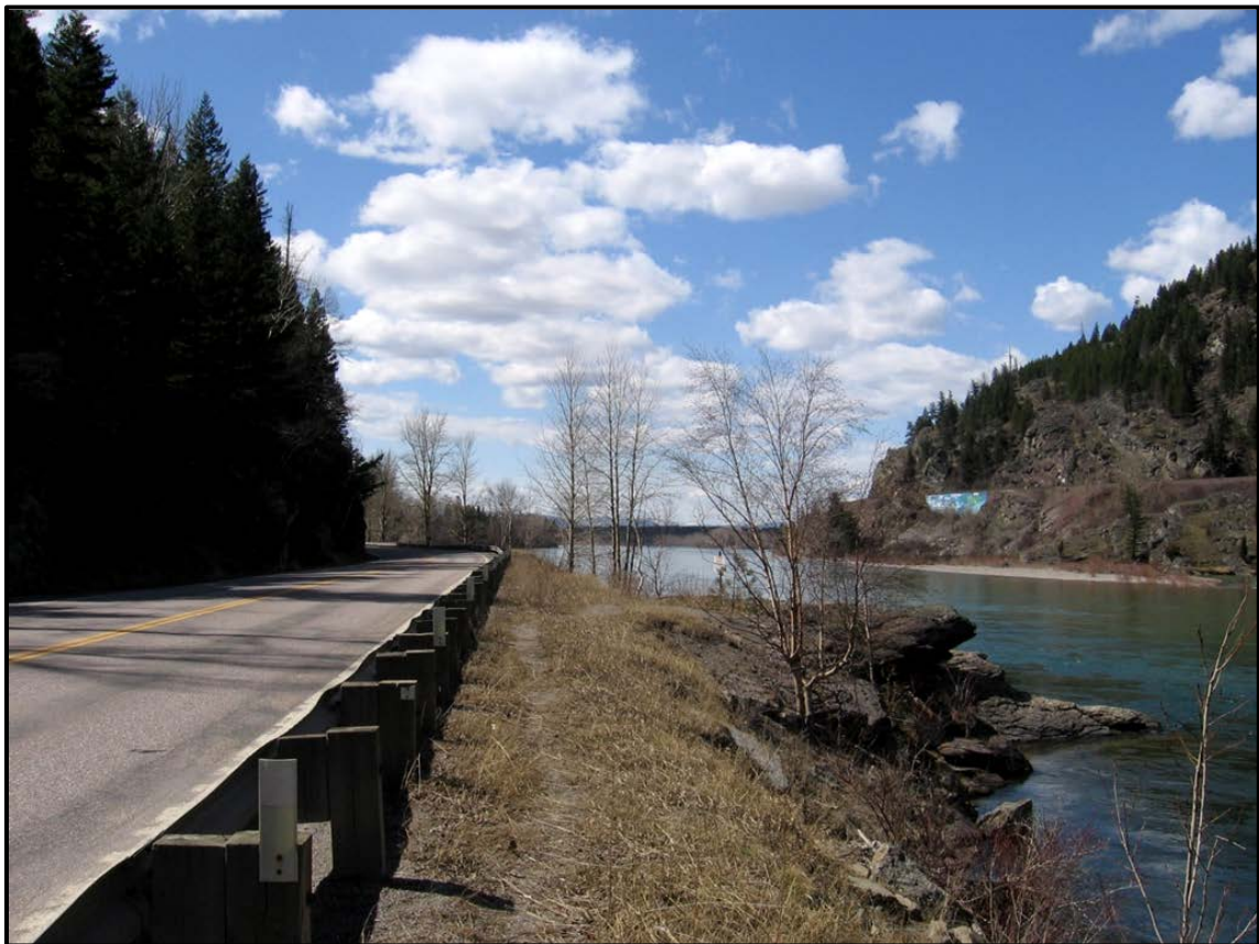
Photo 14. Looking west on the north side of US 2 at Fisherman's rock. RP 140.7 (Sta. 54).
