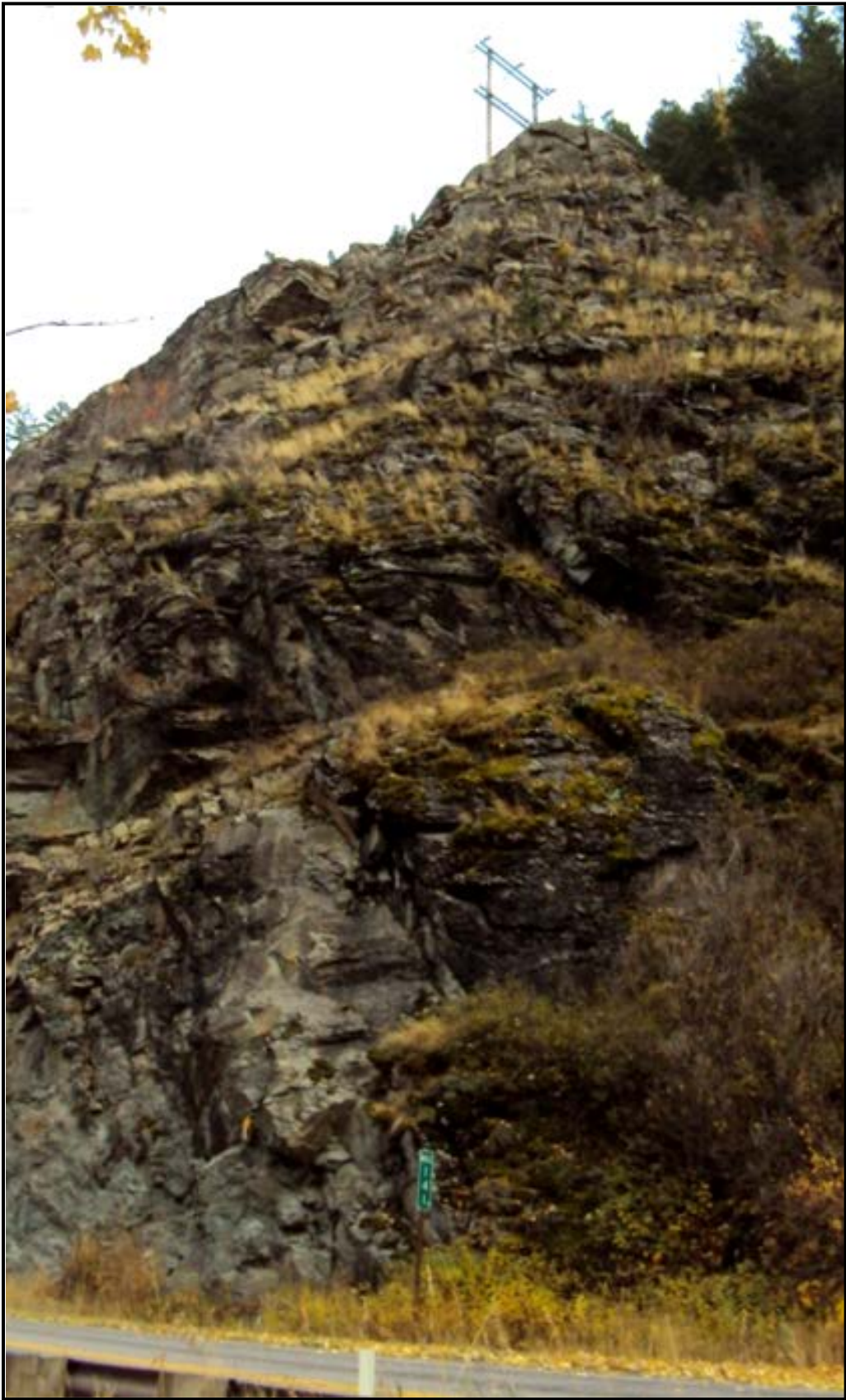
Photo 24. Reference Post 141 marker, power lines overhead, and east outcropping. Potential for falling rock. RP 141.0 (Sta. 65).
