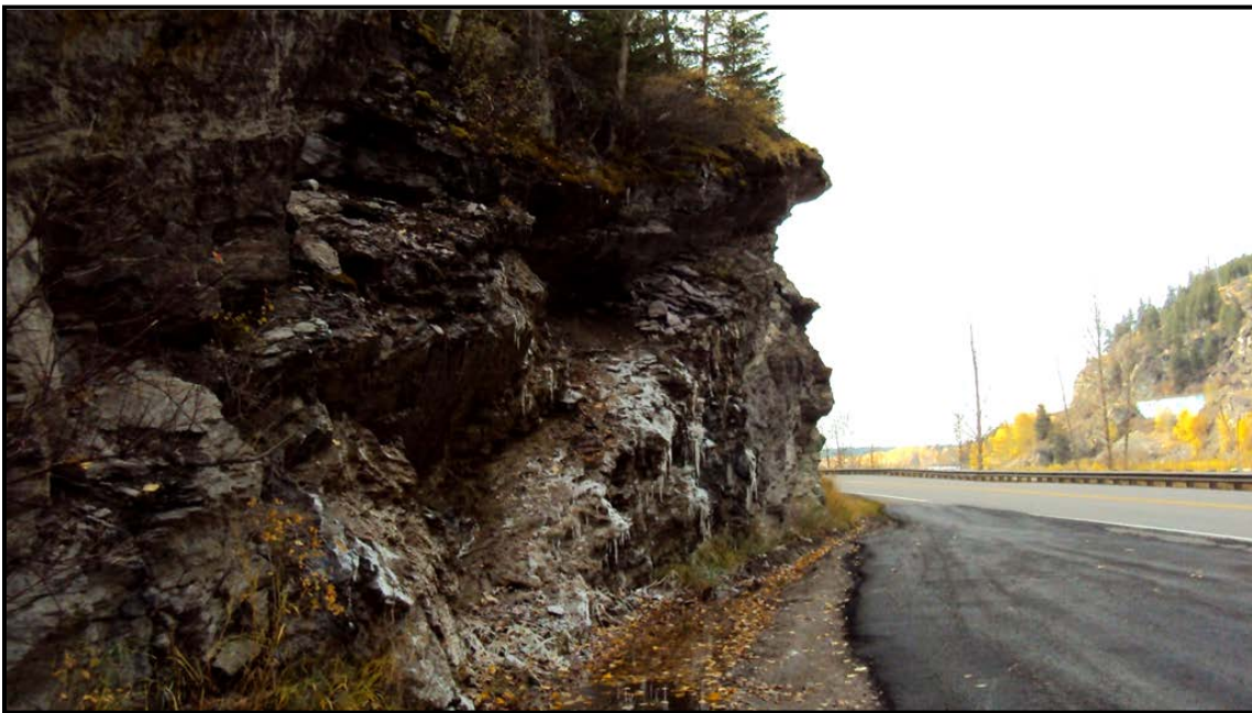
Photo 12. Icing on west outcropping on south side of US 2. RP 140.7 (Sta. 50).
