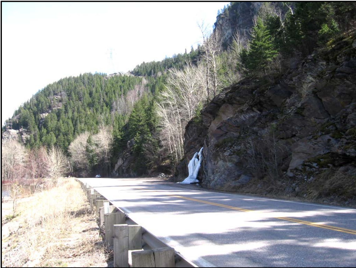
Photo 9. Looking east on the north side of US 2. Snow and ice on outcroppings to the south of US 2 may cause drainage issues. RP 140.6 (Sta. 47).
