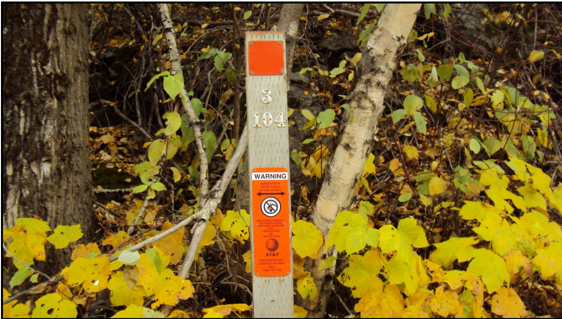
Photo 21. Fiber optic marker at east pullout. RP 140.9 (Sta. 57).
