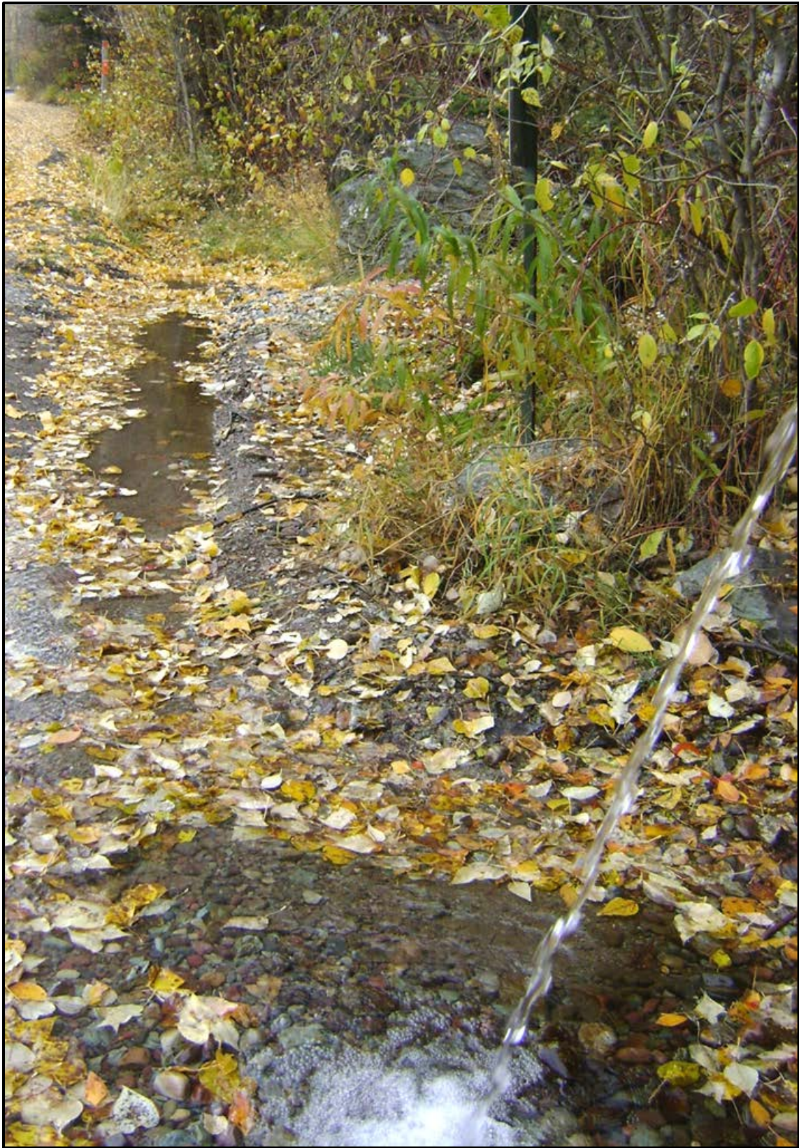
Photo 19. Drainage issues associated with Berne Memorial Park spring. RP 140.8 (Sta. 56).
