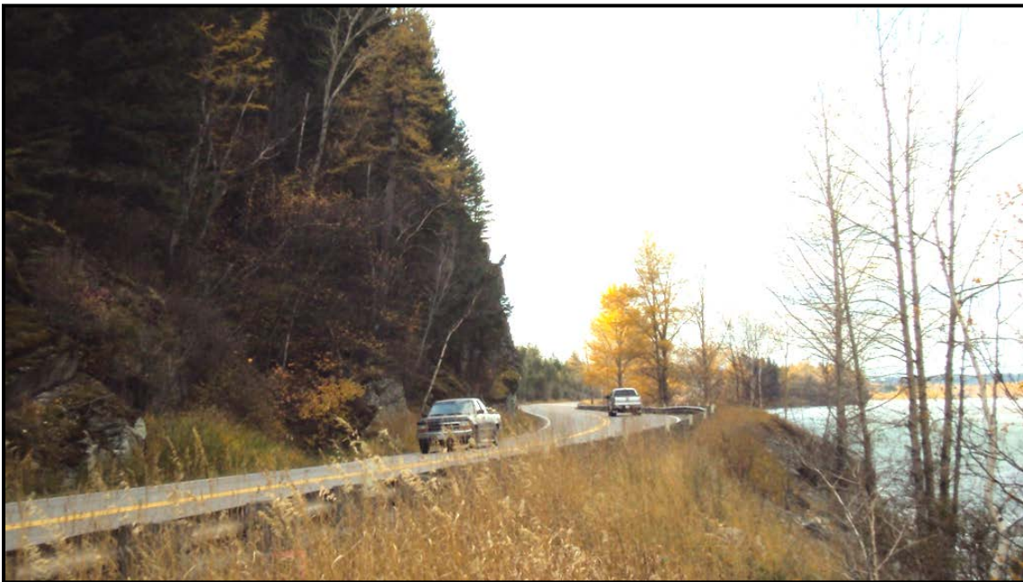
Photo 10. West outcropping along the south side of US 2, steep slope adjacent to river on the north side, and sharp horizontal curve. RP 140.7 (Sta. 50).
