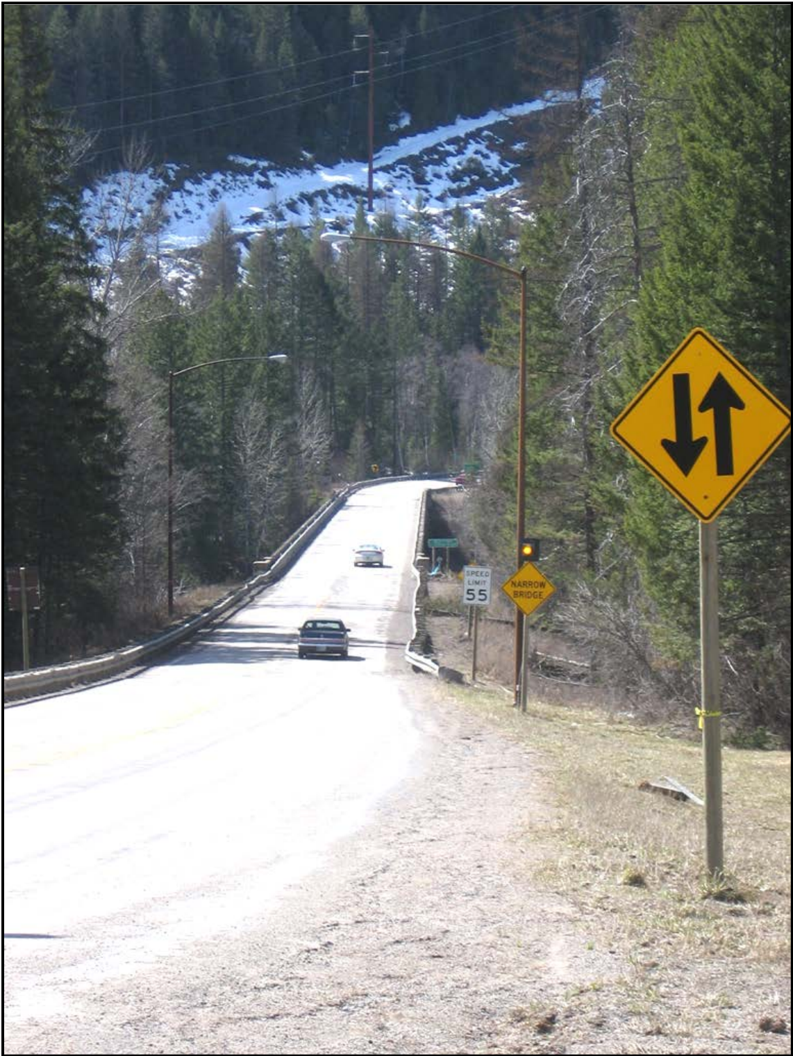
Photo 40. Looking west at the narrow bridge deck over the South Fork of the Flathead River. RP 142.0 (Sta. 120).
