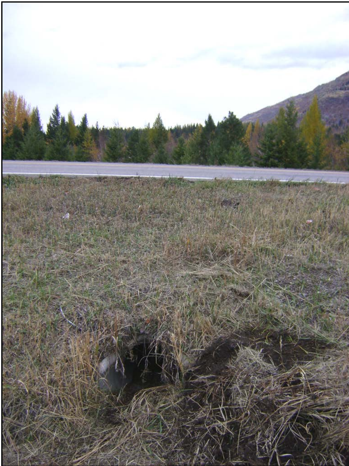
Photo 3. Single 18-inch corrugated metal pipe (CMP) on south side of US 2 at RP 140.1 (Sta. 21).
