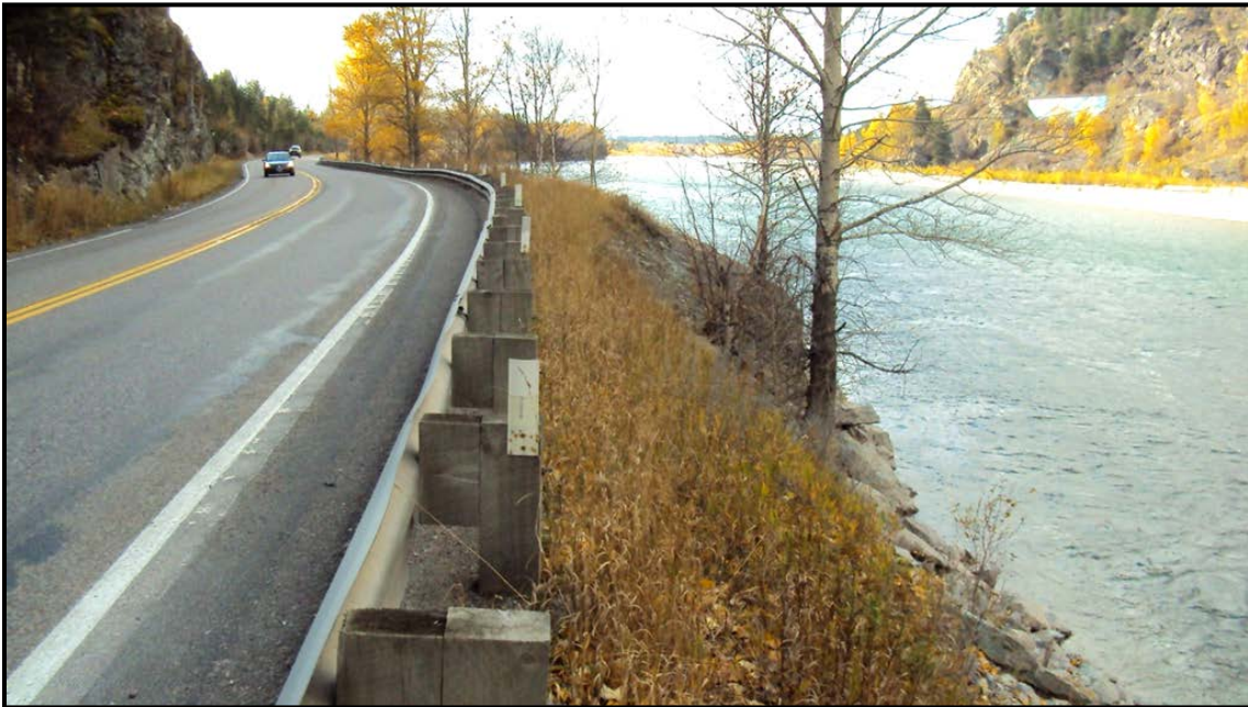
Photo 11. Steep slope adjacent to river on the north side of US 2. RP 140.7 (Sta. 50).
