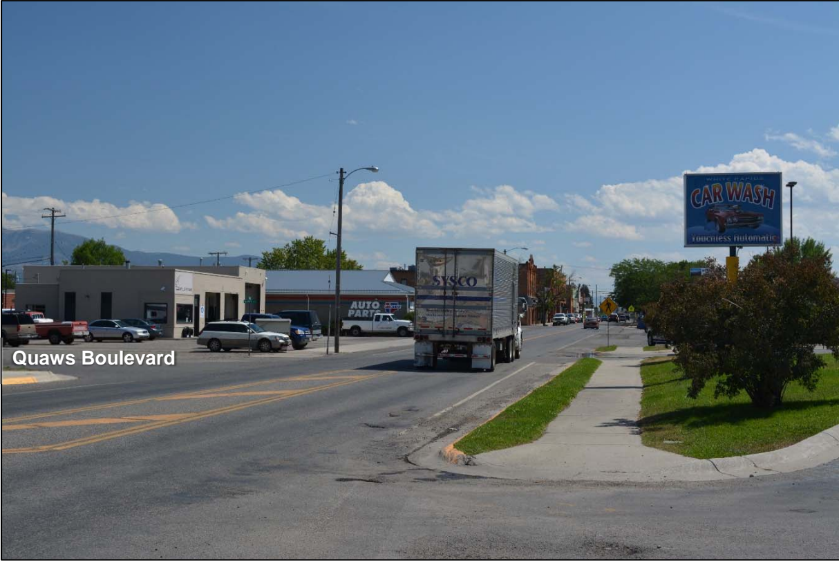
Photo 5: Looking east near Quaws Boulevard (RP 20.0)
