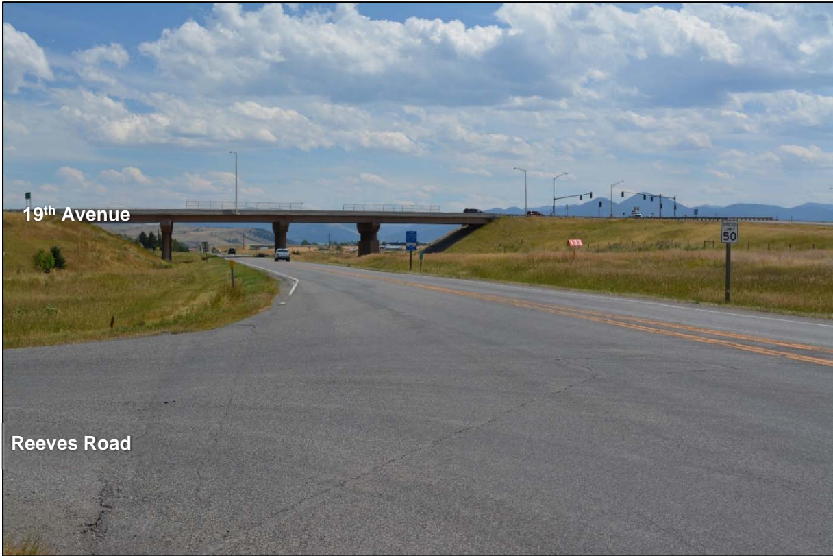
Photo 27: Looking east at Reeves Road (RP 3.1)
