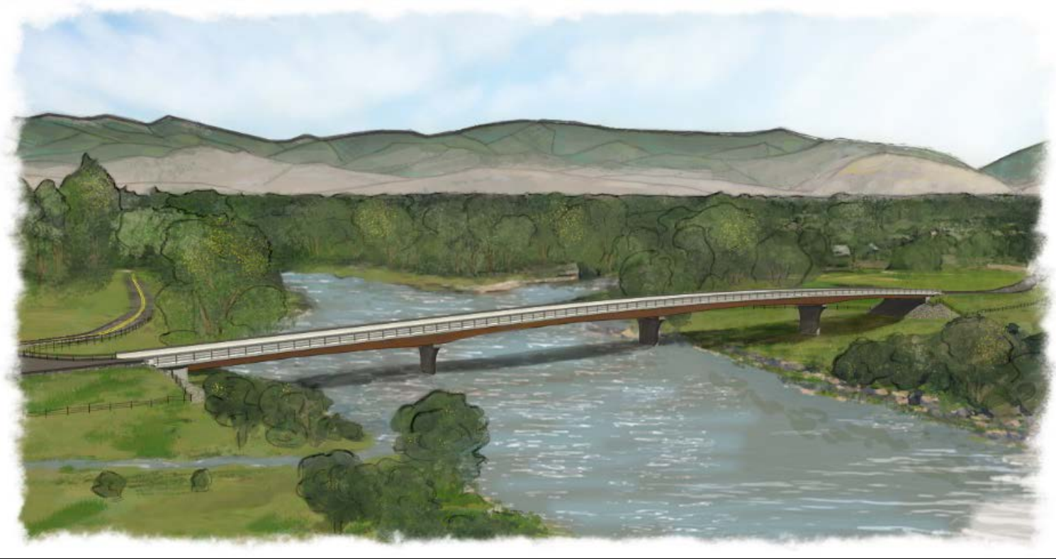
Arched girder profile and wall piers
