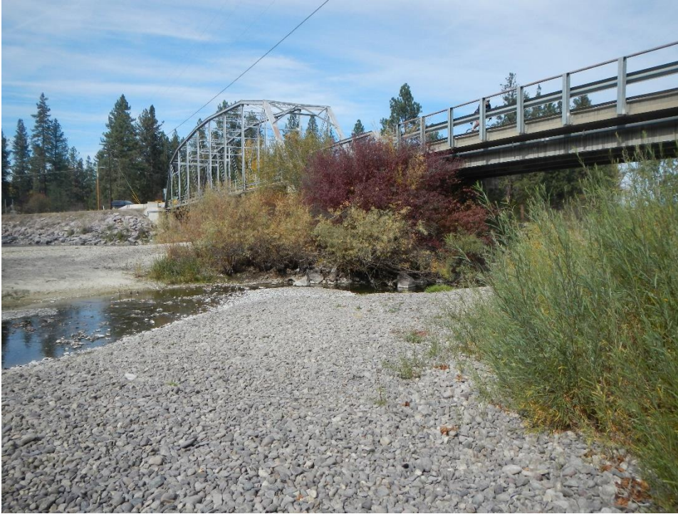
Photo 3: Maclay Bridge and east concrete approach span
