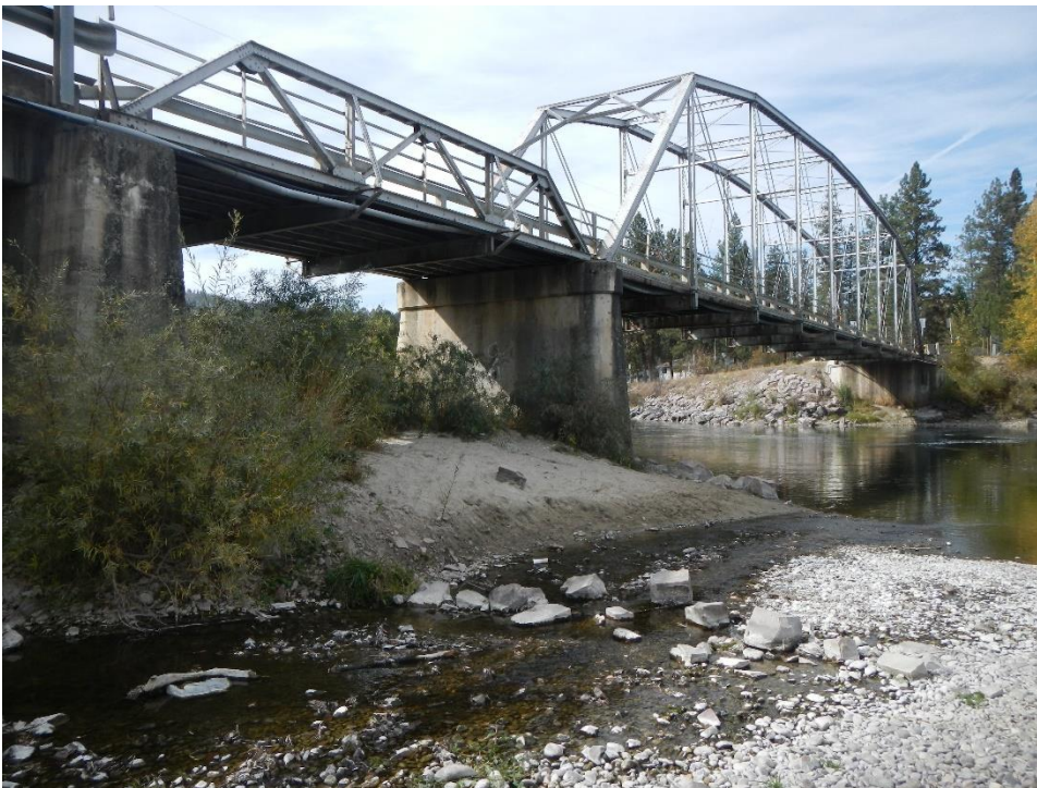
Photo 4: Maclay Bridge and the pony truss segment
