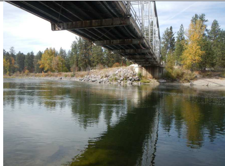
Photo 10. Maclay Bridge, looking across Bitterroot River at left bank.
