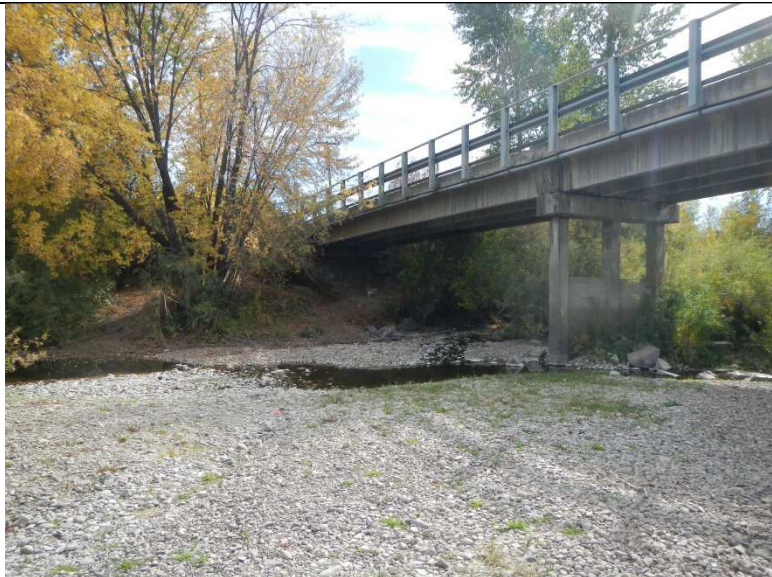
Photo 9. Maclay Bridge, looking at right bank abutments
