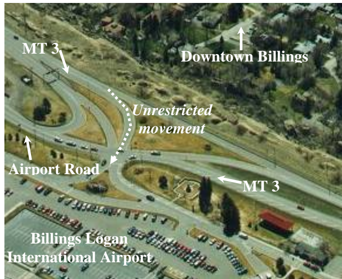
Photo 1-1 Existing Airport Intersection
