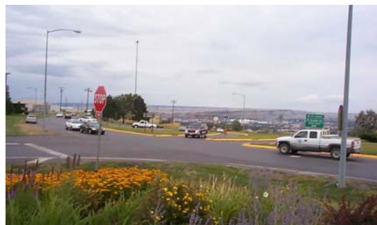
Photo 1-2 View of Airport Intersection (looking southeast)
