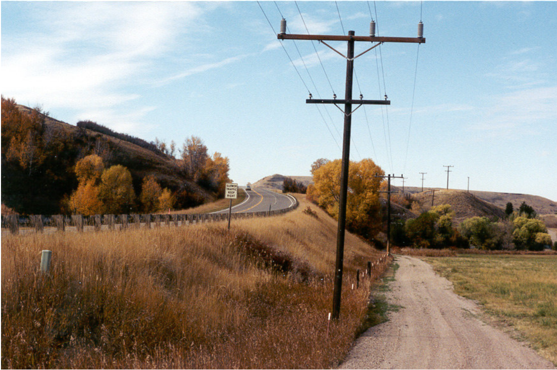
US 89 on approach to Belt Hill (RP 72.6) – looking west
