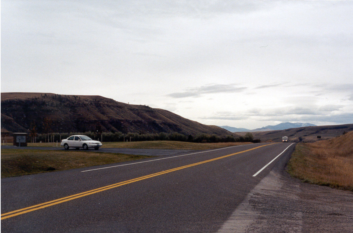
US 89 at entrance to church building (RP 71.9) – looking east
