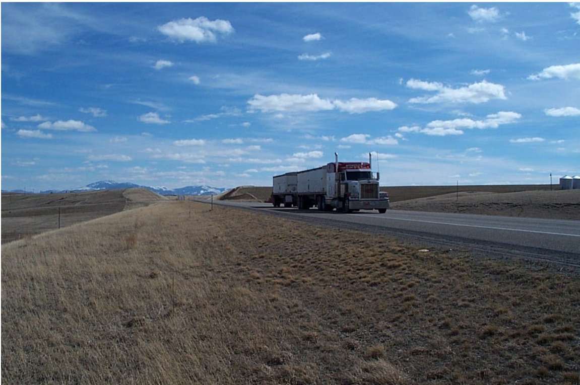
US 89 along northwest extension (RP 83.5) – looking east
