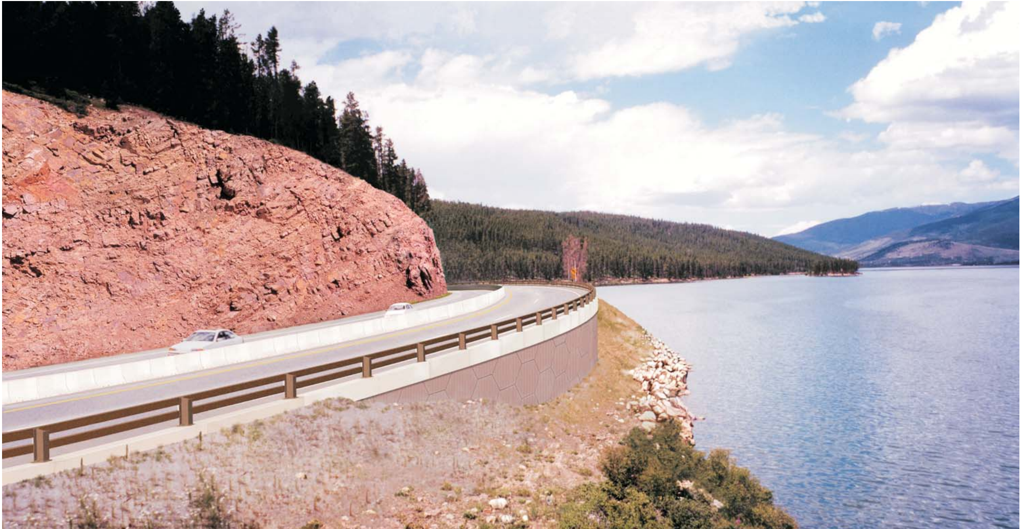
Project: State Highway 9, Summit County, Colorado
