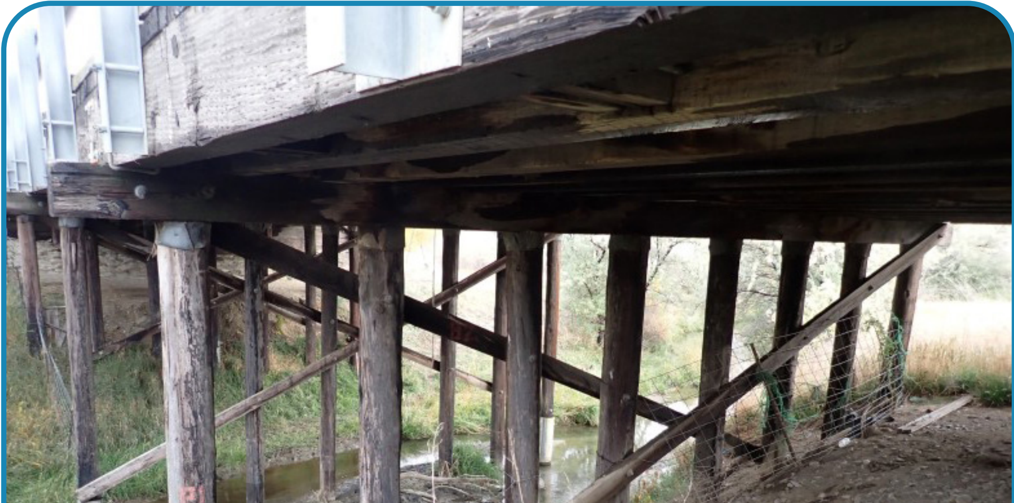
Many of the piles supporting the bridge are bent and corroded.
