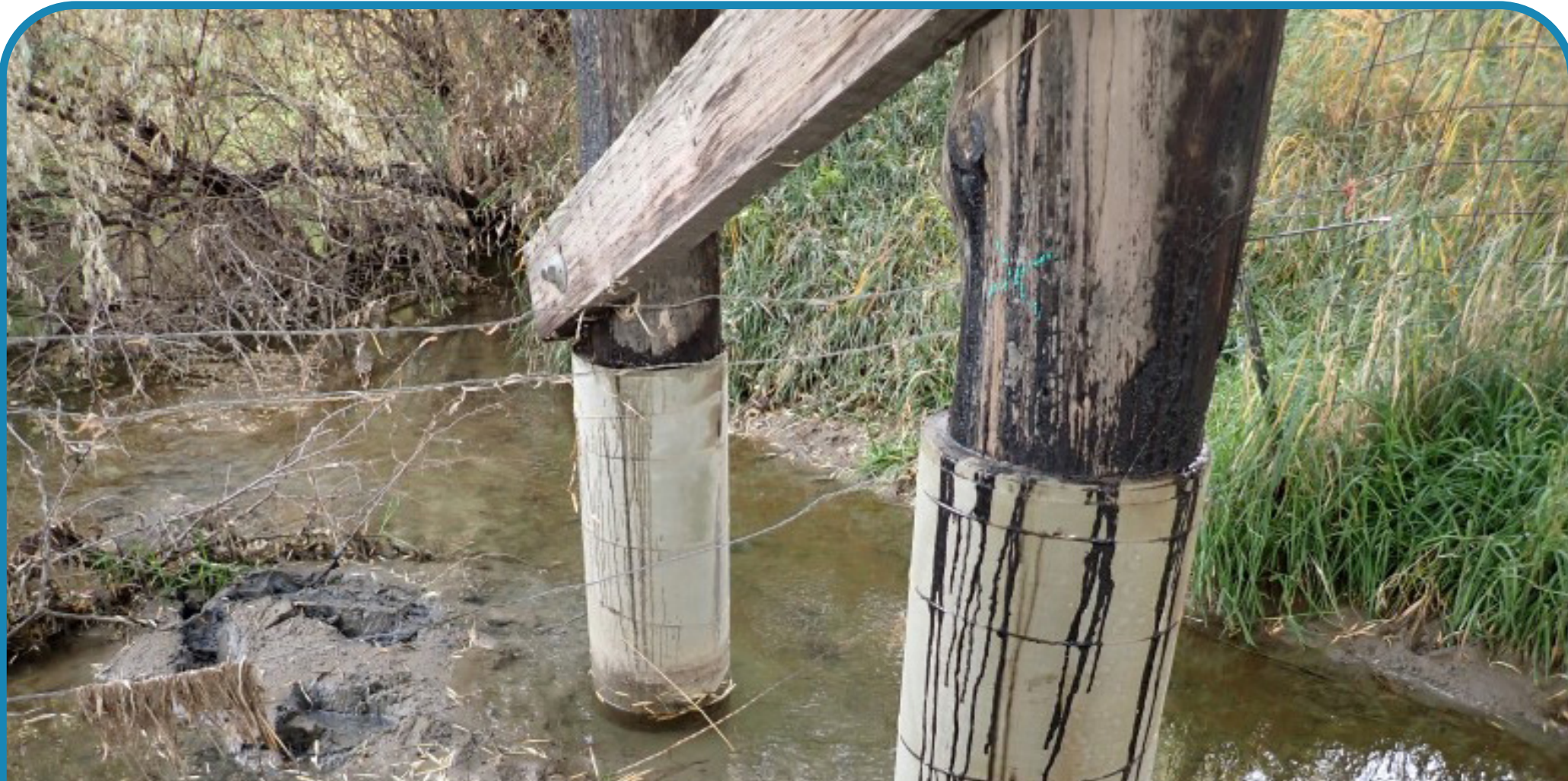
A close-up of bent bridge piles.
