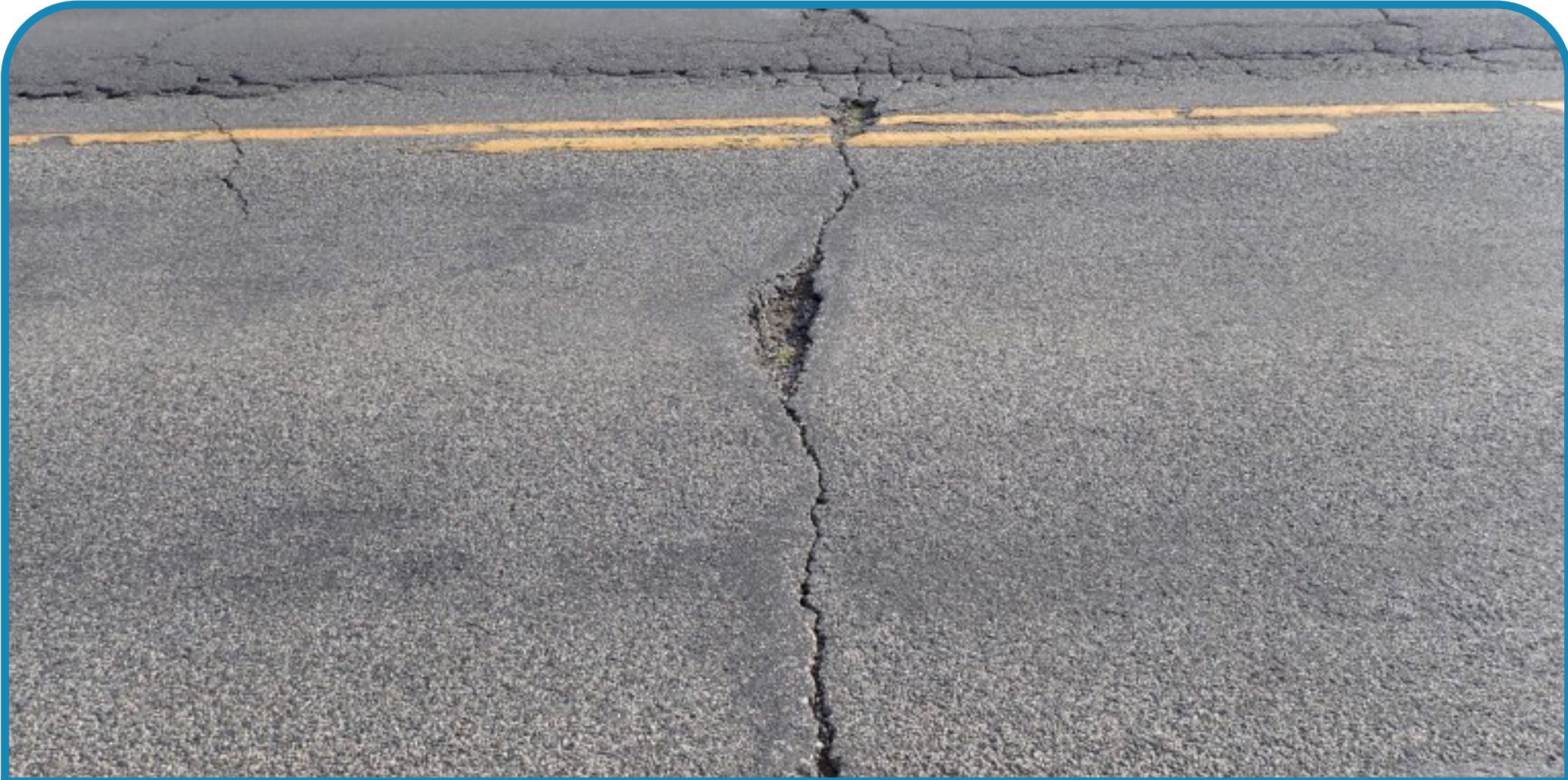
The bridge deck surface is cracked and deteriorating.
