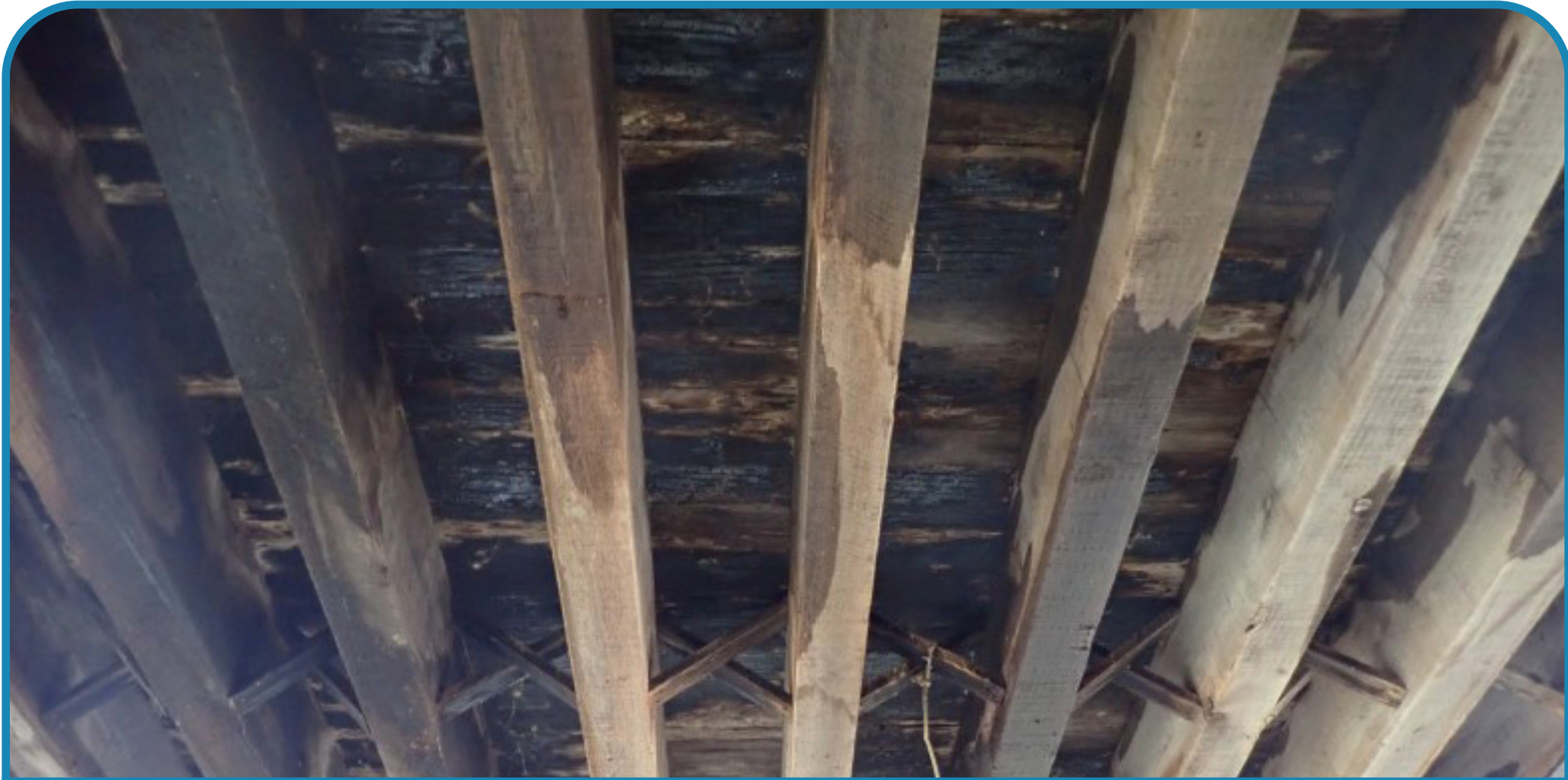
Many of the girders supporting the bridge substructure are cracked and decaying.
