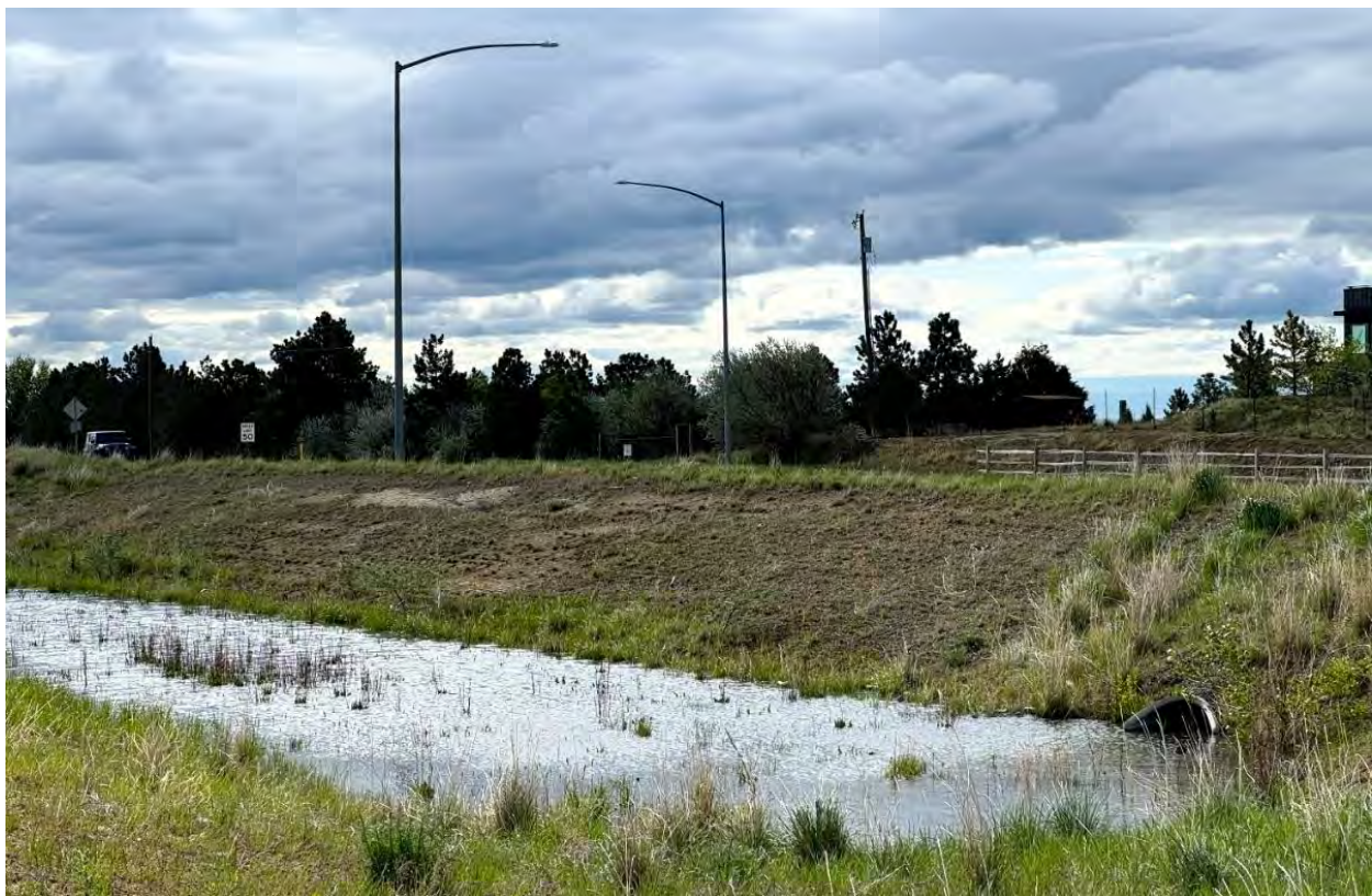
Stormwater detention pond northeast of the Zimmerman Trail roundabout
