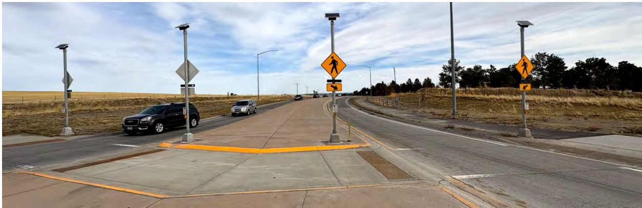
Existing RRFB on the eastern leg of the Zimmerman Trail roundabout
