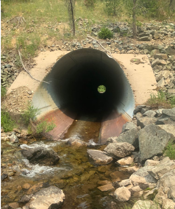
Photo 7: St. Regis River culvert outlet at approximately RP 1.75.
