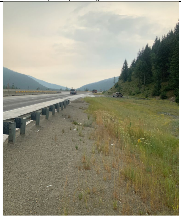
Photo 4: Pullout near RP 1.7, looking west.
