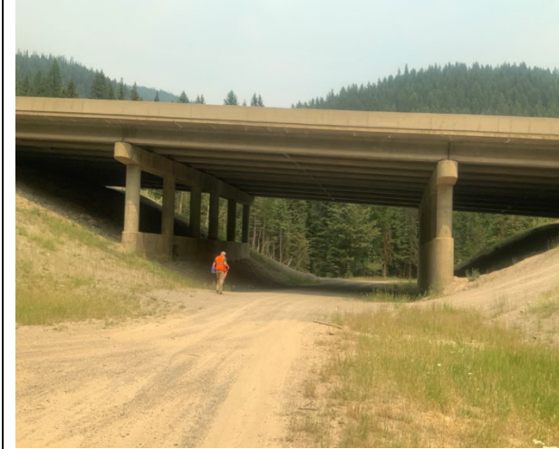
Photo 5: I-90 bridge with NORPAC road underneath, at RP 1.9.
