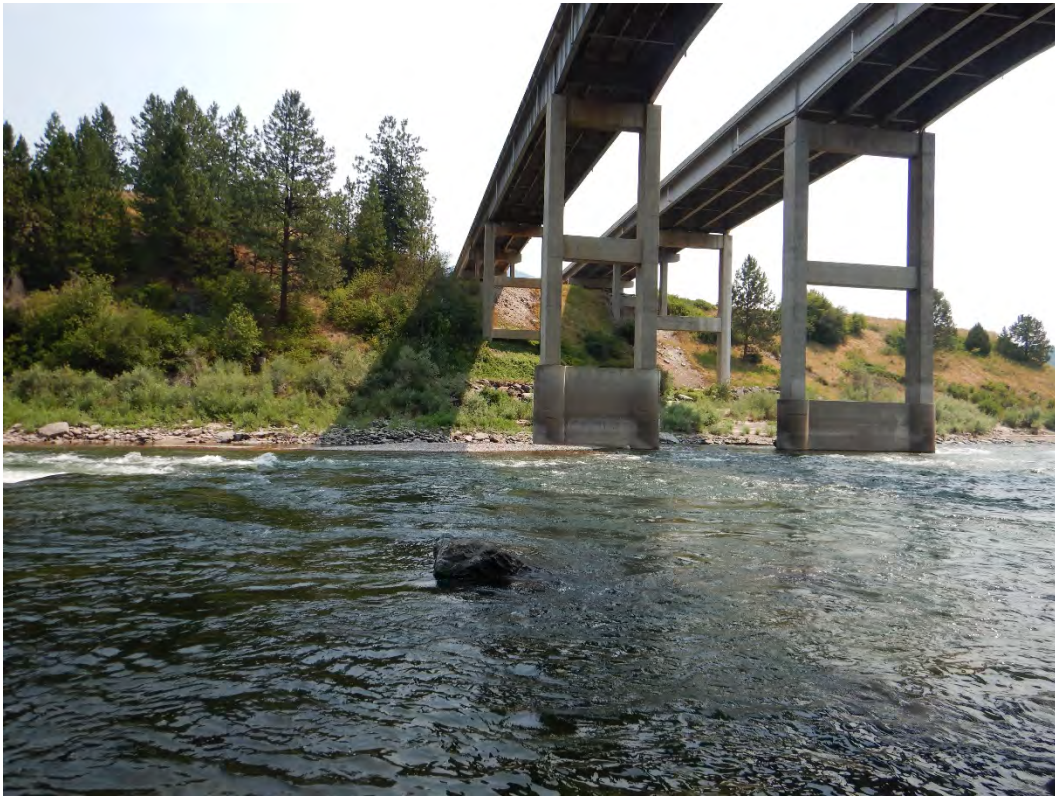
Figure 6: Underside of Cyr Bridge facing east.
