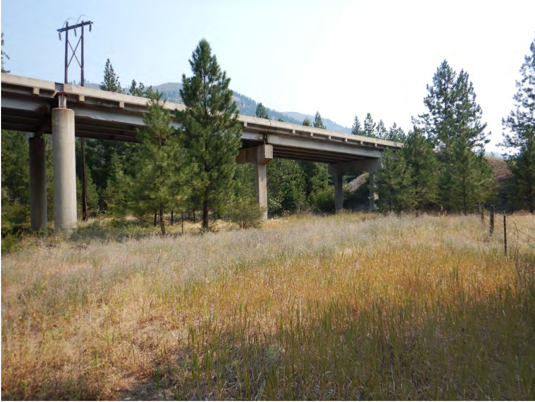
Figure 1: Existing wildlife accommodation below Old Highway 10 Bridge.
